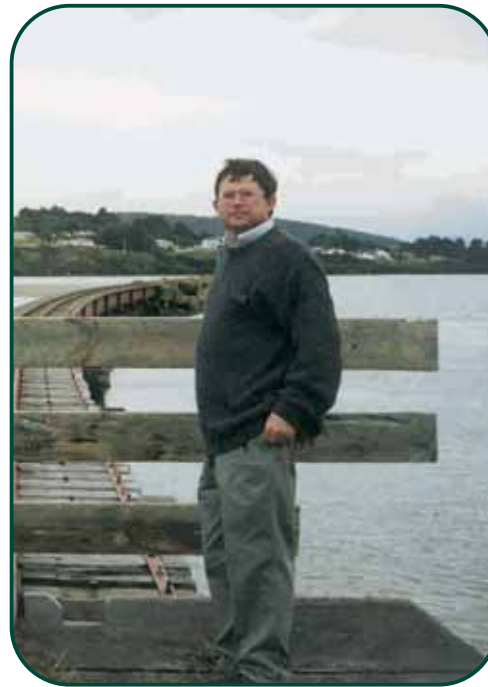
Manager Crown Property Contracts Paul Jackson gets a first-hand look at the enormity of the task ahead demolishing and removing the Riverton Rail Bridge.
