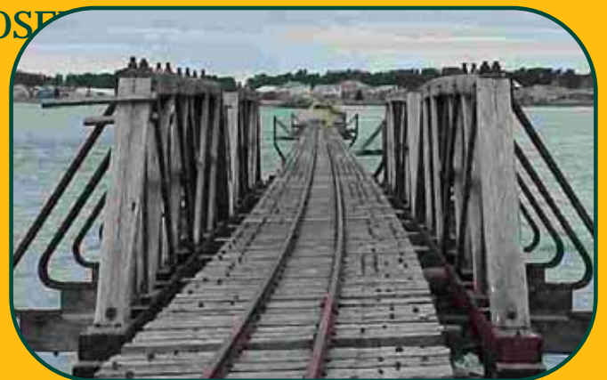
Demolition of the Riverton Bridge will pose some logistical challenges.
