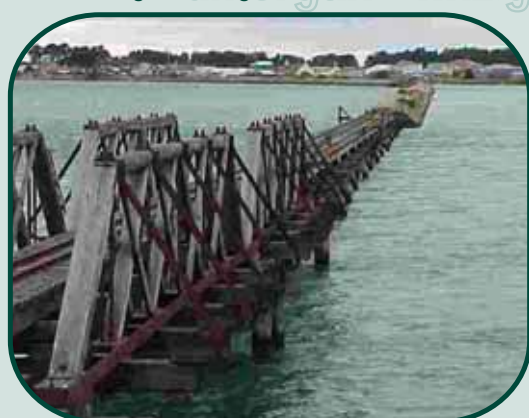
A Howe truss, one of the wooden supporting structures, will be preserved for display.
