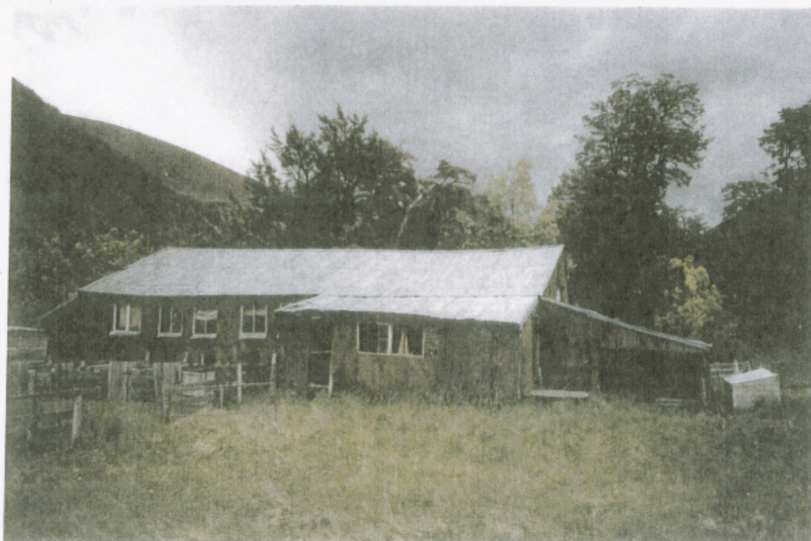
Fig. 4 The historic 7-stand woolshed is still in working order, and provides additional interest for recreational visitors. It includes a wool room, covered yards, a drafting race and nearby, an old fashioned pot dip.
