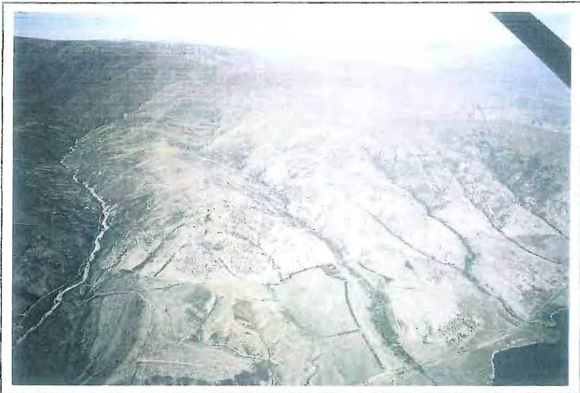
Fig. 5. State Highway 83 can be seen alongside Lake Aviemore in this view, while the dome of St Mary's Range and the St Mary's Conservation Area can be seen on the skyline (top left). Access to St Mary's Range has not been easy in the past but the proposed public access up the spur on the true left of McRaes Creek (centre) will greatly improve this situation and is strongly supported by FMC.
