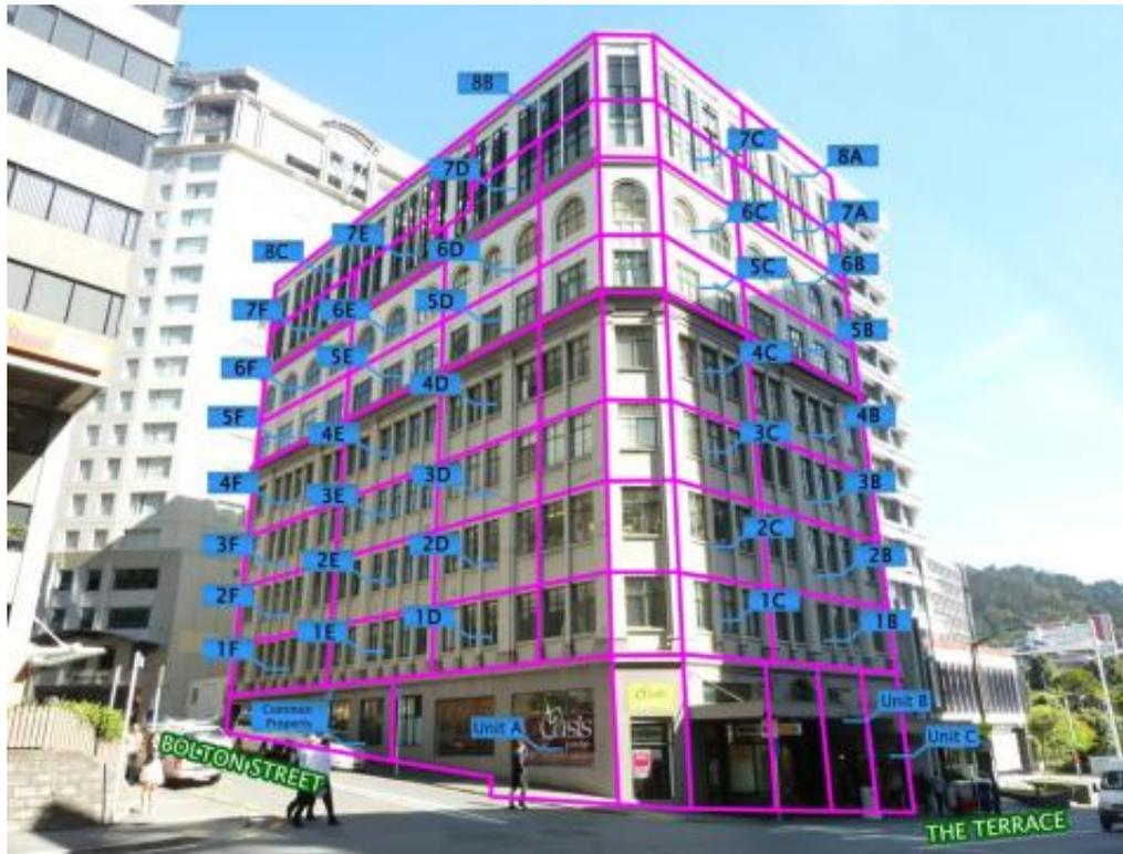
Mock up showing building with 3D unit boundaries overlaid. Gulliver T. F. D. (2015). Developing a Three-dimensional Digital Cadastral System for New Zealand (working title). Thesis in preparation. University of Canterbury.
