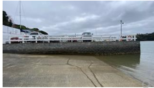
Eastern Side of Reclamation
