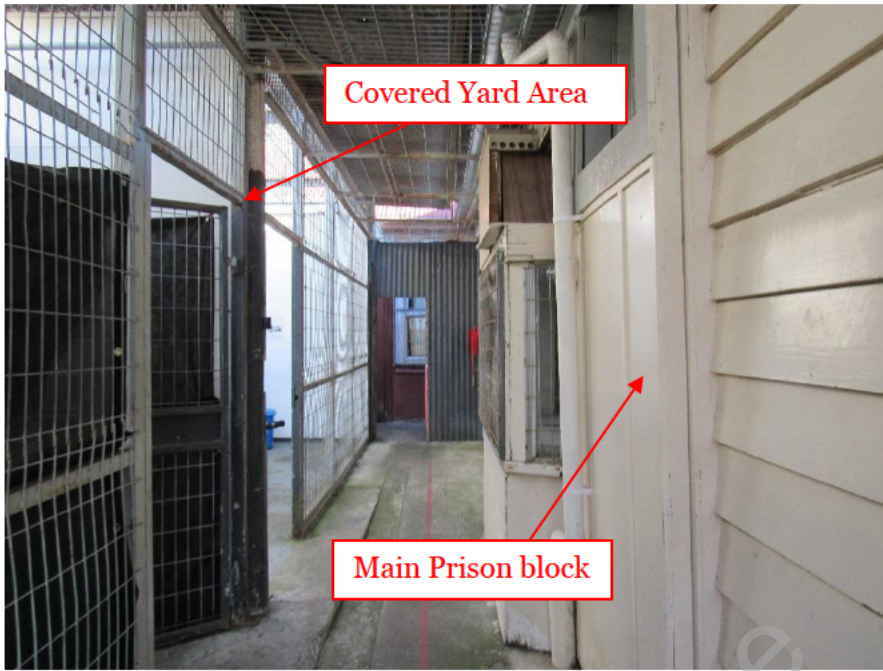
Figure 20: Corridor between the main prison block and the covered yard area
