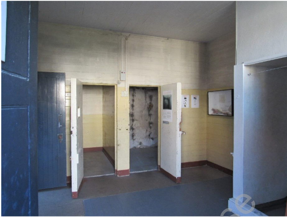
Figure 8: Timber sarking for internal walls.
