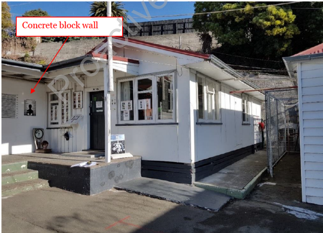
Figure 9: External view of the main office block.
