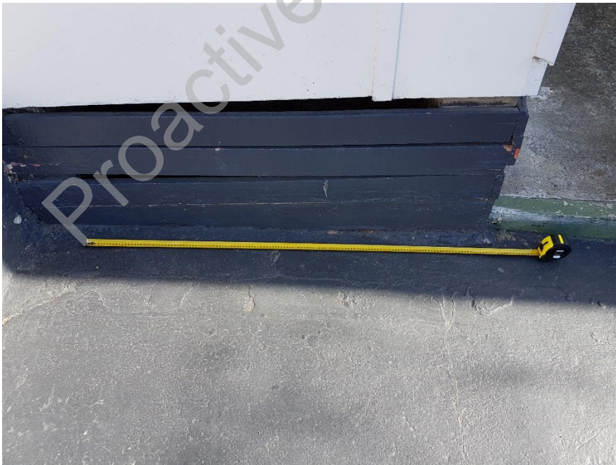
Figure 3: Timber board walls around the perimeter of the building.
