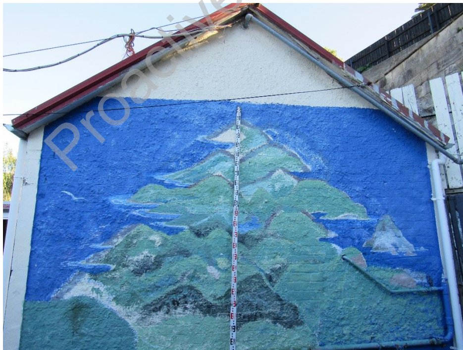
Figure 17: External wall lining for the wash/shower block.
