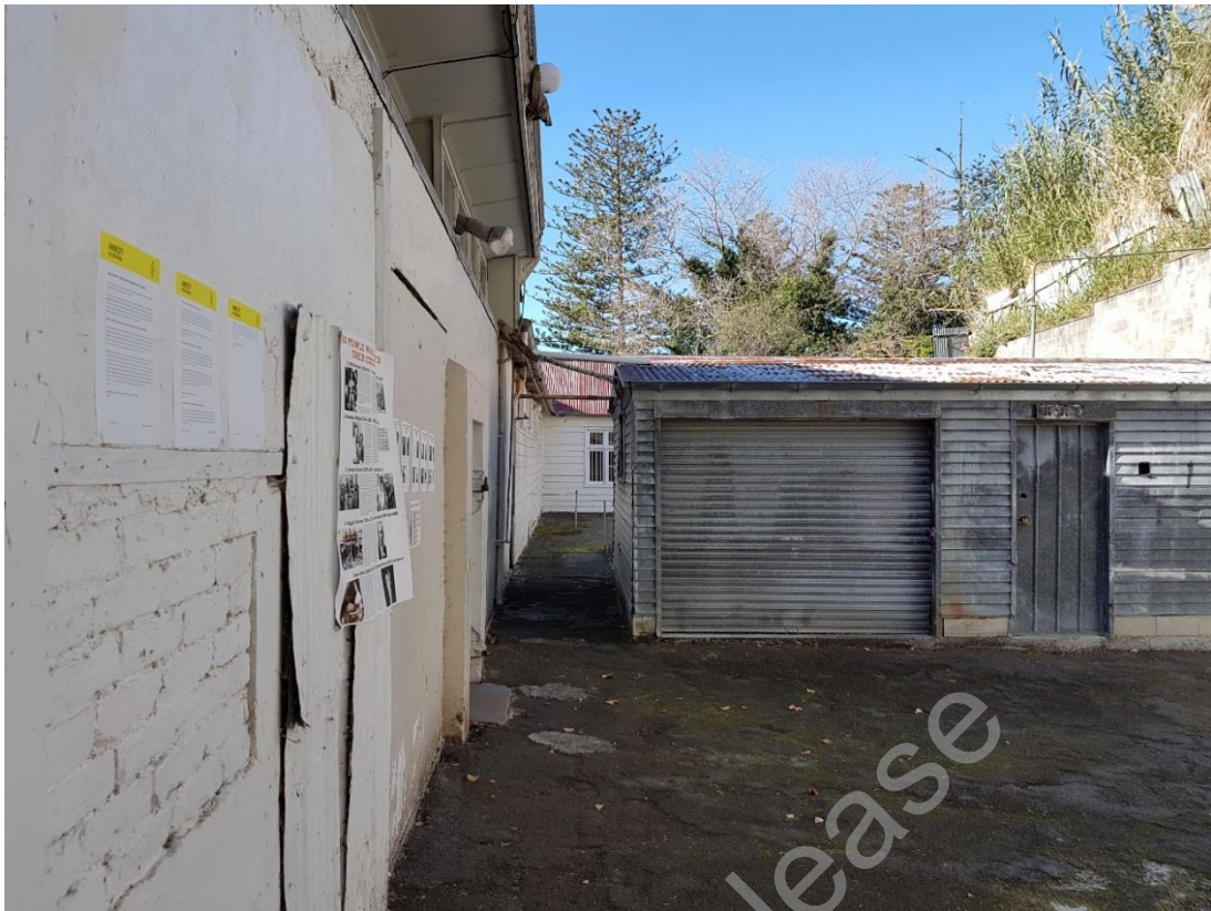
Figure 15: External view of the wall of the Dining Hall.
