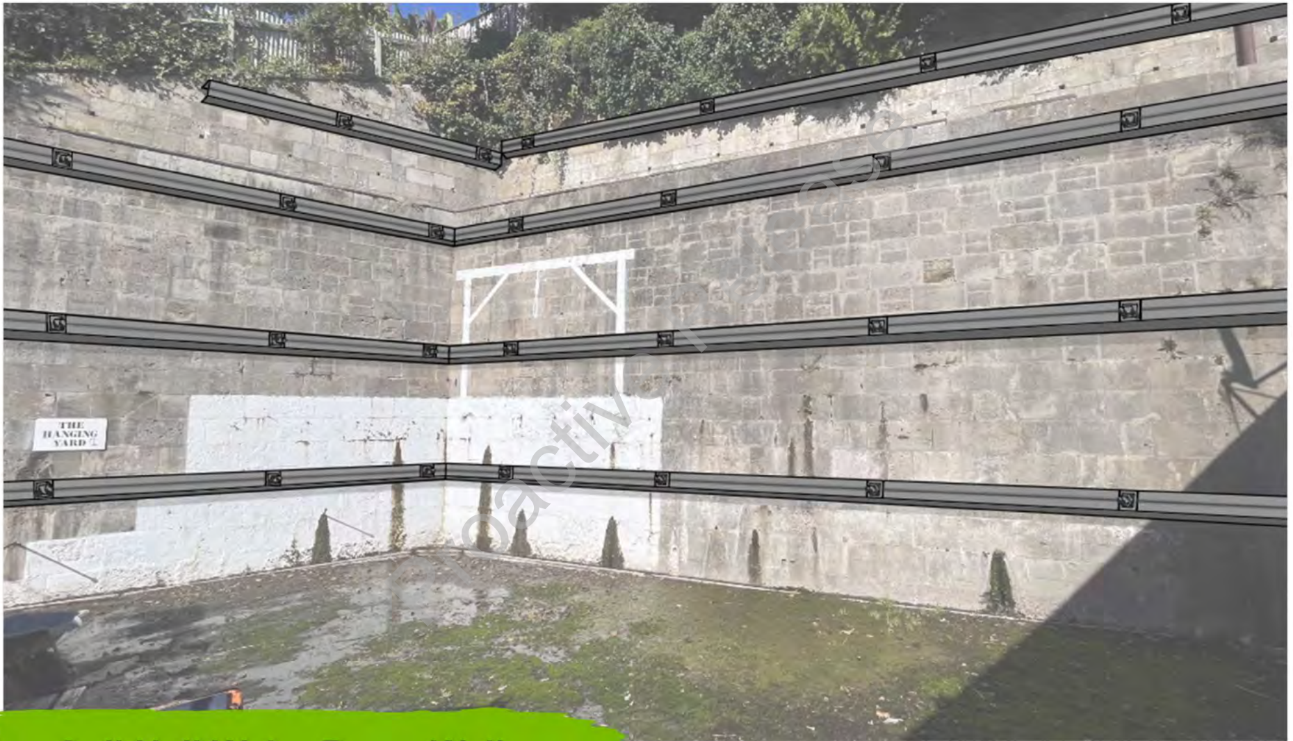
Soil Nail Waler Beam Wall
