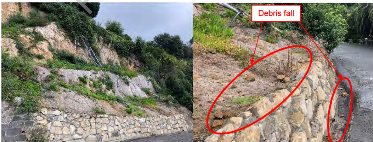
Figure 8: Retaining Wall RW6, the existing slip and loose debris during the site inspection between 14 and 17 March 2022.
