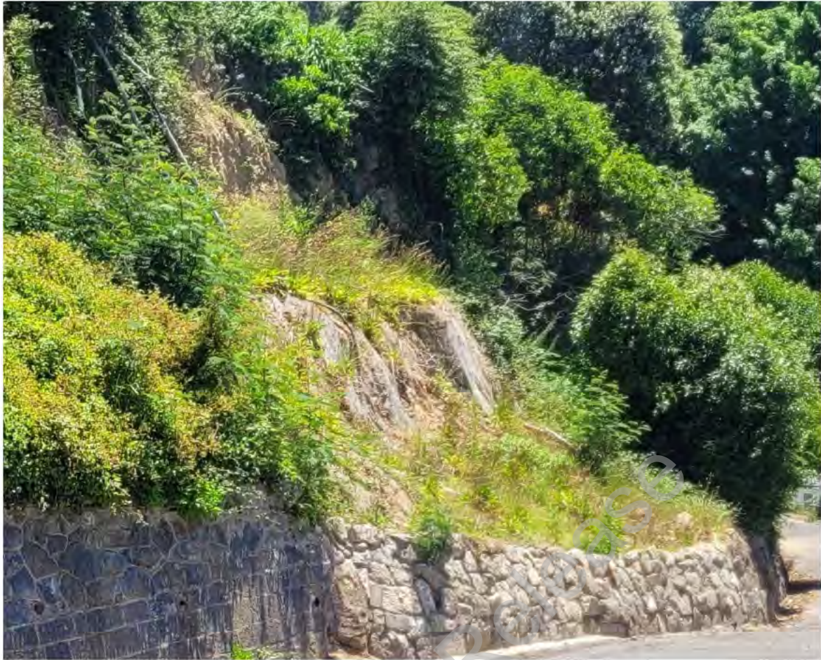
Figure 9: Retaining Wall RW6 and the existing slip with increased vegetation cover on 22 November 2022.
