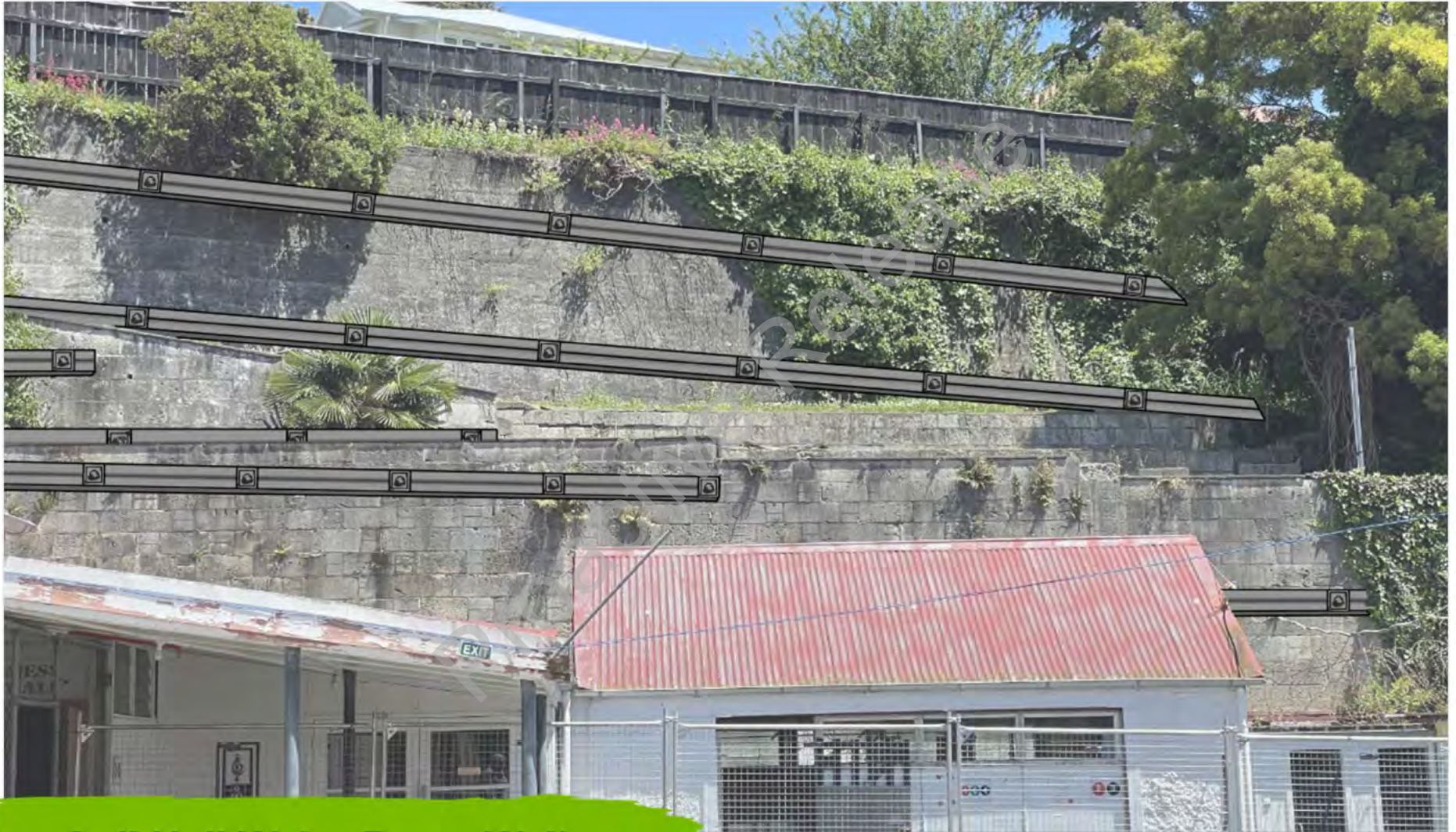
Soil Nail Waler Beam Wall
