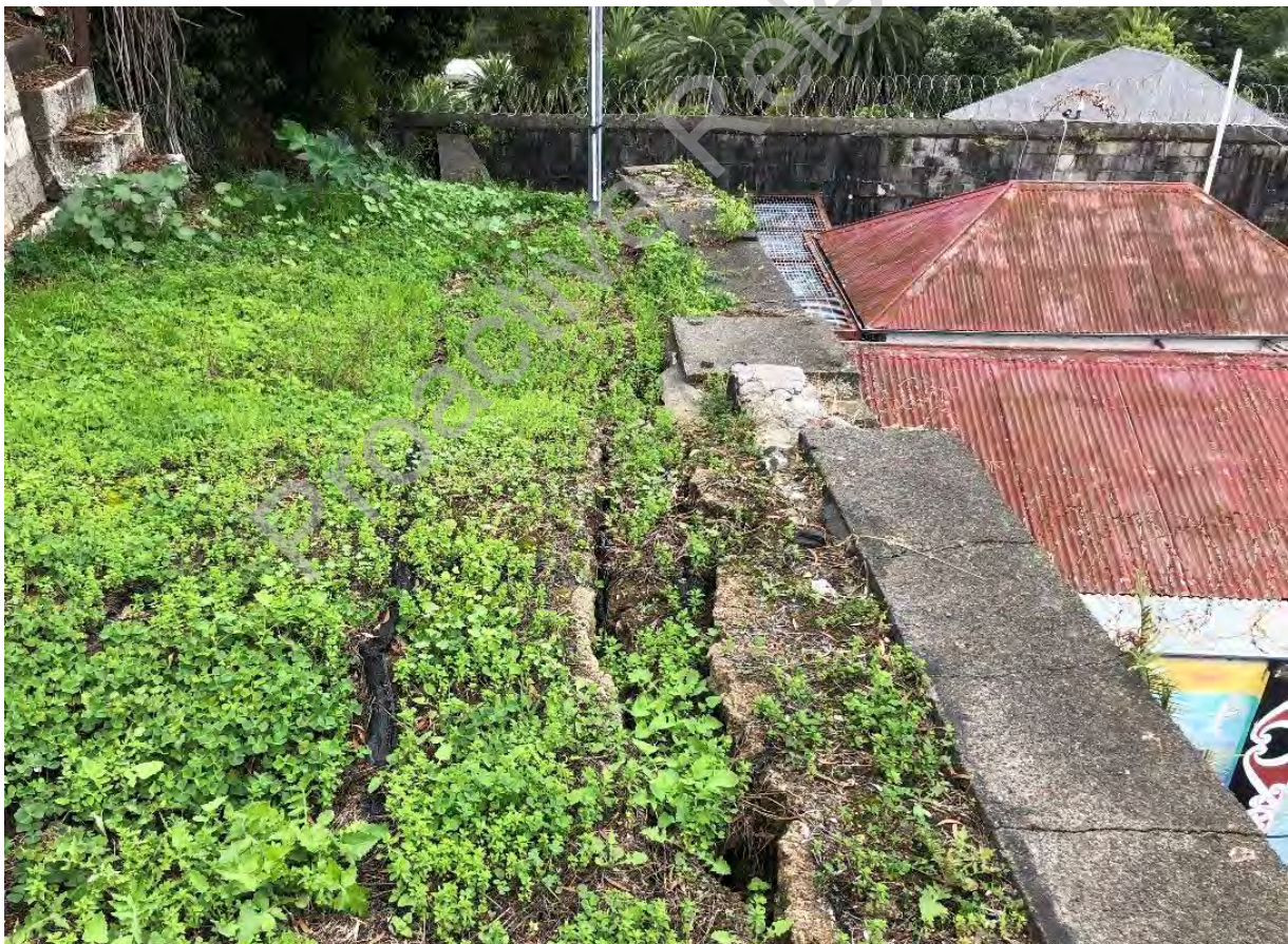
Figure 4: Tension cracks in the inferred silt backfill behind Retaining Wall RW10 during the site inspection between 14 and 17 March 2022.
