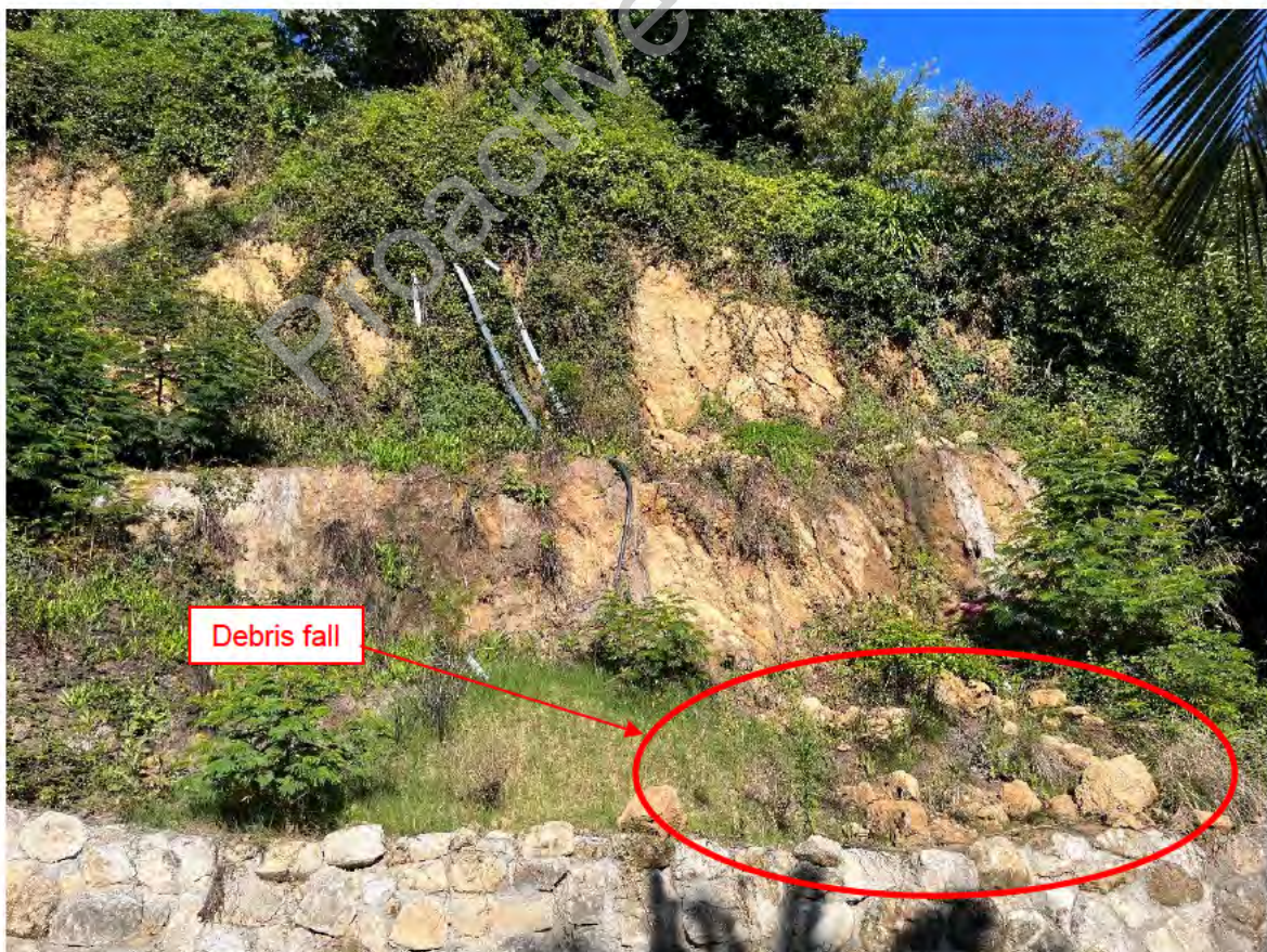
Figure 10: Retaining Wall RW6, the existing slip and larger pieces of debris on 3 March 2023.
