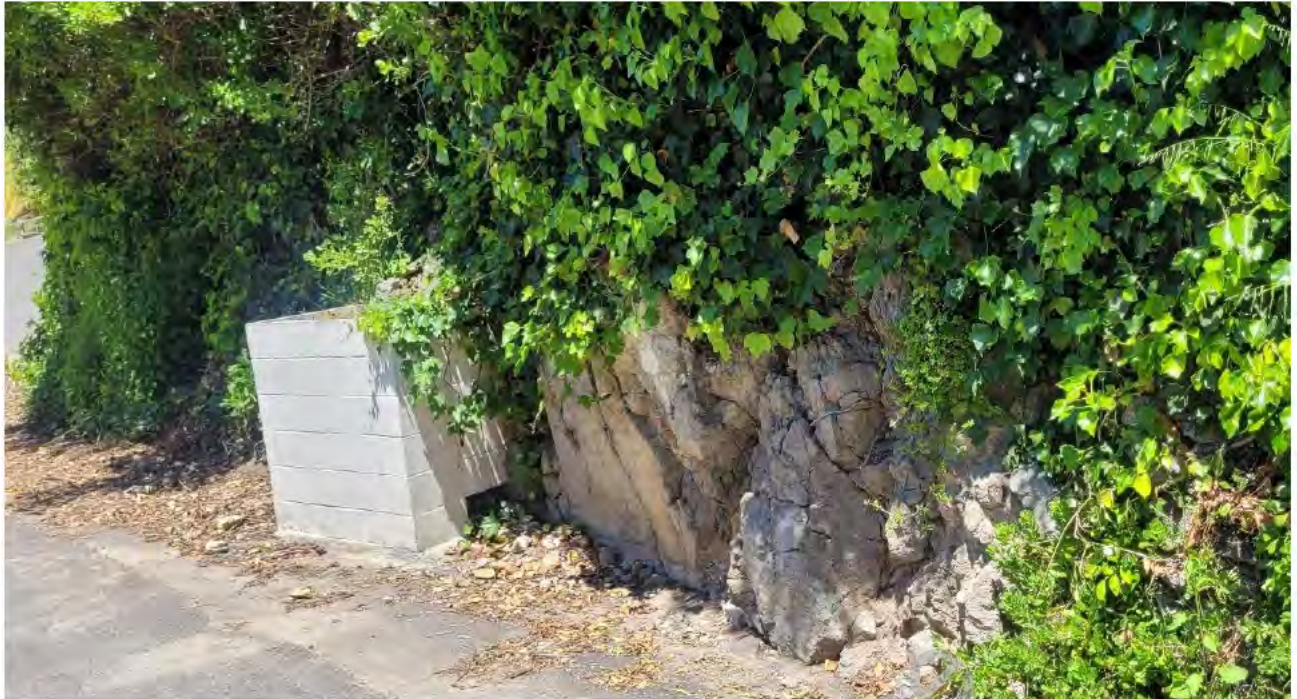
Figure 7: Exposed cut limestone rock face along site access driveway on 22 November 2022.
