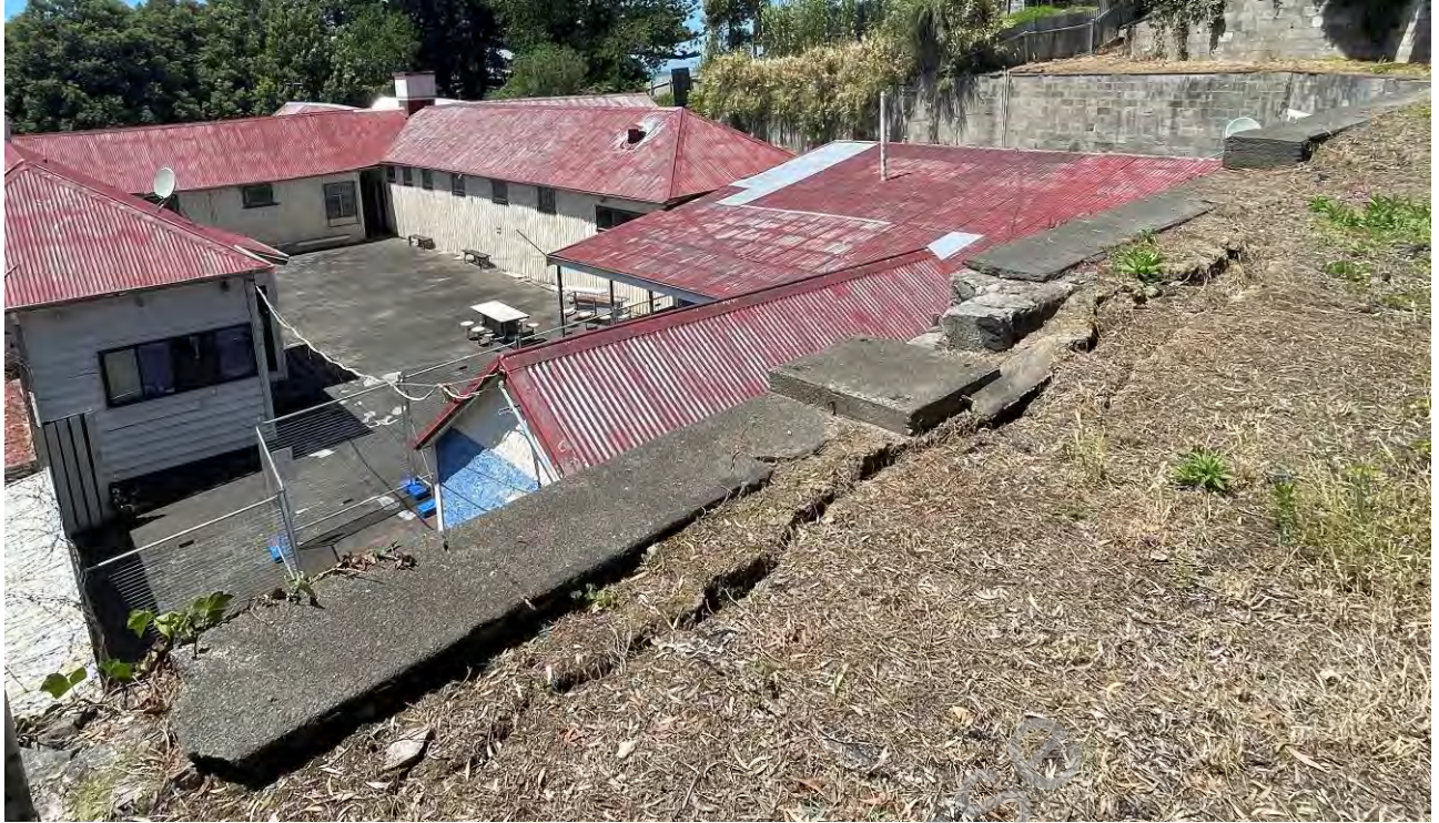
Figure 5: Tension cracks in the inferred silt backfill behind Retaining Wall RW10 during the site inspection on 24 November 2022.
