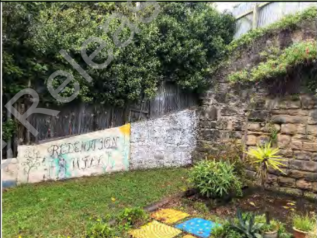
Photo 4) Mass concrete wall observed adjacent to NAP-PRIS-RW17.
