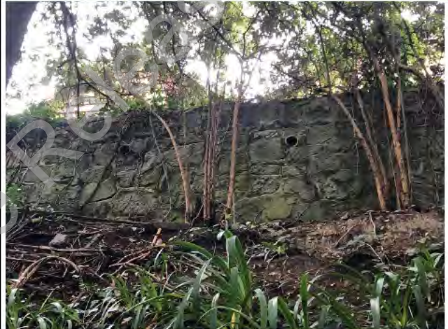
Photo 4) Typical wall face condition.
