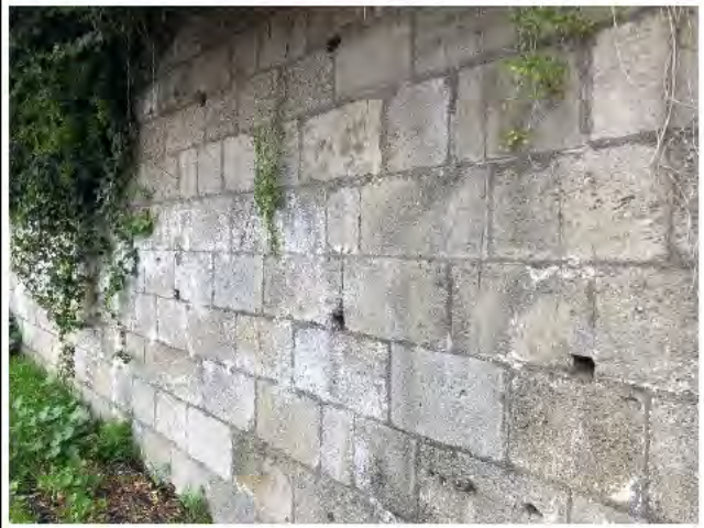
Photo 2) Typical wall face observed. Note "square" holes are weep holes/wall drainage.
