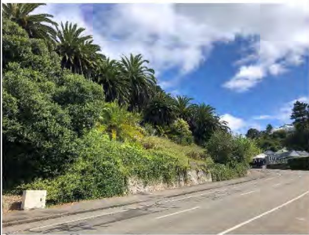
Photo 1) NAP-PRIS-RW21 view. Note Coote Road in foreground.
