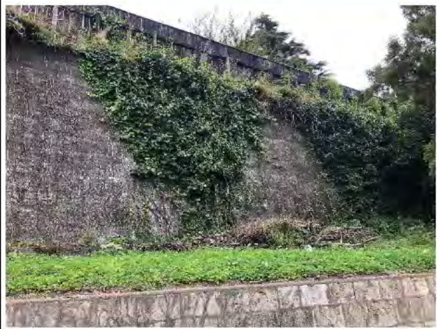
Photo 2) NAP-PRIS-12 view. Located along upslope property boundary.
