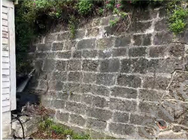
Photo 3) Typical view of wall face.
