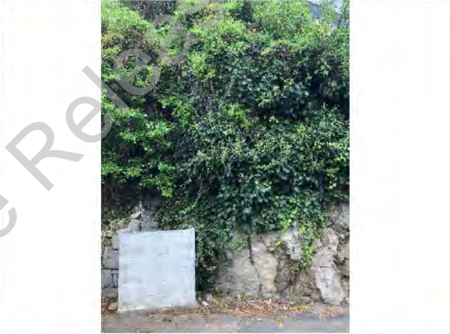
Photo 4) Historical concrete stormwater channel (inferred) observed in front of wall.
