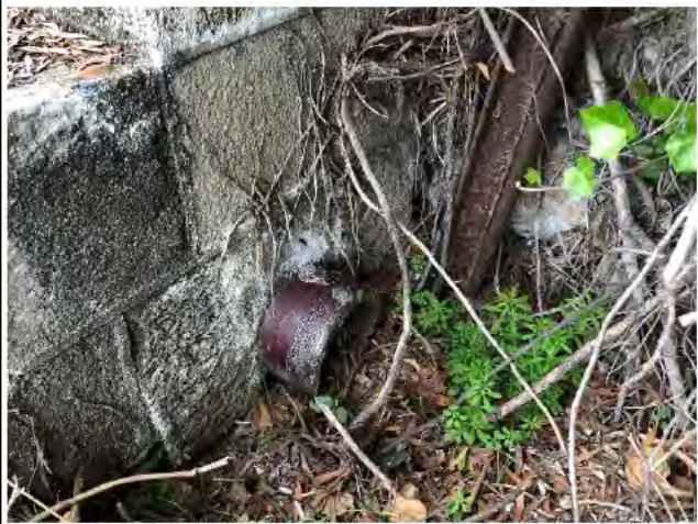
Photo 2) Drainage outlet at wall toe.
