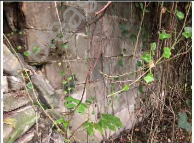
Photo 4) Concrete block section of NAP-PRIS-09.
