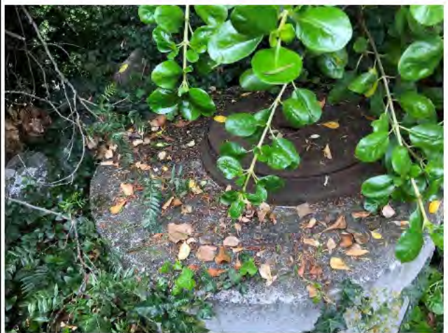
Photo 6) Manhole observed immediately behind top of wall.
