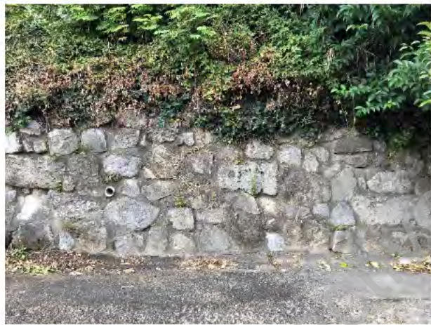
Photo 3) Retaining wall face and weep hole/drain
