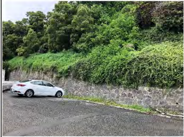
Photo 2) NAP-PRIS-07 view. Note heavy vegetation at top of wall.
