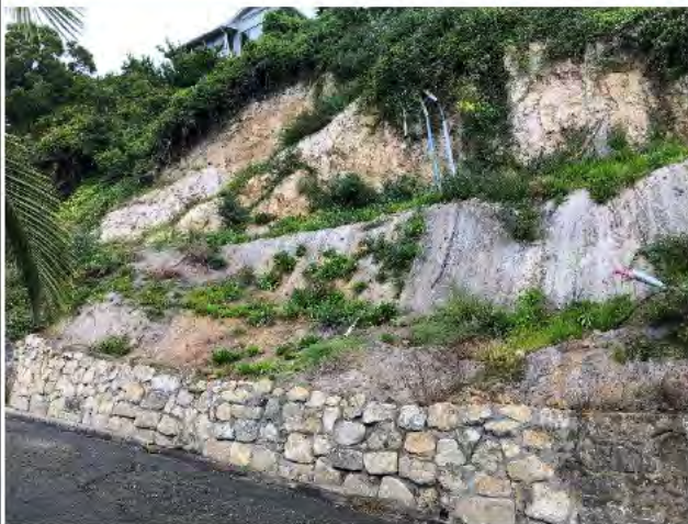
Photo 1) NAP-PRIS-06 view. Note recent slope failure and “new” construction of wall, also upslope residential property.
