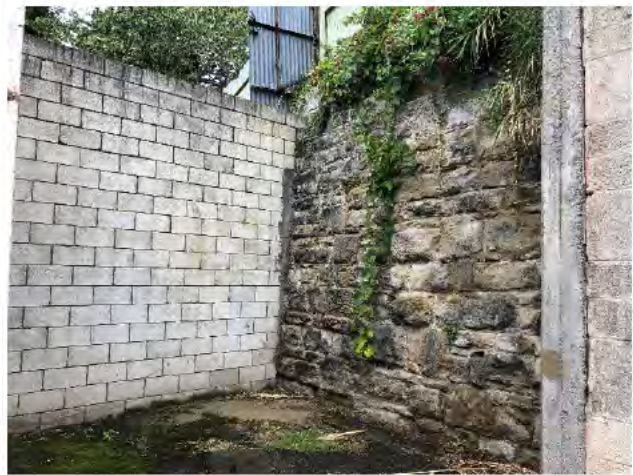
Photo 2) NAP-PRIS-RW17 view. Note concrete block wall appears to be recently constructed.
