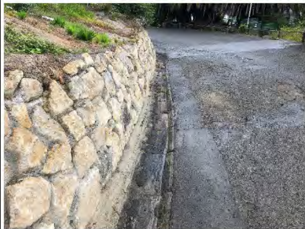
Photo 6) Wall face and drainage channel at toe of wall.
