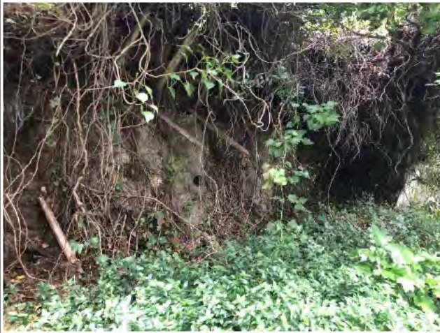
Photo 1) NAP-PRIS-RW14 view. Located below neighbouring residential property.
