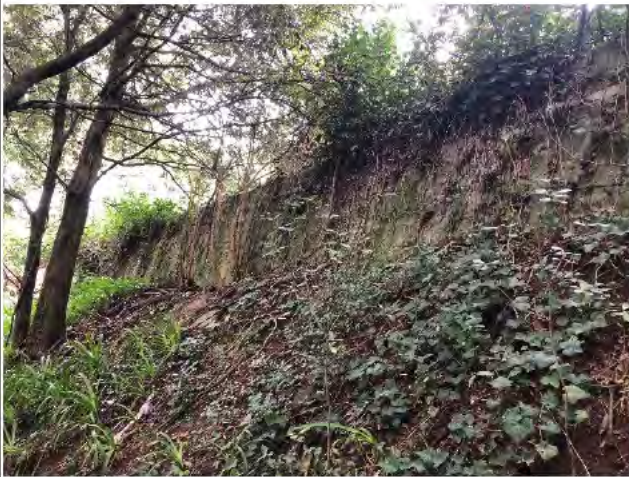
Photo 1) NAP-PRIS-RW19 view. Note steep toe slope.
