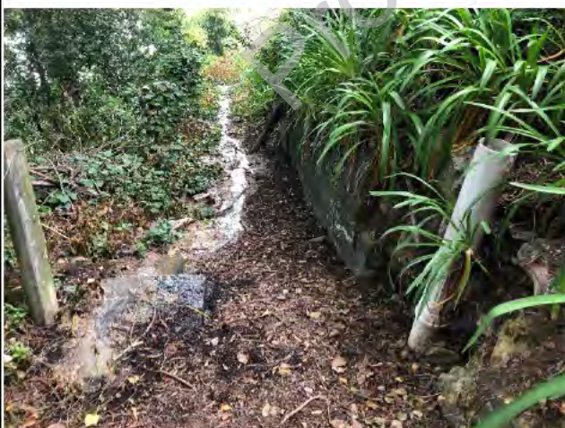
Photo 5) Raw sewage leaking from sump in front of wall.
