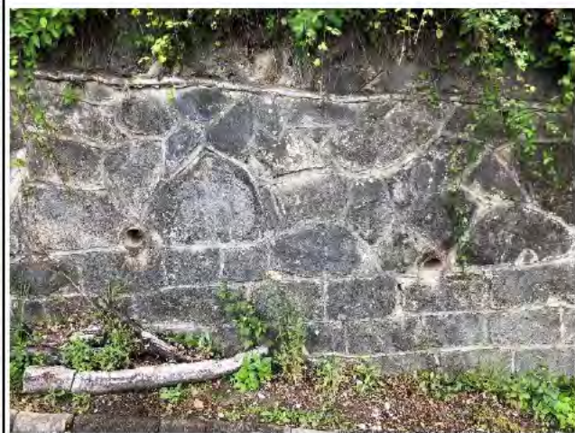
Photo 6) Wall face and drainage holes.
