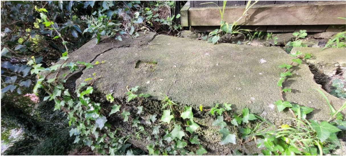
Photo 1 – Cracking at the end of RW12.
