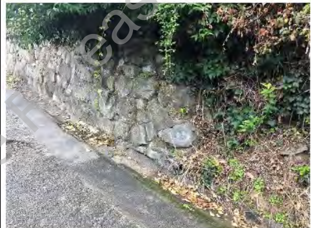
Photo 4) End of wall, drain pipe located at toe of wall.
