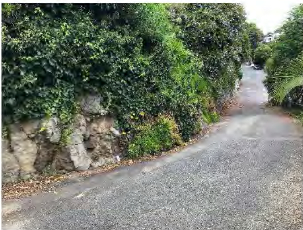
Photo 1) NAP-PRIS-03 view above site access/driveway.
