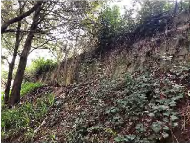
Photo 1) NAP-PRIS-RW19 view. Note steep toe slope.
