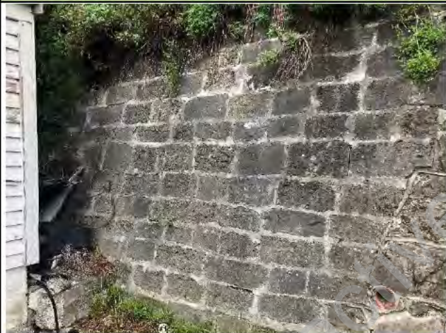
Photo 3) Typical view of wall face.
