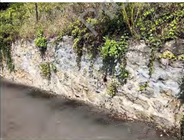
Photo 5) Section appears to have been re-mortared recently.
