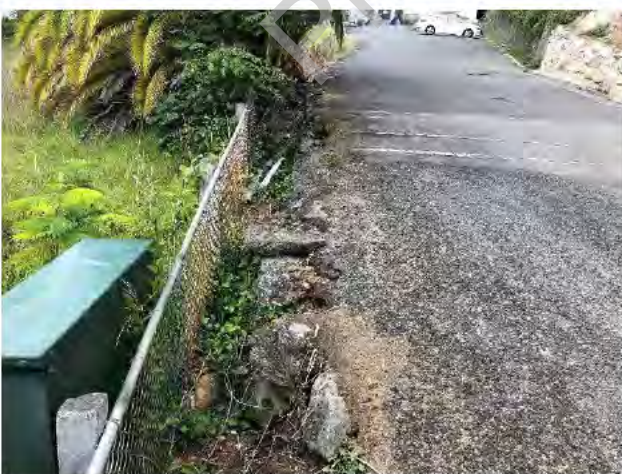
Photo 5) Power box observed in front of wall.
