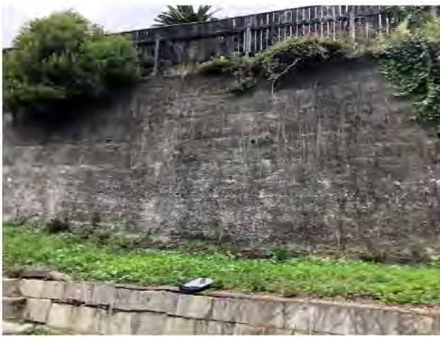
Photo 1) NAP-PRIS-12 view. Located along upslope property boundary.
