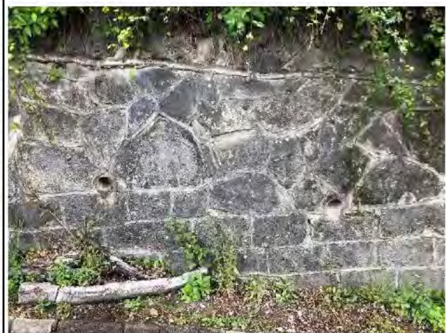
Photo 6) Wall face and drainage holes.
