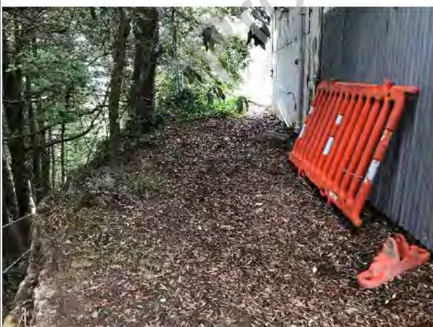
Photo 5) Top of wall. Note edge of prison building shown on right.
