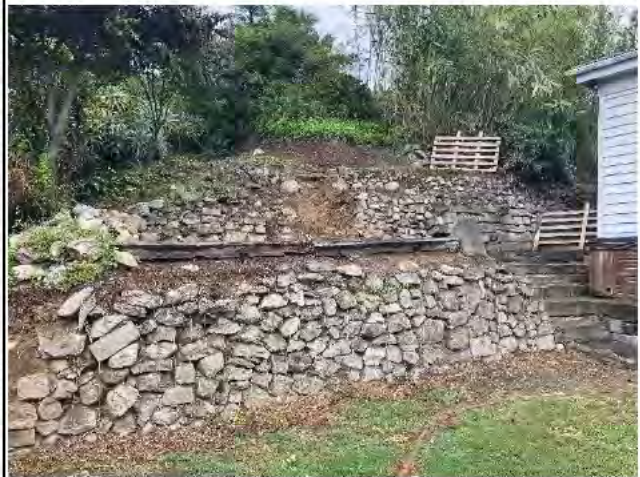
Photo 2) NAP-PRIS-RW18 view, section used for landscaping.
