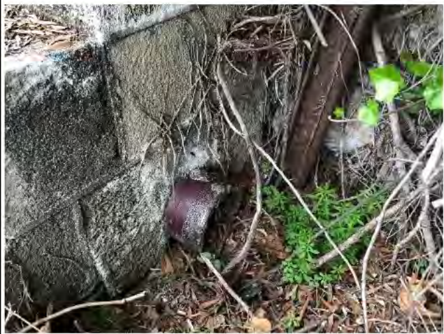
Photo 2) Drainage outlet at wall toe.
