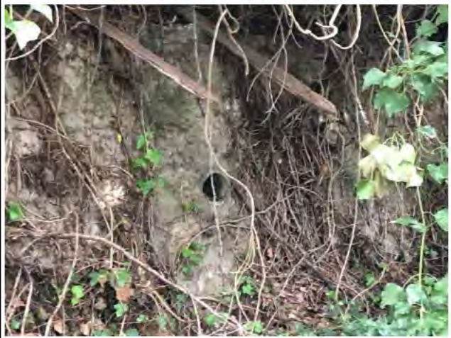
Photo 2) Drainage pipe observed.
