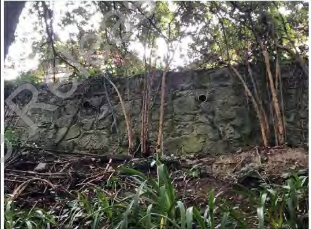
Photo 4) Typical wall face condition.
