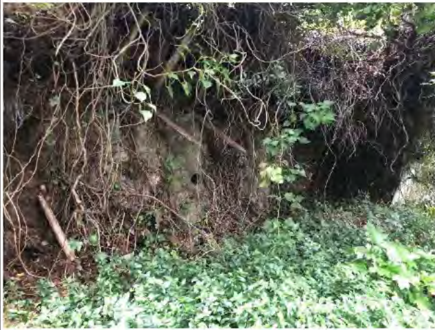
Photo 1) NAP-PRIS-RW14 view. Located below neighbouring residential property.
