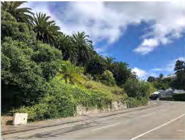
Photo 1) NAP-PRIS-RW21 view. Note Coote Road in foreground.
