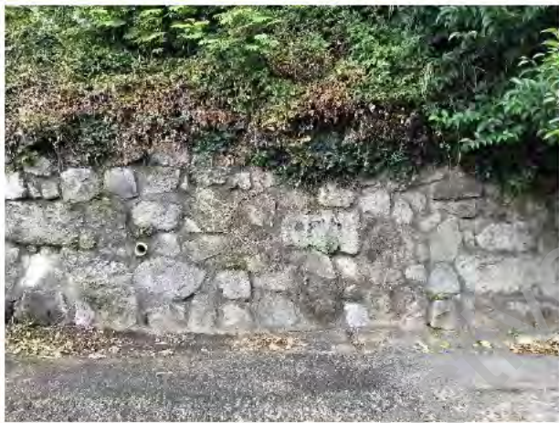
Photo 3) Retaining wall face and weep hole/drain
