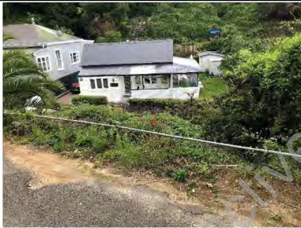
Photo 3) Erosion of driveway/asphalt and "channel" completely filled with soil.
