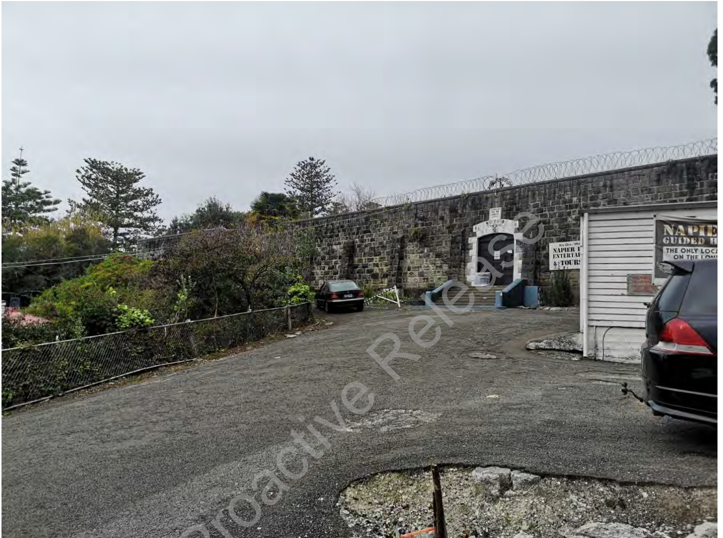
Site Identification Photograph – Northern Elevation of the Prison Wall (External)
