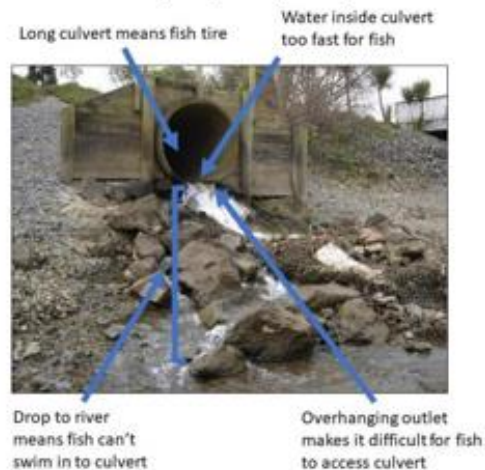
Figure 2-1: Example of a culvert that impedes fish movements.
