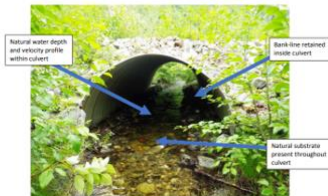
Figure 2-2: An example of a stream simulation culvert design.
