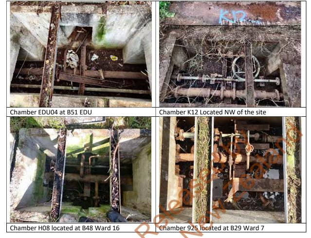
Figure 10: Representative Photos of the Concrete Ducting System
