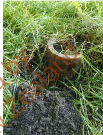
B3 – Ceramic pipe protrusion
