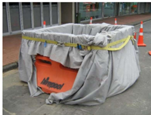
Figure 3: Top - Turkey’s nest made from filter socks; Bottom left: dewatering bag and pipe sock; Bottom right: mobile “turkey’s nest.”
