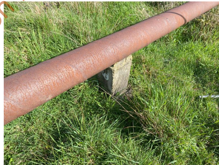
Southern pipeline with concrete pile
