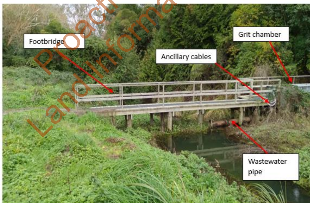
Figure 4: Infrastructure to be removed within the Wharekōrino Stream wetland.
