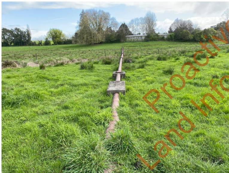
Southern pipeline with concrete casing
