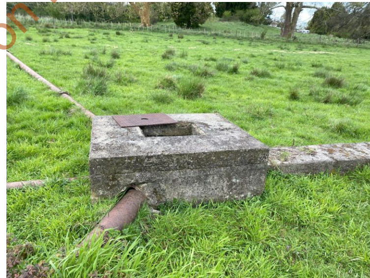
Concrete chamber connecting all four pipelines
