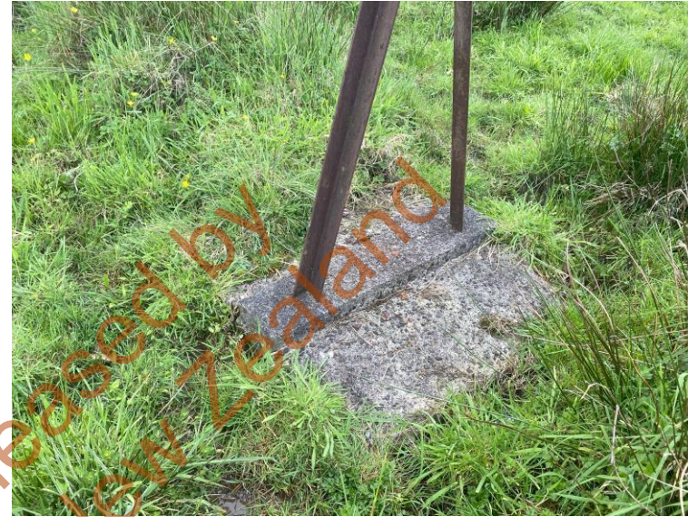
Southern pipeline footings and concrete foundation
