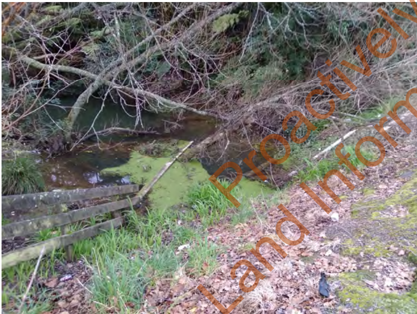
Culvert 1 Outlet – note extensive debris/windfall
