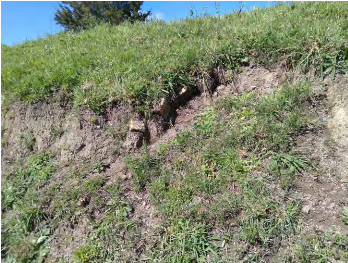
H6 – debris protruding
