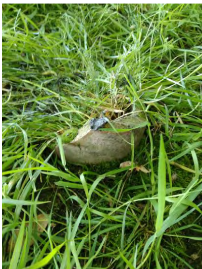
B3 – Ceramic pipe protrusion
