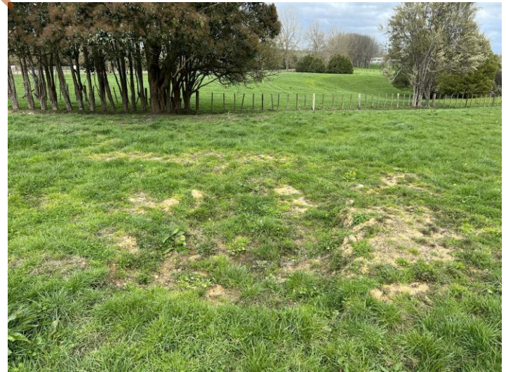
B5 - Trench Subduction, Minor Ponding
