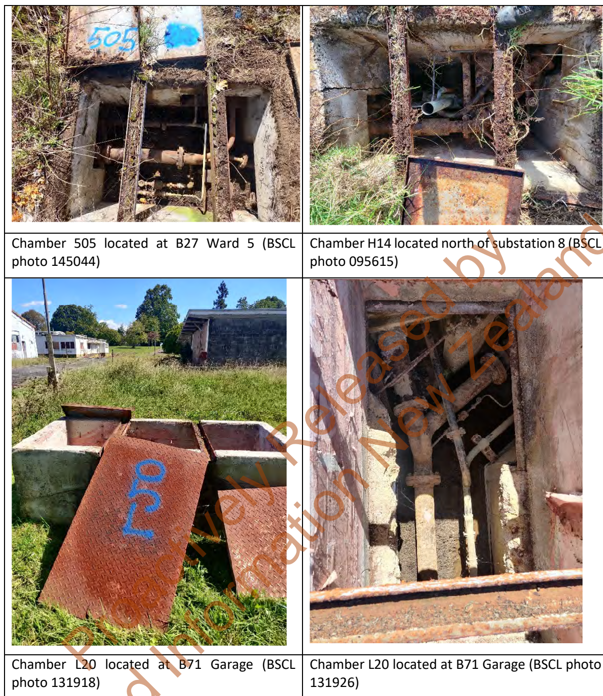
Figure 18: Photos of the Concrete Ducting System
