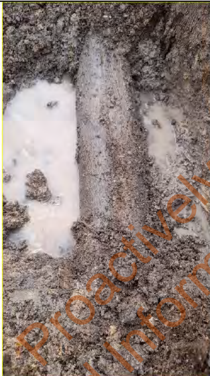
180mm diameter AC pipe exposed during hydroexcavation at location 17, refer to Civtec documents.
