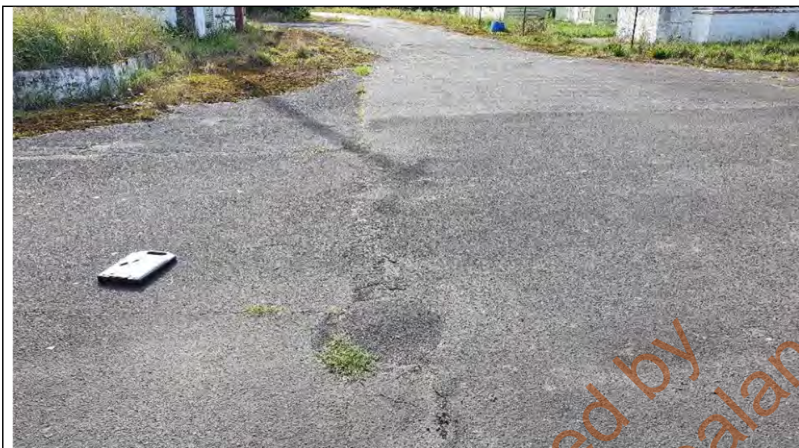
Figure 7: Typical joint without seal
