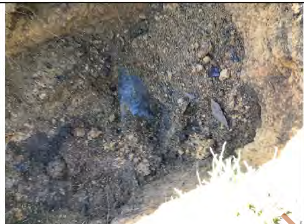
Pothole in southern area of site adjacent to fire hydrant: 100NB AC pipe at 1.2m depth.
