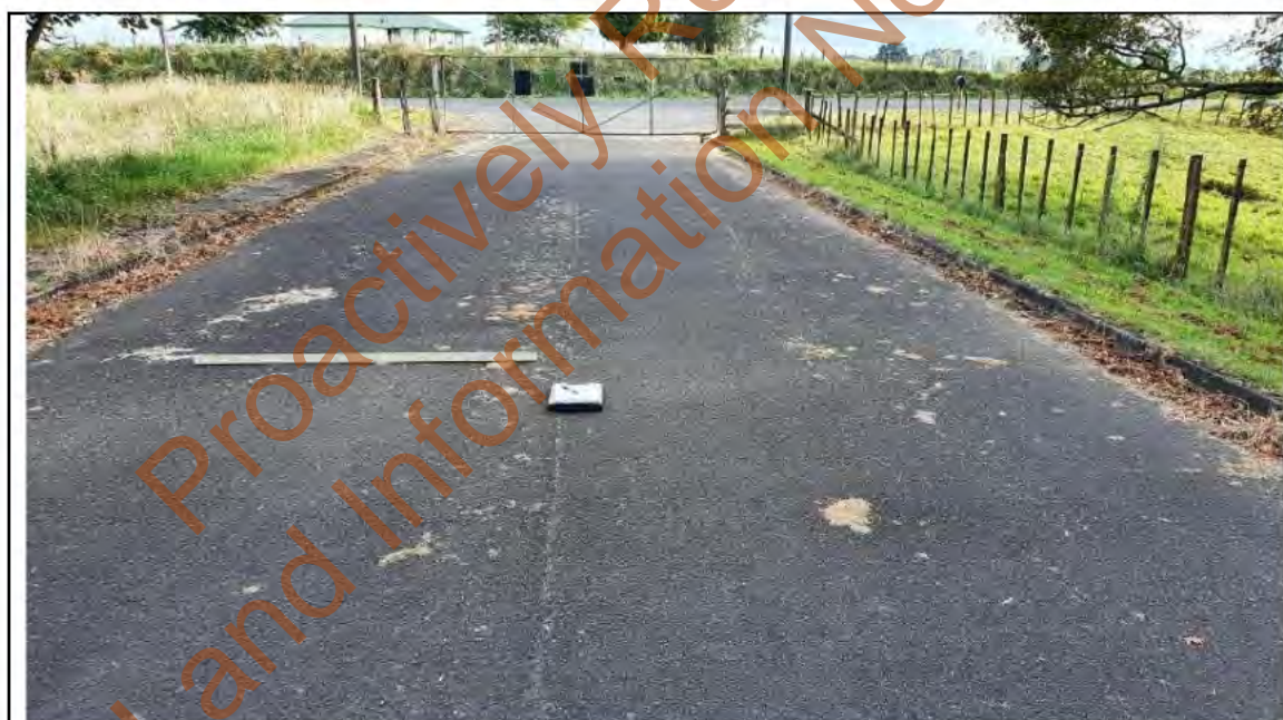
Figure 4: Typical good dual cross-fall, kerb and channel but overgrown
