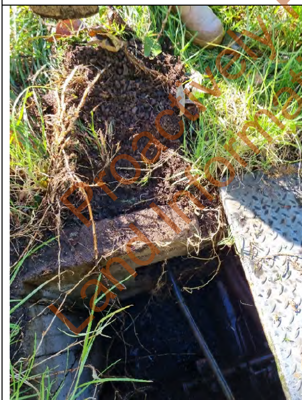
Chamber – LID K01 showing 50mm cover where the duct connects to the building
