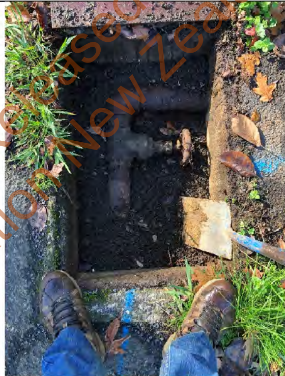
Inspection of a valve chamber at the northern area of the site showing heavily pitted and corroded pipes.
