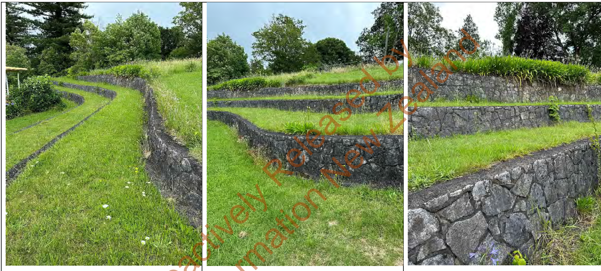
Figure 14: Three views of retaining wall showing the terraces and its general condition
