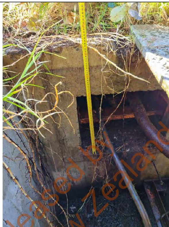
Chamber – LID K01 located at B55 Ward K showing the internal duct height as 500mm
