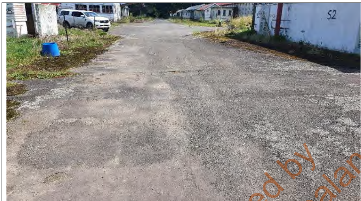
Figure 5: Typical settlement at service trench road crossings
