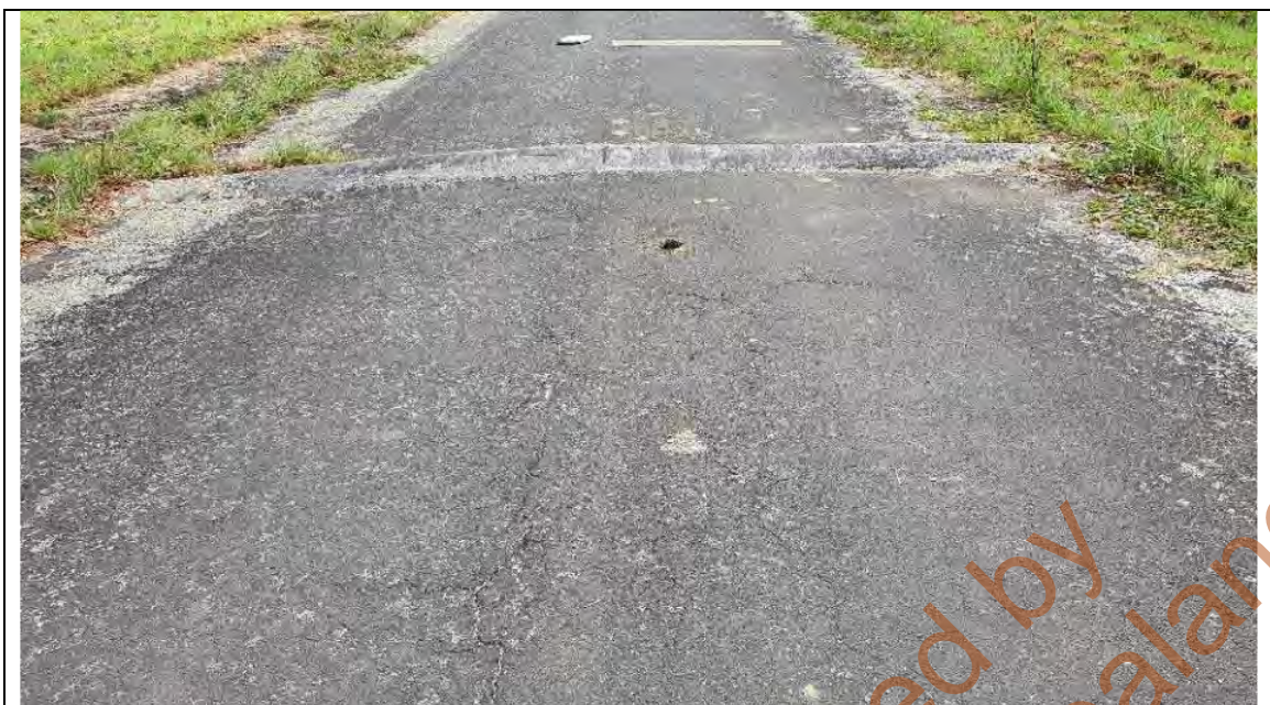
Figure 9: Typical speed hump
