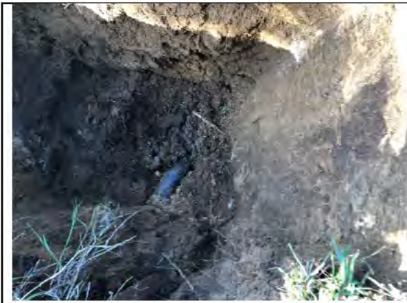
Pothole adjacent to fire hydrant. 150NB (200OD) Ductile Iron Pipe found at approx. 1m depth. Pipe wrapped in denso tape.
