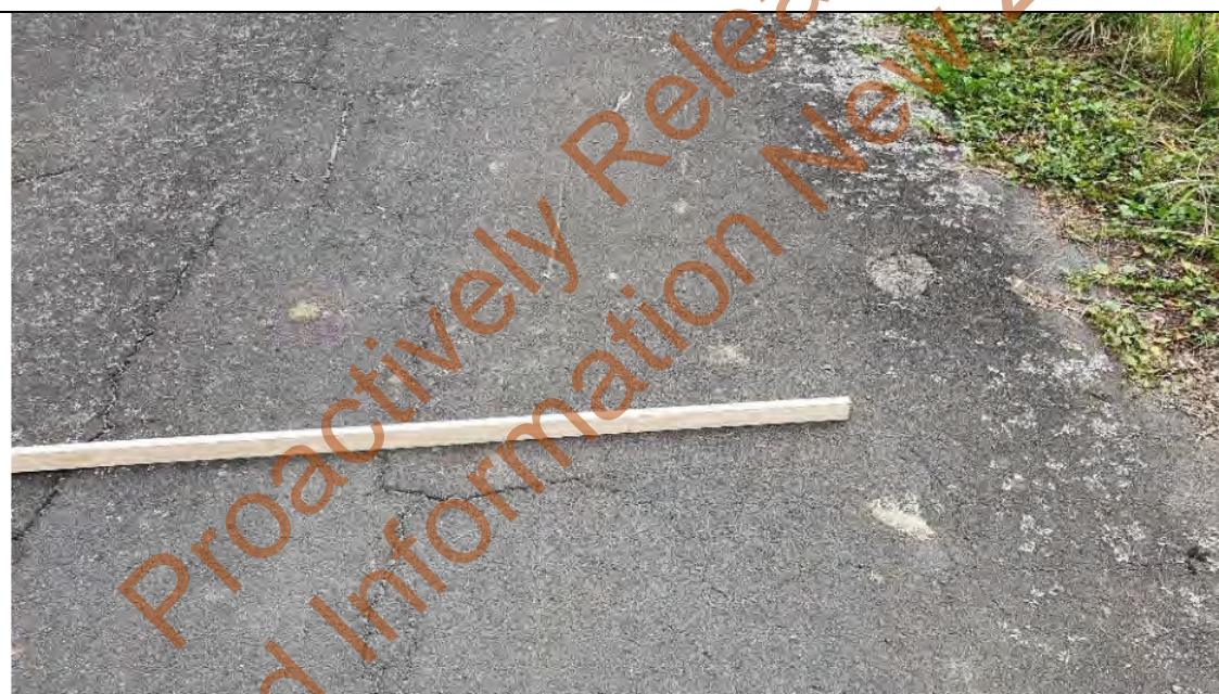
Figure 5: Typical settlement at service trench road crossings
