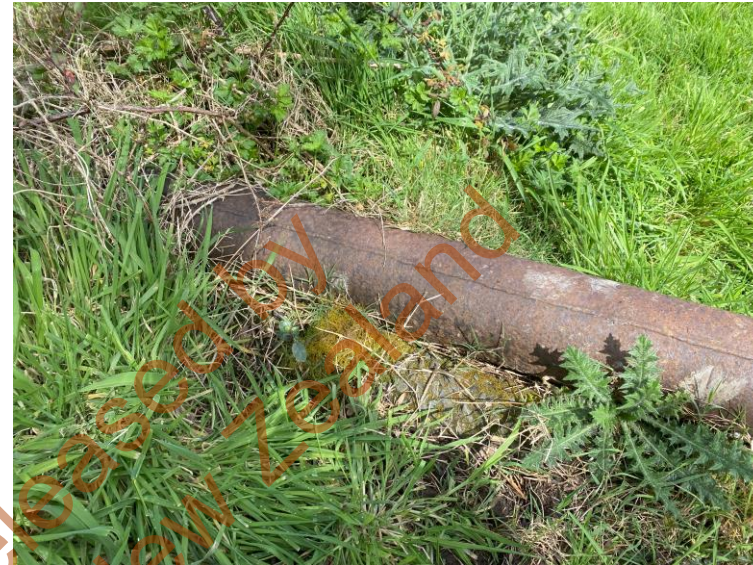
Pipeline situated on concrete foundation
