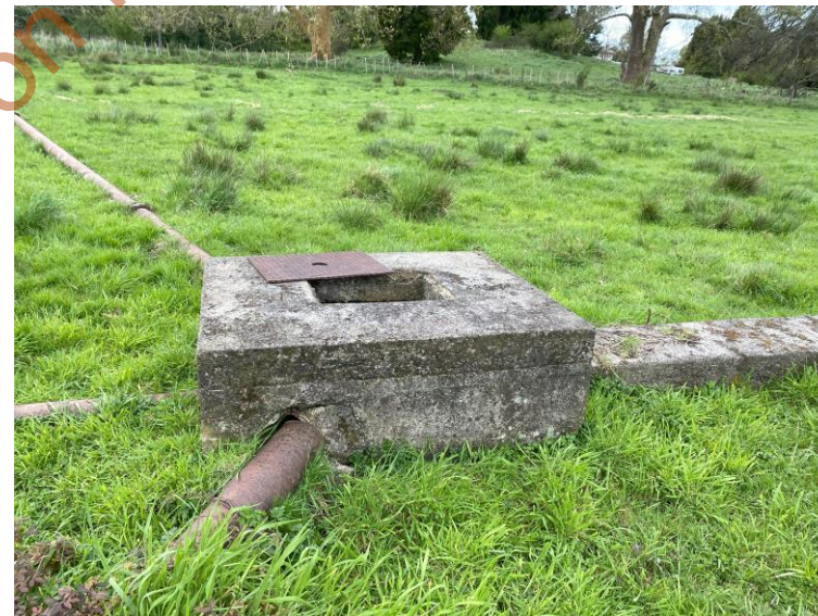
Concrete chamber connecting all four pipelines
