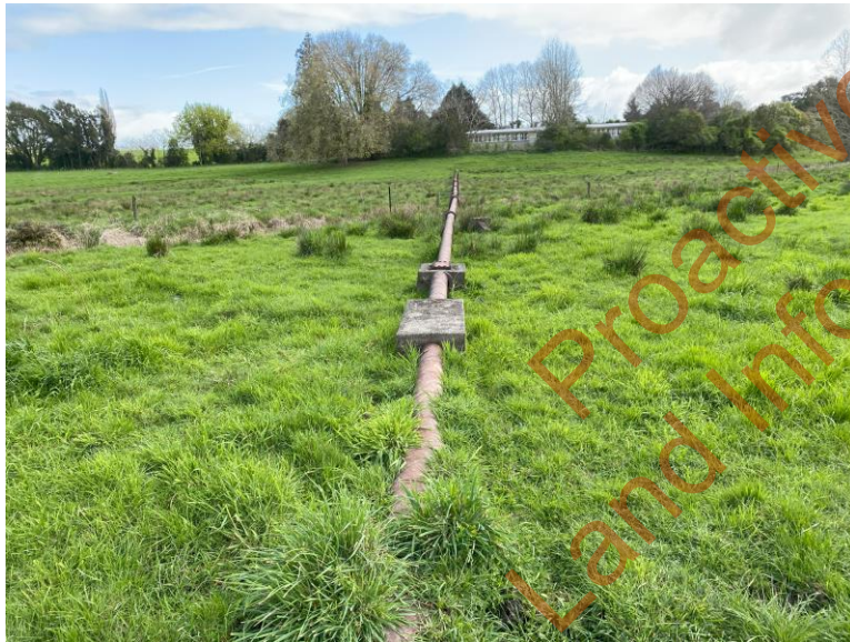
Southern pipeline with concrete casing
