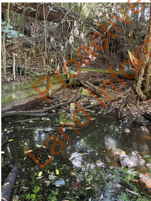
Figure 5: Inlet of Culvert 2 with Pooled water and debris directly upstream.
