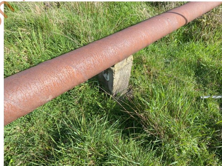
Southern pipeline with concrete pile
