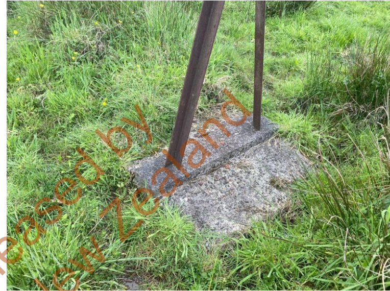
Southern pipeline footings and concrete foundation
