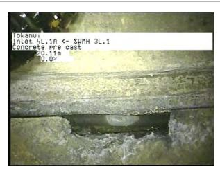
MH 3L.1 To 4L.1A Inlet\_87e499ee-67c2-4bf4-9c4e-d0c141d2ad9f\_20230406\_14 3037\_117.jpg, 00:05:22, 20.11m
