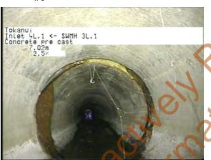
MH 3L.1 To Outlet 4L.1\_e4161afd-e948-44e2-a649-42ff507c516a\_20230406\_12 4650\_316.jpg, 00:01:54, 7.02m
