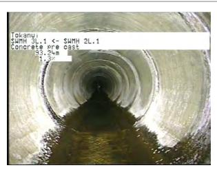
MH 2L.1 To MH 3L.1\_e1d52d70-a10c-49b9-82e1-83502db2b1e9\_20230406\_1 22921\_487.jpg, 00:29:01, 93.24m
