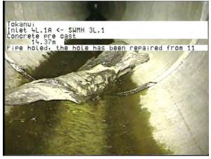
MH 3L.1 To 4L.1A Inlet\_0a5fc193-8175-4f24-b7fc-62fa2161c2dc\_20230406\_142 911\_003.jpg, 00:03:51, 14.37m
