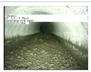
CP J.1 To Main\_2371c38a-bcb7-4626-a41b-950699dc0b05\_20230327\_1 30504\_662.jpg, 00:07:18, 19.96m
