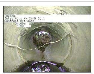
MH 3L.1 To Outlet 4L.1\_11e4b69d-76b0-48b6-869b-82ee541d92a4\_20230406\_1 25256\_863.jpg, 00:07:33, 24.60m
