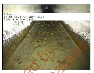
MH 3L.1 To Outlet 4L.1\_8e005ace-6982-4f74-a075-611227db762a\_20230406\_1 24600\_011.jpg, 00:01:16, 3.62m
