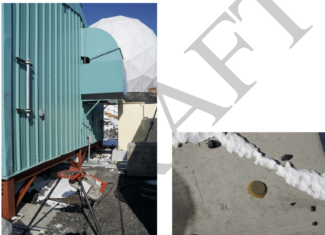
Figure 2.3: Radarsat building 71 and benchmark at Radarsat Station. The benchmark is located on the pillar on the lower left corner of the left picture.
