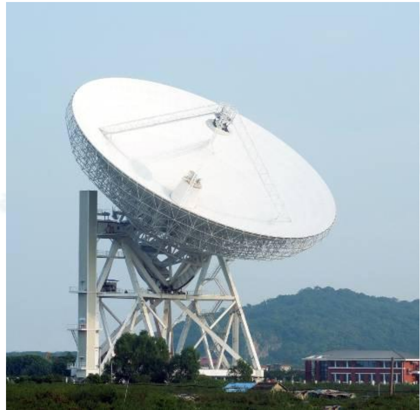
65m Antenna ( L, S/X, C, X/Ka, Ku, K, Q bands) for Shanghai Astronomy Observatory
