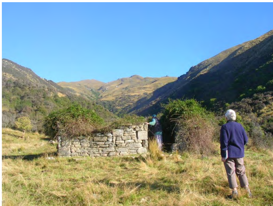
Figure 1. View up Last Creek showing the historic boundary-rider's stone cottage at ~400m just beyond the mouth of lower gorge. Although the walls are intact there is a dense cover of climbing Pohuehue ( Muehlenbeckia australis ) over the collapsed roof. AFM photo. April, 2012
