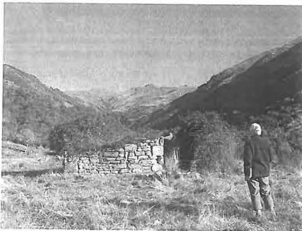
Fig. 1. View up Last Creek showing the historic boundary-rider's stone cottage at ~400m just beyond the mouth of lower gorge. Although the walls are intact there is a dense cover of climbing Pohuehue ( Muehlenbeckia australis ) over the collapsed roof.
