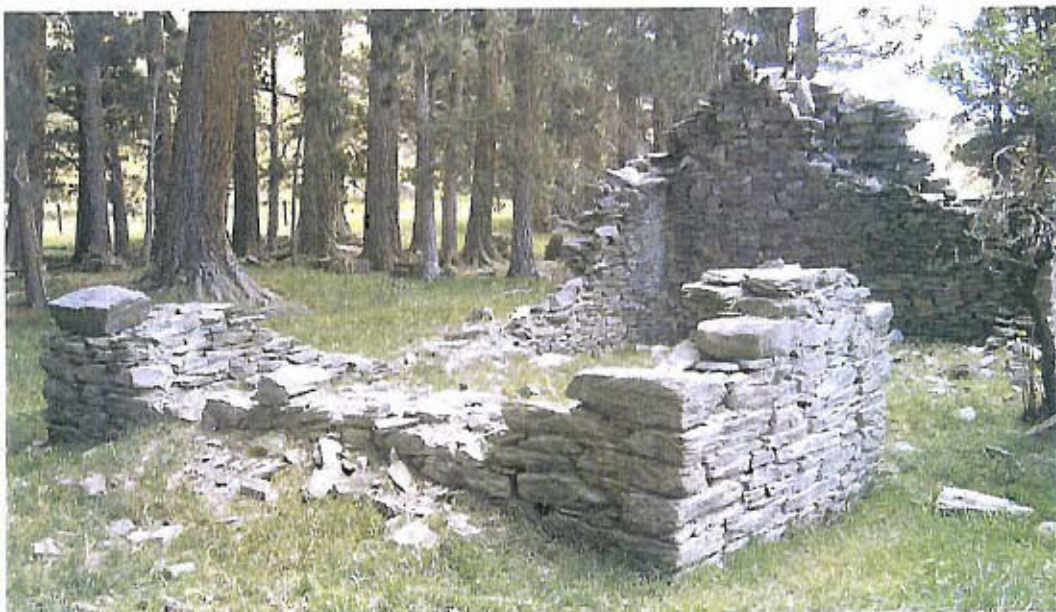
Photo 17: The remains of a large schist hut (also at site 8), which may have been built circa 1870, consisted of two rooms and probably was largely intact in the 1930s. Over the last 80 years stone has been removed for other building projects.
