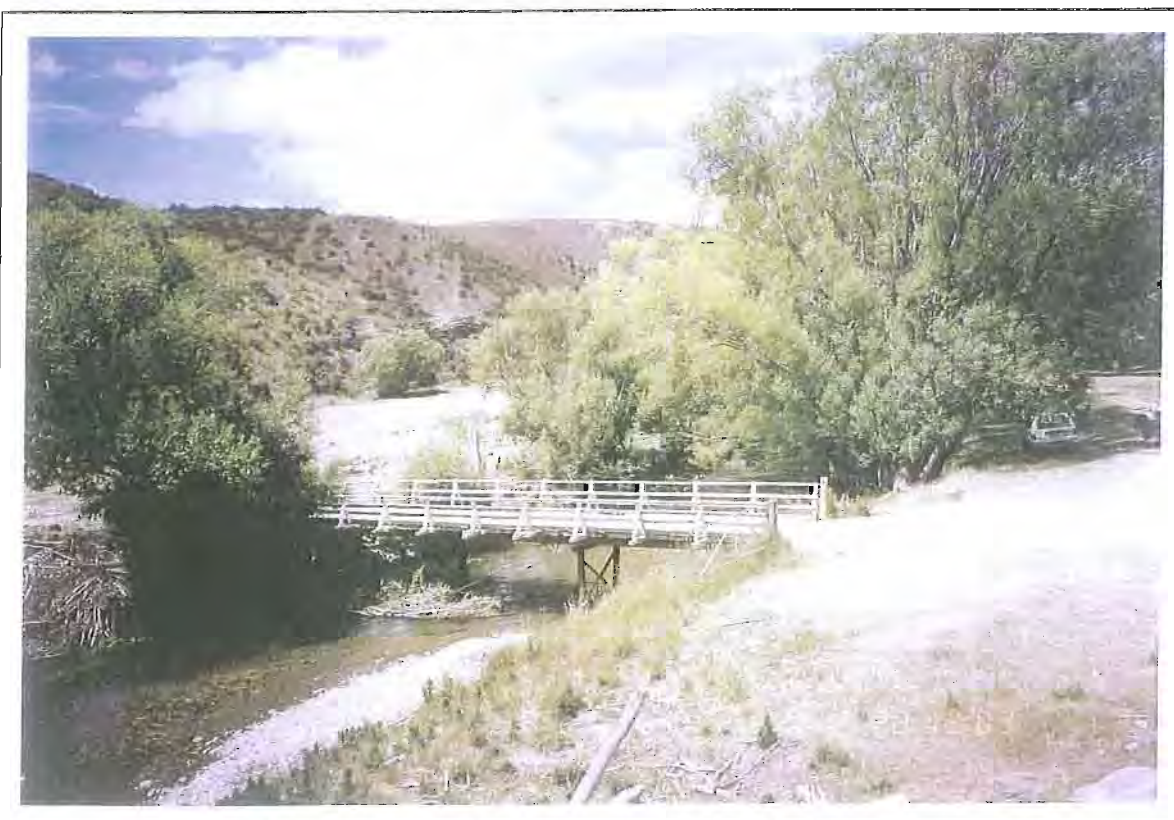
Fig. 12 The Cluden Bridge over the Lindis River not only gives access to the Cluden Stream and its valley, but is also a convenient starting point for gentle walks along the banks of the Lindis River. Although marginal strips have been laid off, in places these are not wide enough to negotiate bluffs and wetlands adjacent to the river. Appropriate widening should be included in the tenure review provisions.
