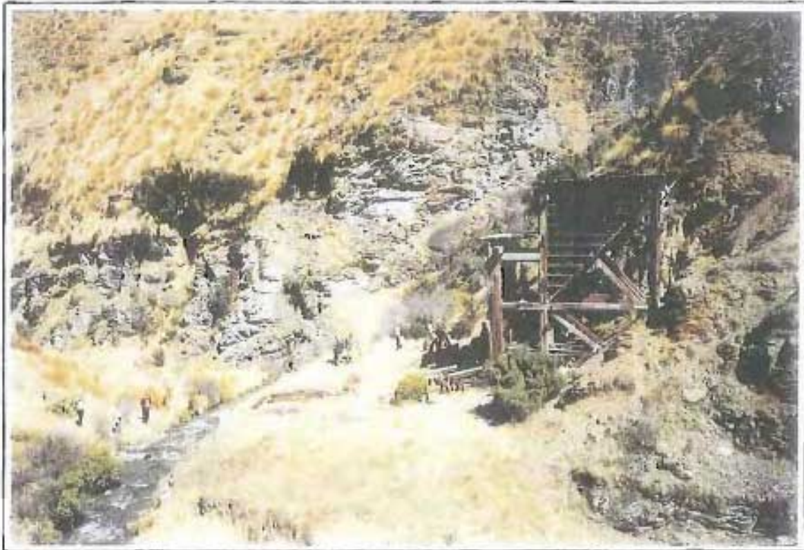
Fig. 17. The existing Reserve does include the beautifully restored Homeward Bound battery with its huge wooden hopper which fed gold-bearing ore into the crusher. The site is only about a half-hour walk from Macetown but is very close to the upper limit of the Reserve. Even the remains of the cableway which brought the ore down from the mine is excluded from the existing reserve.
