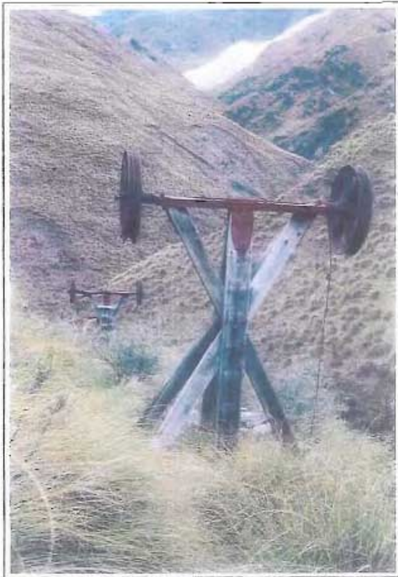
Fig. 19. The former cableway which transported the gold-bearing ore from the mine high above the valley to the Homeward Bound battery in the Rich Burn is worth exploring to understand the lengths to which the miners would go to win their riches.
