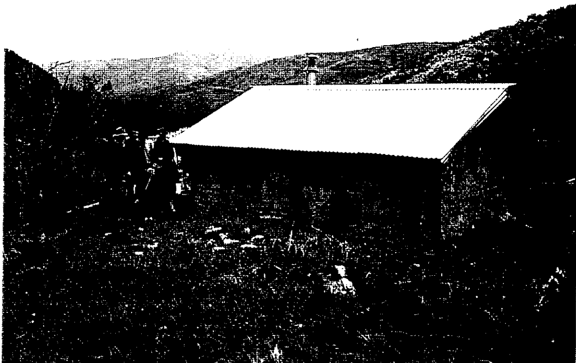
Glenlapa Station Reconstructed raceman's hut near the Muddy terrace water race.
