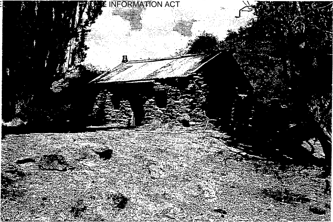
Photo # 5. Stone miner's hut in Duffers Creek, well worthy of protection. Also well worth a walk to inspect..
