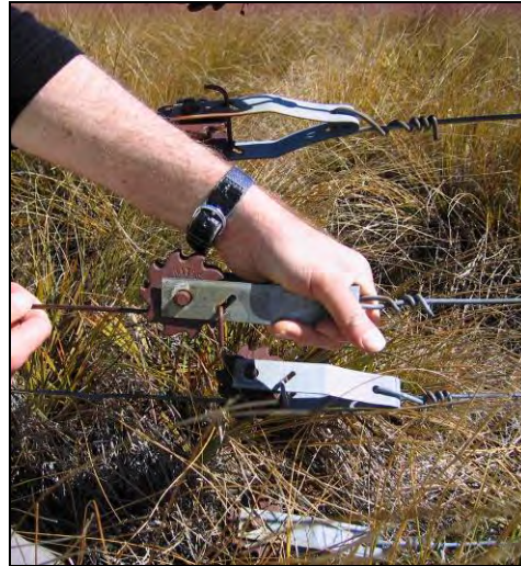
Plate 2. Hayes strainers on internal fence line ca.1050m contour at GPS 041.
