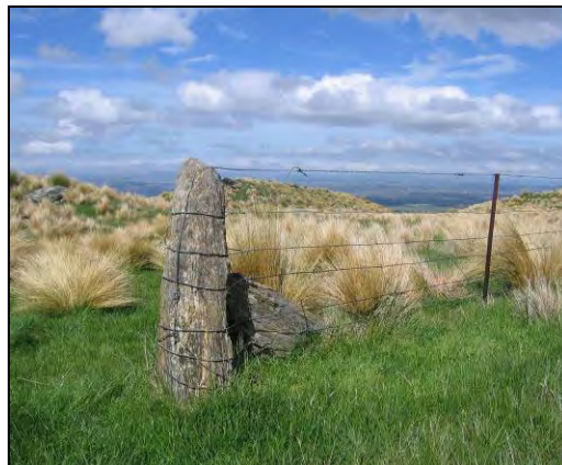
Plate 4. Restored 19 th C fence line incorporating schist uprights and flat standards at GPS 049.
