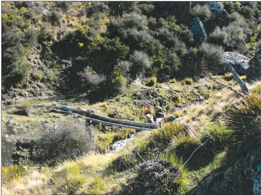
Photo 14. Fluming pipe across Duohys Gully (GPS 028) above Towans Camp. View South - West.
