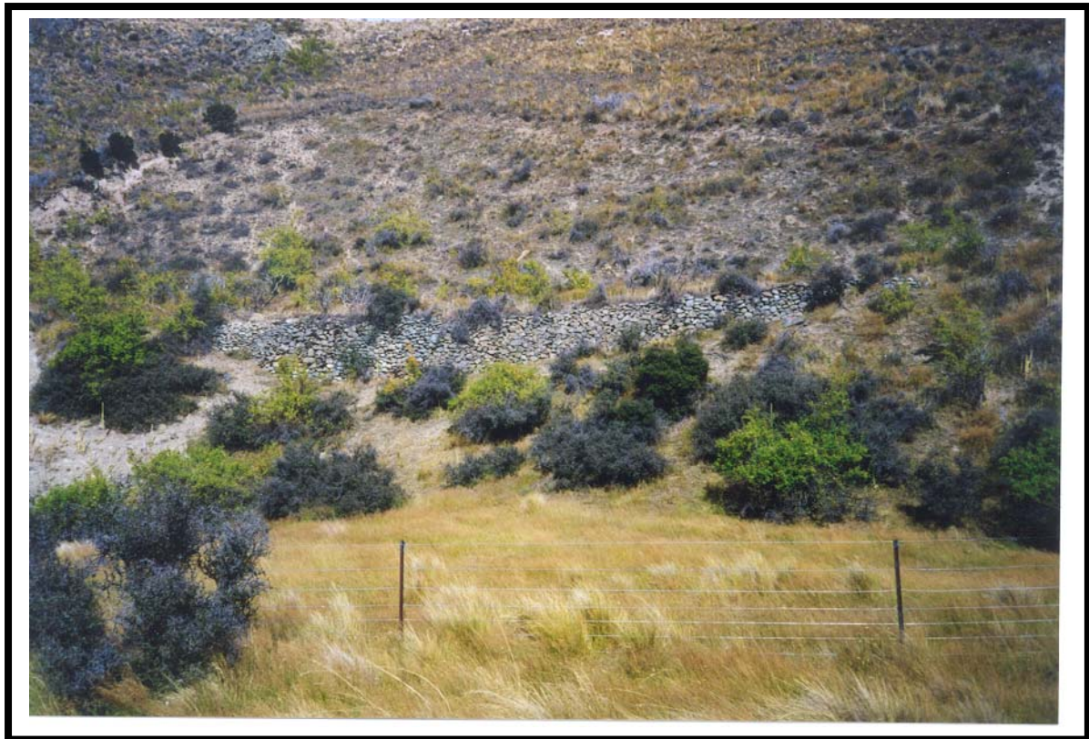
Photo Four. Revetted Section of the Scandinavian Water Race
