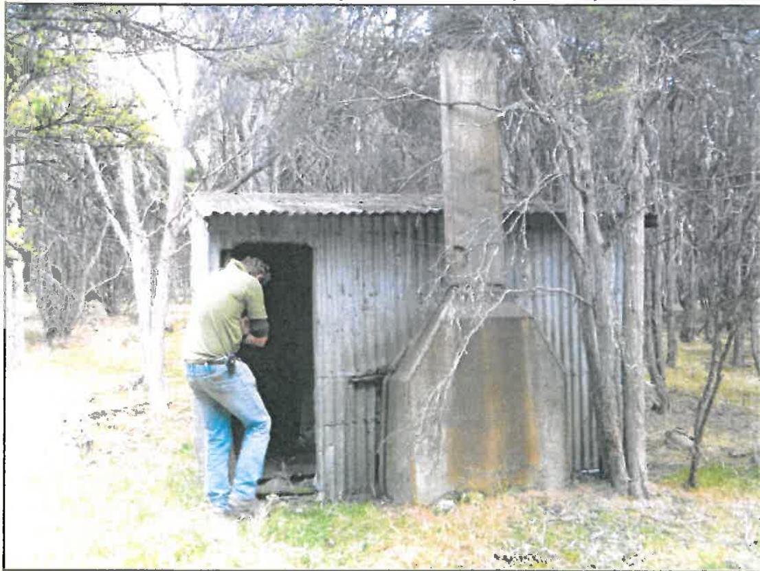
Tin hut with kanuka pole framing and external metal chimney, Bell's Creek (GPS 032)
