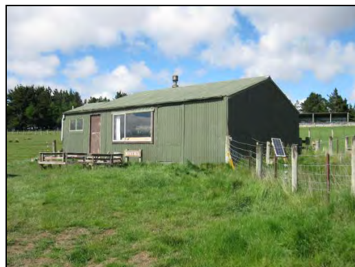
Plate 6. Modern replacement Scout Hill hut (GPS 001) and stock yards. View west.
