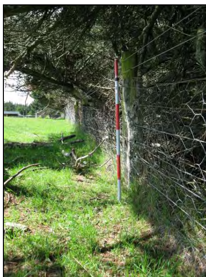
Plate 21. Natural split post bored 7 hole at Scout Hill stock yards (GPS 002).
