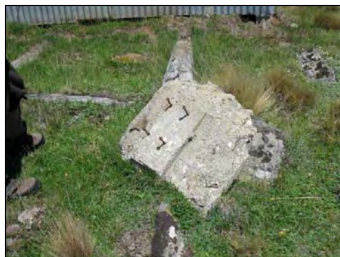
Plate 18. Concrete lump with bolts embedded.
