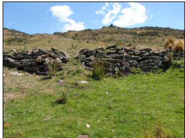
Plate 9. Front wall of Gray's Dam above Gray's Hut site
