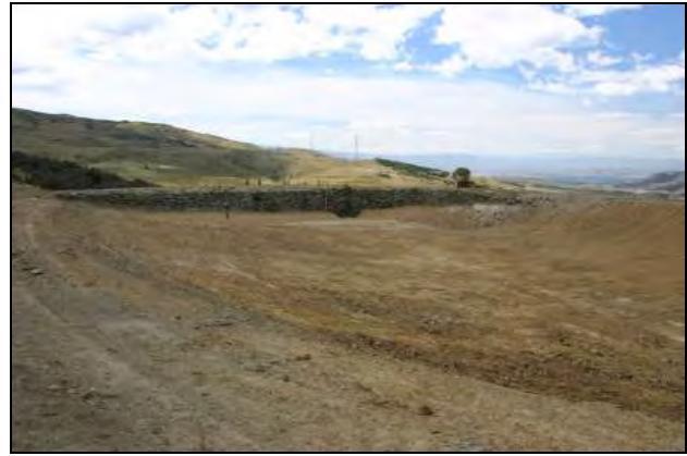
Plate 7. Last Chance Dam
