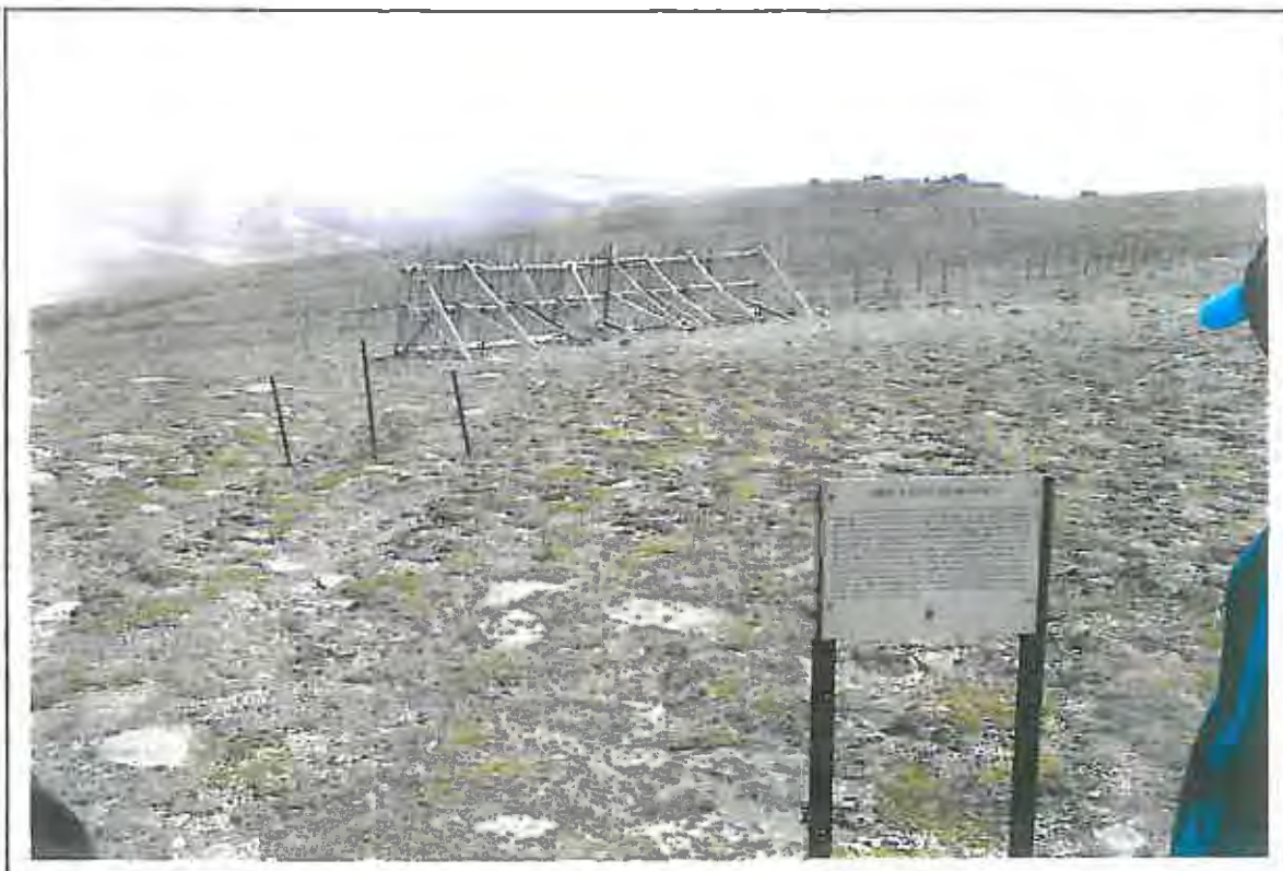
Fig. 11 An experimental snowfence was built in 1959 by the Otago Catchment Board to test the capture of snow which, after melting, could augment the water yield of the Fraser Basin, rather than blowing over the crest of the Old Man Range. The fence has stood the test of time and recent signage explains the purpose of the structure to interested visitors to the Kopuwai Conservation Park.
