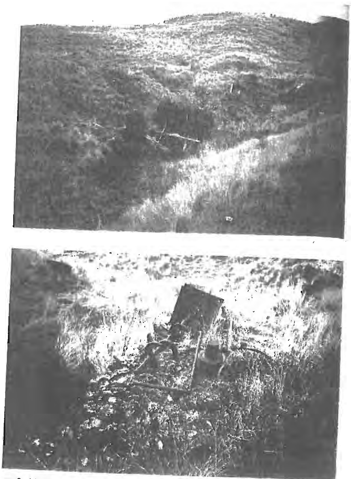
Figure 6. 11. Remains of two stamper-batteries on the Old Man Range. Upper: Small structure that probably housed the Pelton wheel which drove Syme's last battery. Lower: 3-head stamper camshaft and stamper shoes probably from Exhibition battery.
