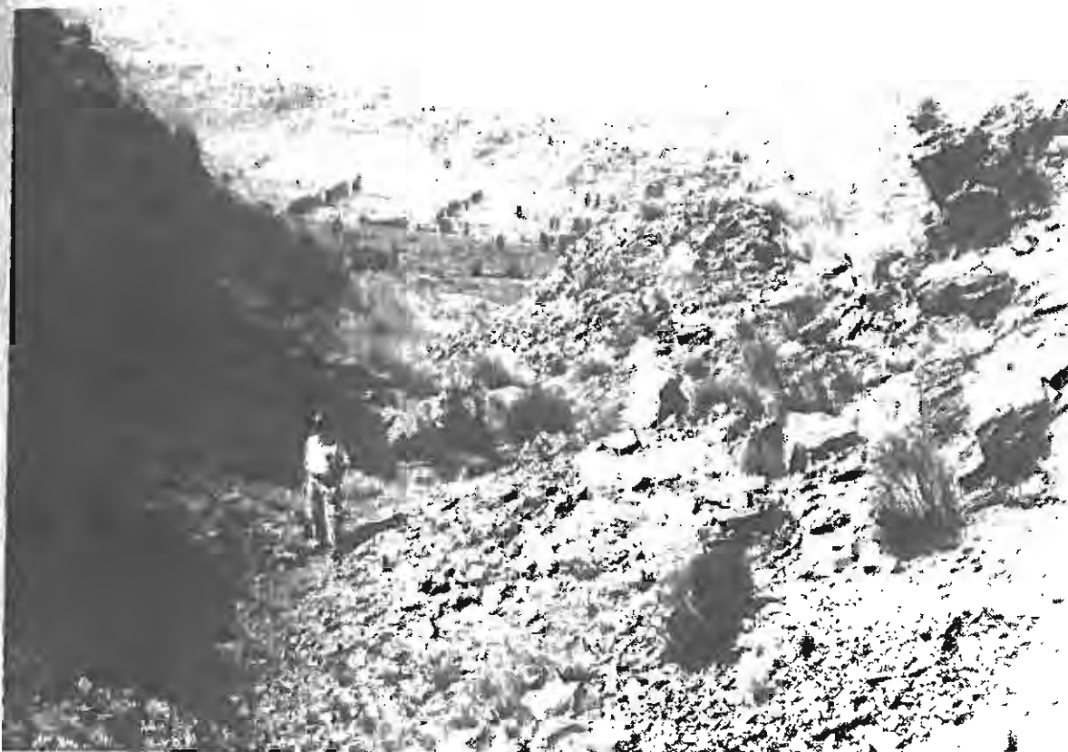
Figure 6. 13. Sluicing the reef material left this large trench, about 80 metres long and 6 metres deep. It cuts right through the ridge and is the most conspicuous feature of the Excelsior mine today.
