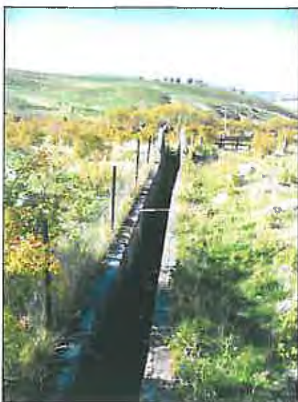
Photo 10. Sheep Dip (GPS 132). View South.
