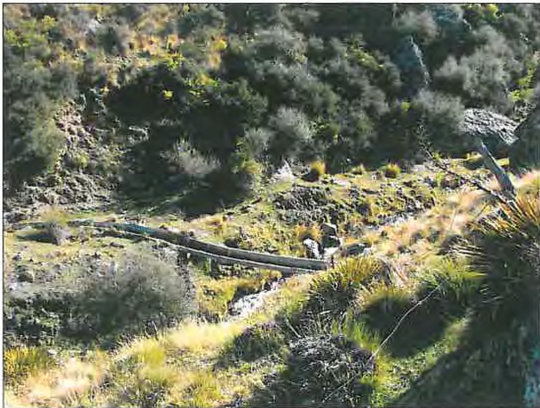
Photo 14. Fluming pipe across Duohys Gully (GPS 028) above Towans Camp. View South - West.
