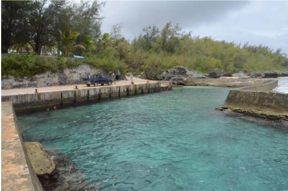
Figure 18 : The Main Landing at Taunganui
