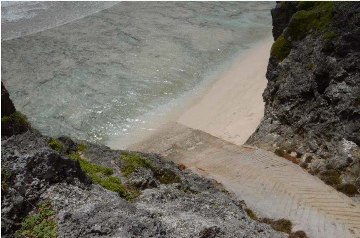
Figure 19 : The Steep Concrete Ramp Comprising the Second Landing at Aitu
