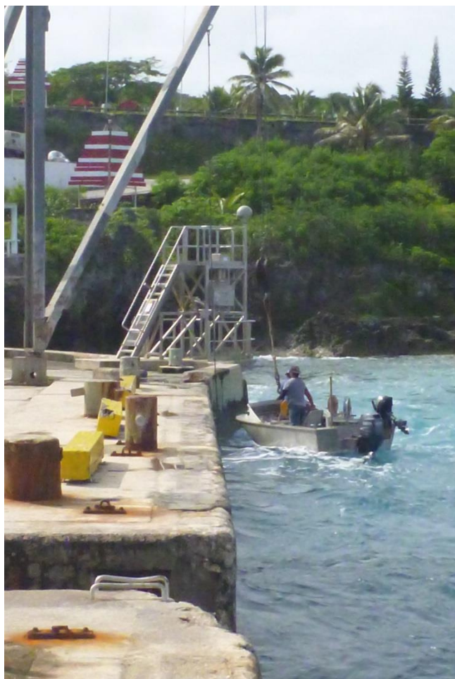
Figure 10: Alofi Wharf showing lead daymarks, BOM tide gauge and fishing boat preparing to be hoisted on wharf derrick
