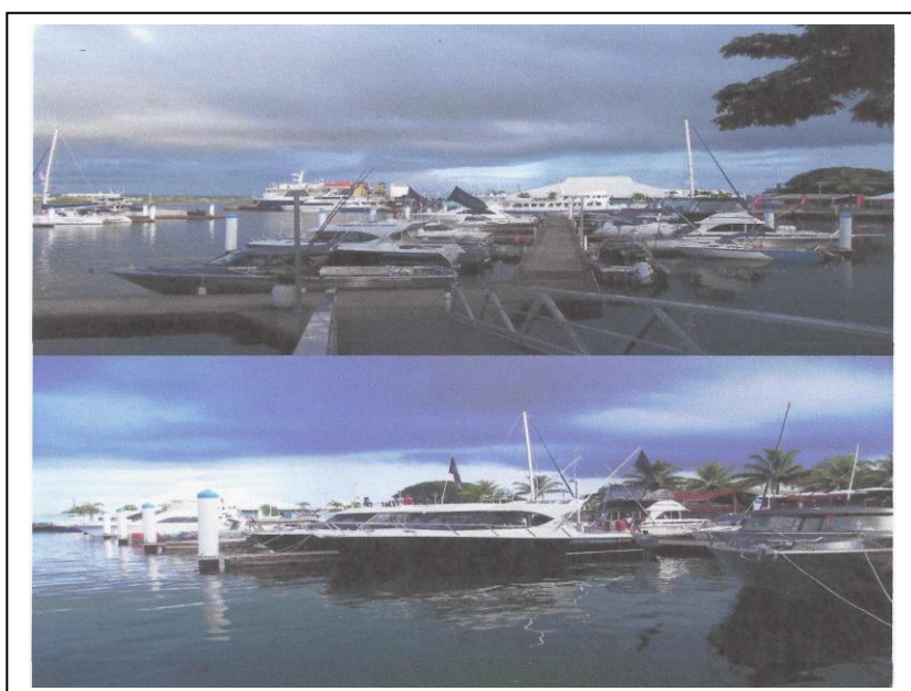
Figure 37: Apia Marina prior to cyclone damage (Source: Samoa Ports Authority)
