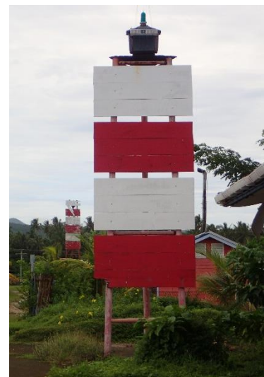
Figure 72: Aleipata Leading beacons (rear beacon light missing)
