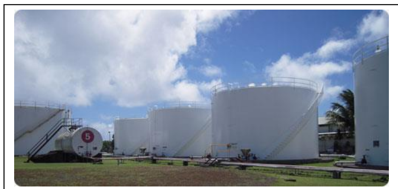
Figure 44: Petroleum Storage Tanks at Sogi Terminal (Source: PPS)
