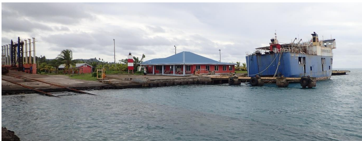
Figure 70: Aleipata Port – slipway, front lead, terminal & wharf ( Lady Samoa II being dismantled)
