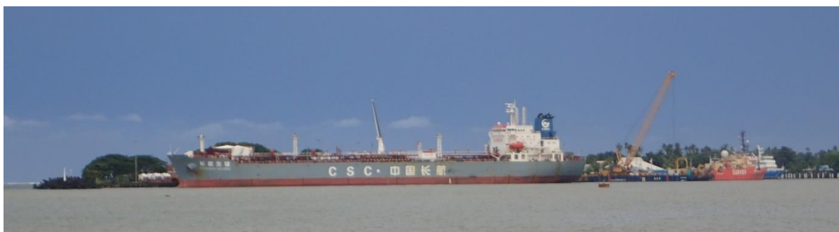
Figure 42: Fuel product tanker discharging at Main Wharf
