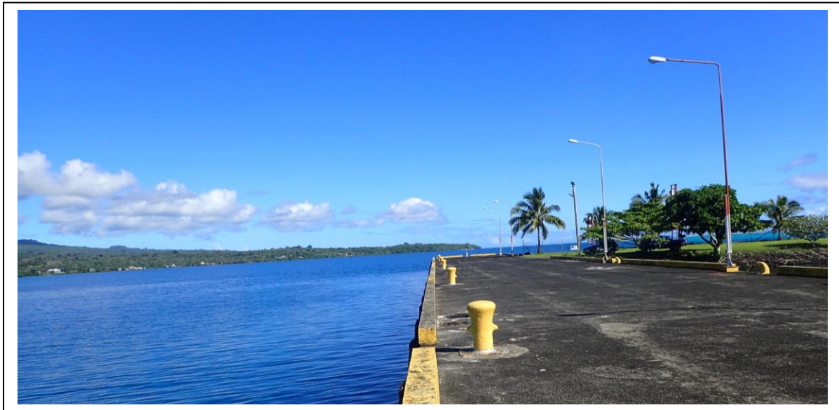
Figure 69: Asau wharf looking west
