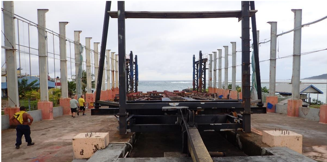
Figure 71: Aleipata slipway looking to the entrance channel
