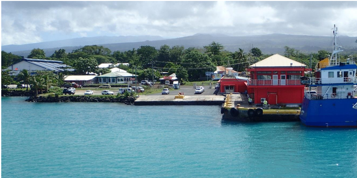
Figure 61: Approaching the ramp and wharf at Salelologa
