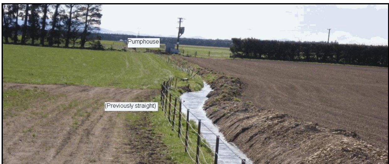
Figure 3 – Effects of fault rupture on previously straight fence and water race. (Photo - Survus Consultants)
