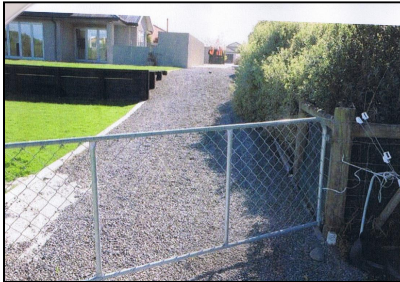
Figure 6 – Boundary point has moved 2.8 metres due to lateral spreading as a result of liquefaction (Photo - Eliot Sinclair and Partners)
