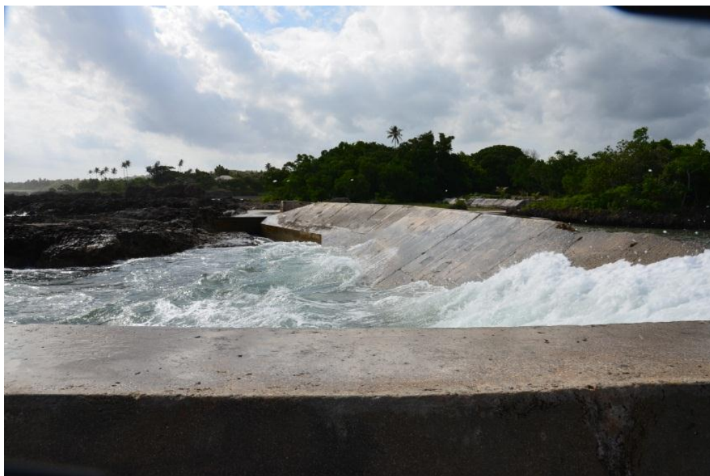
Figure 4-6 : Lénakel Wharf is Open to Significant Surge Loading
