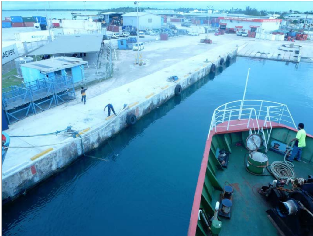
Figure 3: Berthing at No.3 of the Queen Salote Wharf, showing RoRo Ramp
