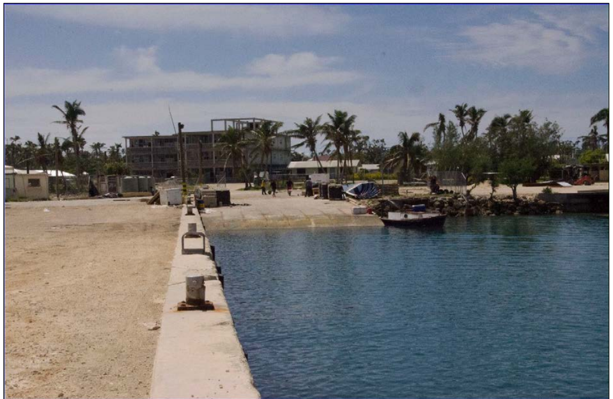
Figure 9 : Pangai Wharf, Ha'apai Showing RoRo Landing
