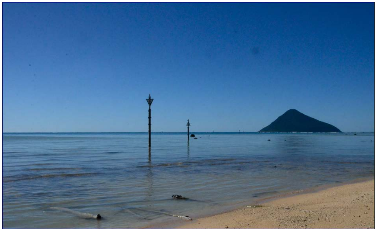
Figure 19: The Channel Entrance leading marks at Niuatoputapu Harbour (solar powered)
