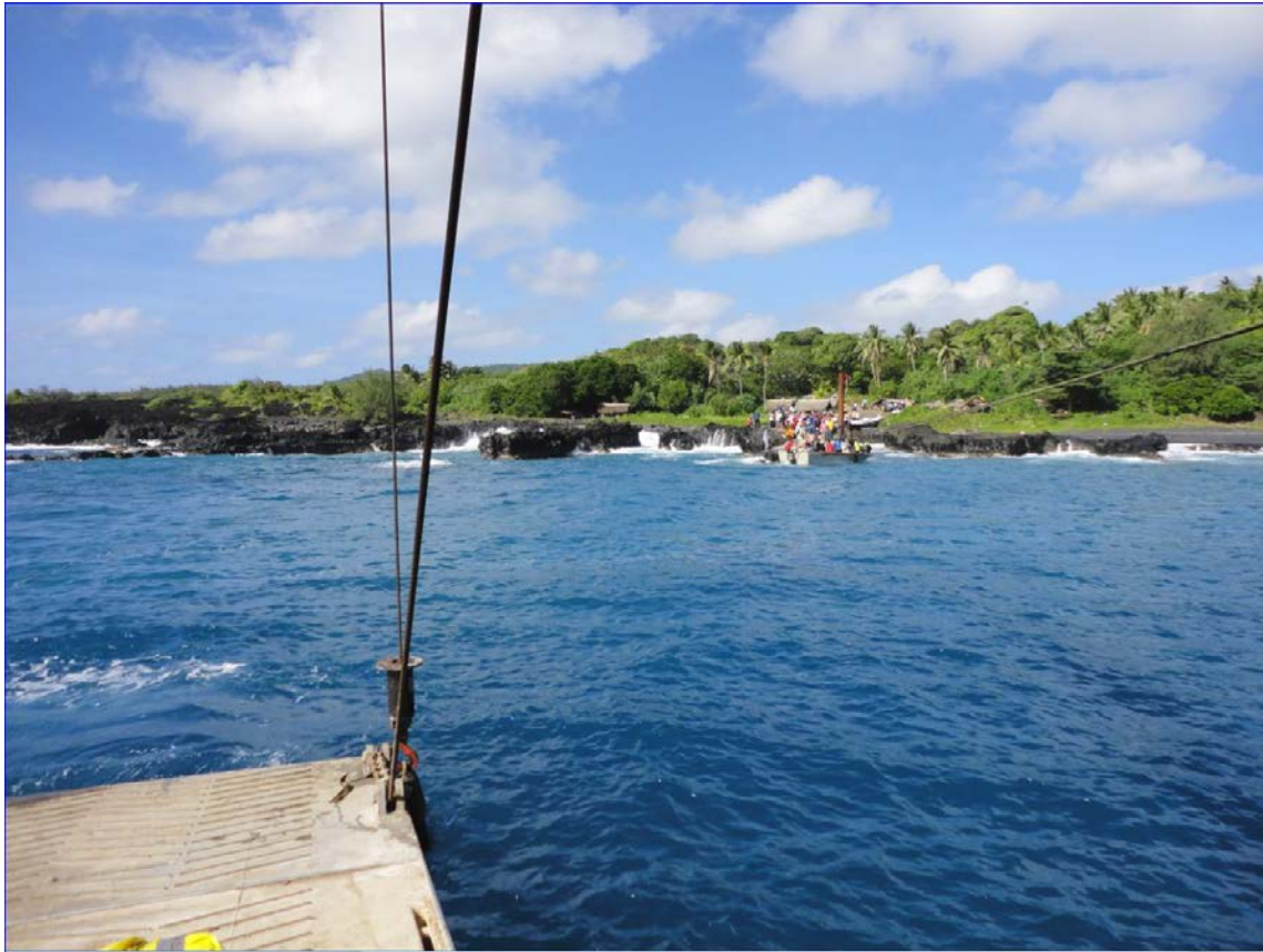
Figure 15: The Harbour Arrangements at Niufo'ou (Landing Stage Open to Sea)
