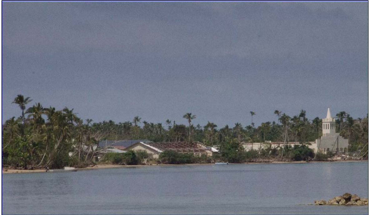
Figure 8 Cyclone Damage in Ha'apai was Extensive
