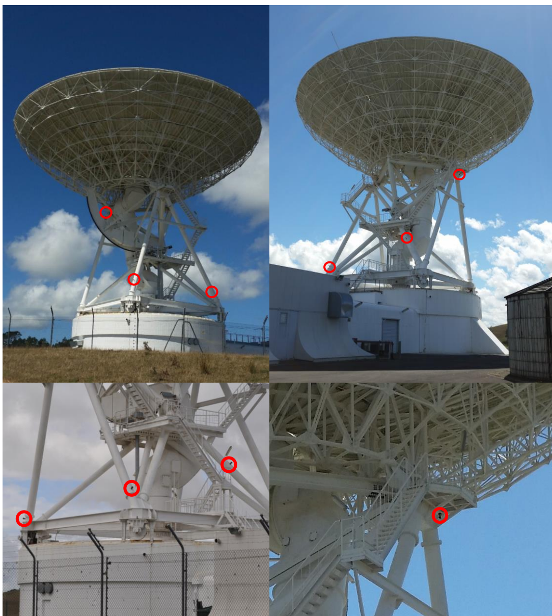
Figure 6.4: Target placement on the main structure of telescope in stall position. View from WAN3 (top left), looking from entrance to compound (top right) and close up of targets looking from WAS3 (bottom left) and close up of highest target (bottom right)
