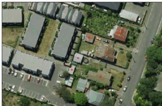
Roof material & condition
