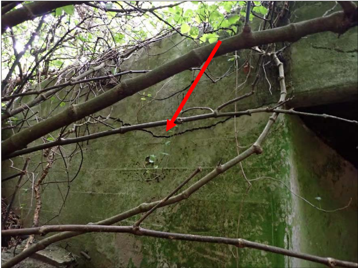
Figure 232, Feature 25: Fort Ballance. Cracking adjacent to opening at see-saw searchlight structure.
