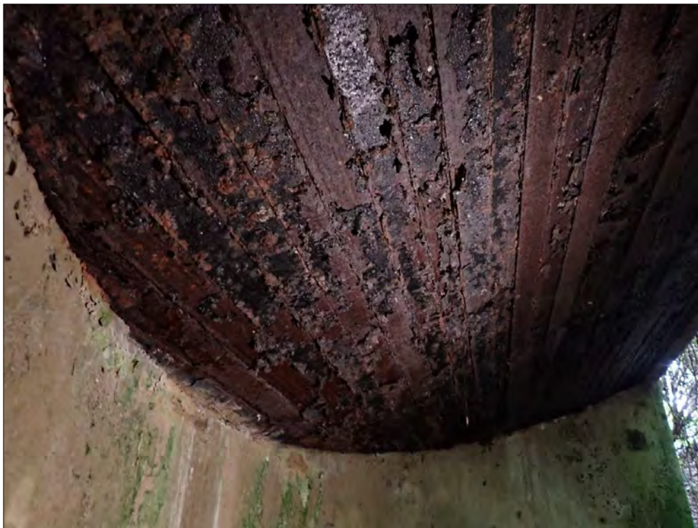
Figure 231. Feature 25: Fort Ballance. Steel formwork/reinforcement to underside see-saw searchlight structure.
