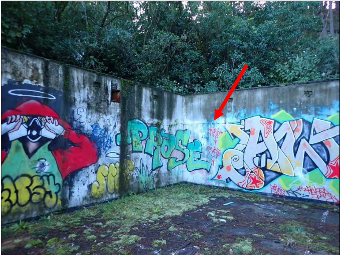
Figure 146. Feature 9: Magazine 9. Interior – Typical horizontal cracking to corners is indicated. Graffiti is present.
