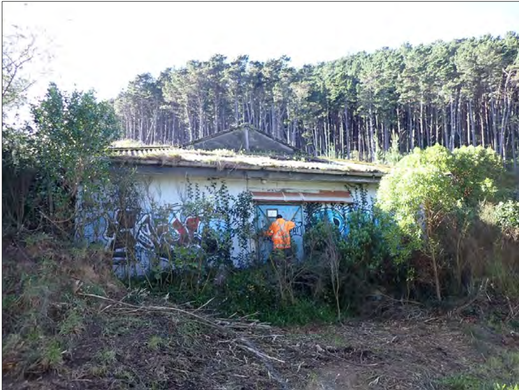
Figure 87. Feature 2: Magazine 2. Looking towards the western (front) elevation. Graffiti is present. There is vegetation on the roof and in the gutters, and the narrow loading deck is being ‘colonised’ by vegetation.
