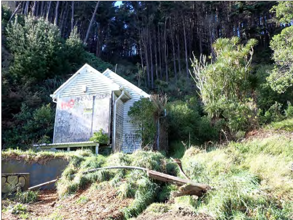
Figure 162. Feature 12: Former sergeant's house. Looking towards the western (front) elevation. Graffiti is present and openings have been boarded up. Vegetation is encroaching onto the house.
