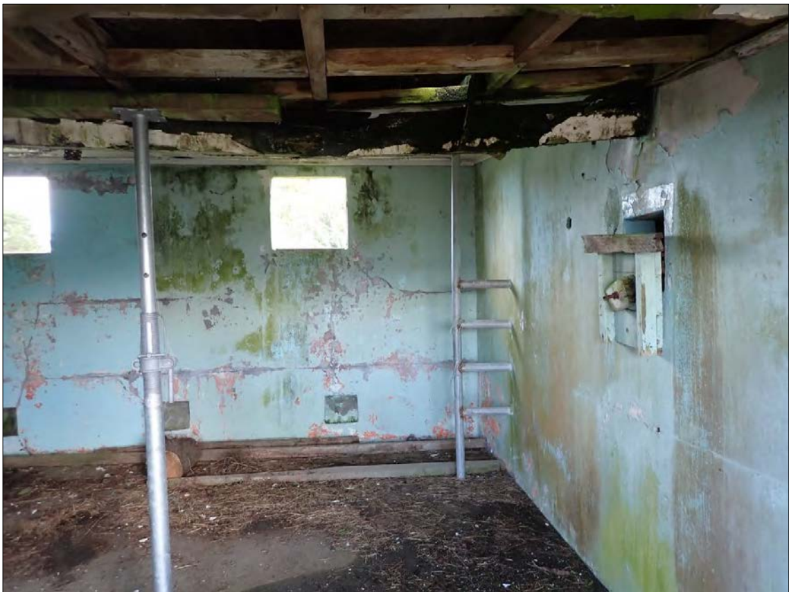
Figure 266. Feature 28: Farmstead. Milking shed interior. Roof being supported with an Acropop. Horizontal cracking is also evident.
