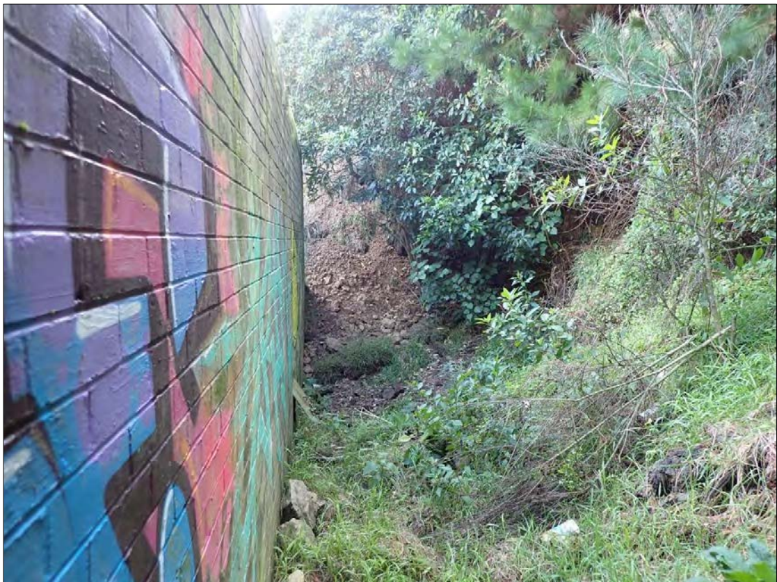
Figure 178. Feature 14: Magazine 11. Looking along the eastern (rear) elevation. A slip has occurred to the rear; and vegetation and debris has accumulated against the side of the structure.
