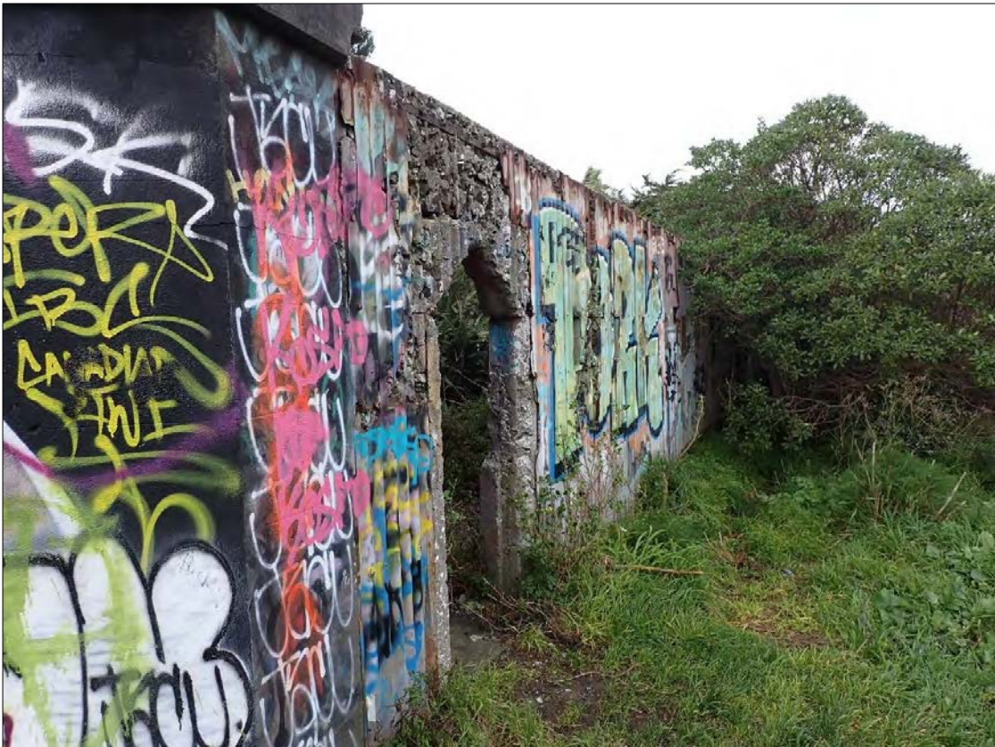
Figure 261. Feature 27: Fort Ballance. Loopholed wall to the east of the artillery barracks. Some corrugated metal formwork remains in position. The wall has been extensively graffitied.
