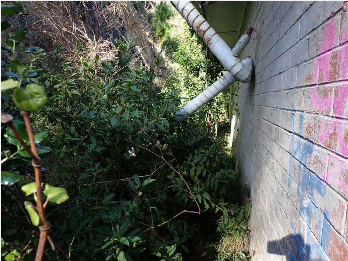
Figure 106. Feature 4: Magazine 4. Looking along the western (side) elevation. Debris and vegetation have accumulated against the structure. Graffiti is present.
