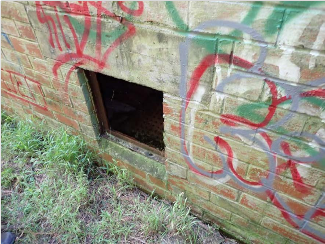
Figure 175. Feature 14: Magazine 11. Looking along the southern (side) elevation. Vent cover to passage between inner and outer wall of structure is missing.
