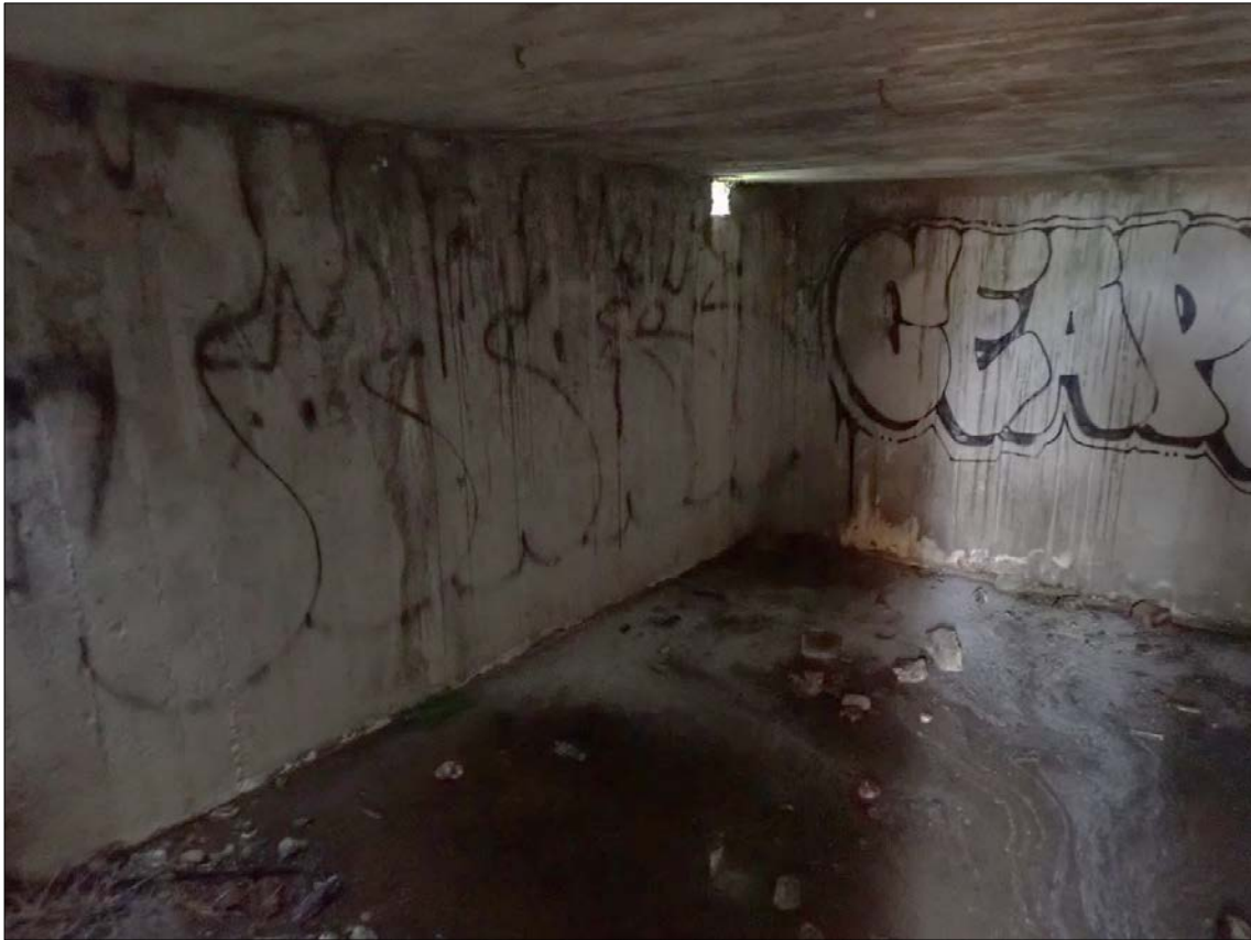
Figure 223. Feature 22: Mount Crawford Anti-Aircraft Battery gun emplacement. typical example of a chamber interior. Water is visible in a number of chambers. Graffiti is present.
