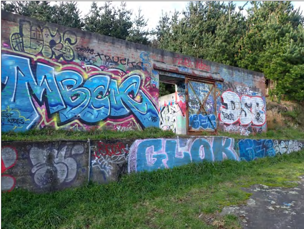
Figure 171. Feature 14: Magazine 11. Looking towards the western (front) elevation. Graffiti is present. The roof is missing.
