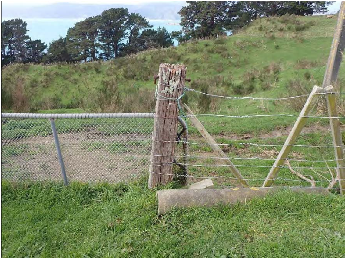
Figure 271. Feature 28: Farmstead. Example of early/original timber posts with gudgeon.
