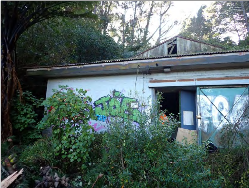
Figure 129. Feature 8: Magazine 8. Looking towards the western (front) elevation. Graffiti is present, the hipped gable is damaged, there are no gutters, and the narrow loading deck is being 'colonised' by vegetation.
