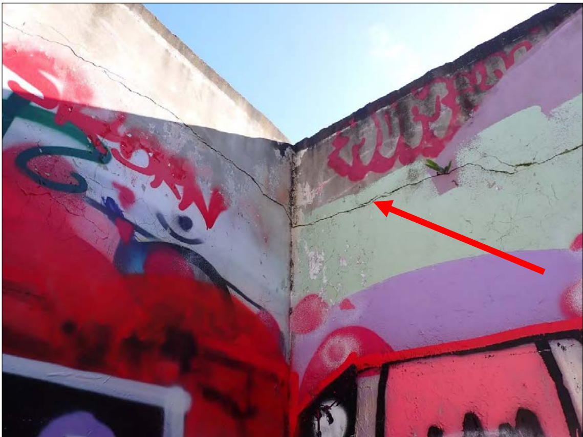
Figure 182. Feature 14: Magazine 11. Interior – Typical horizontal cracking to corners is indicated.
