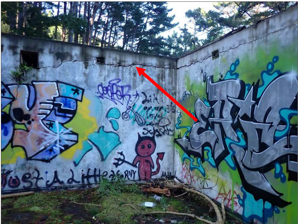
Figure 147. Feature 9: Magazine 9. Interior – Typical horizontal cracking to corners is indicated. Graffiti is present.
