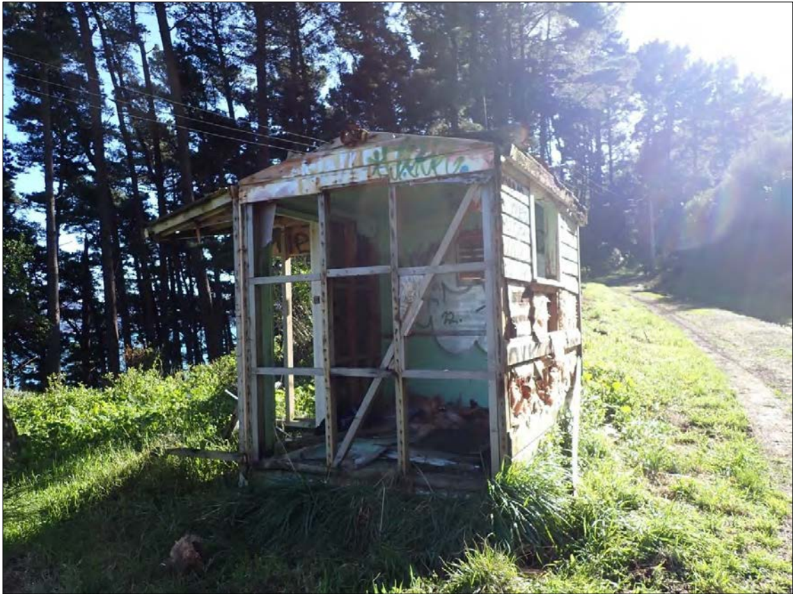
Figure 160. Feature 11: Hut (former use unknown). Looking towards the northern elevation. The weatherboards have come away and the remains of a small entrance porch is visible to the RHS.
