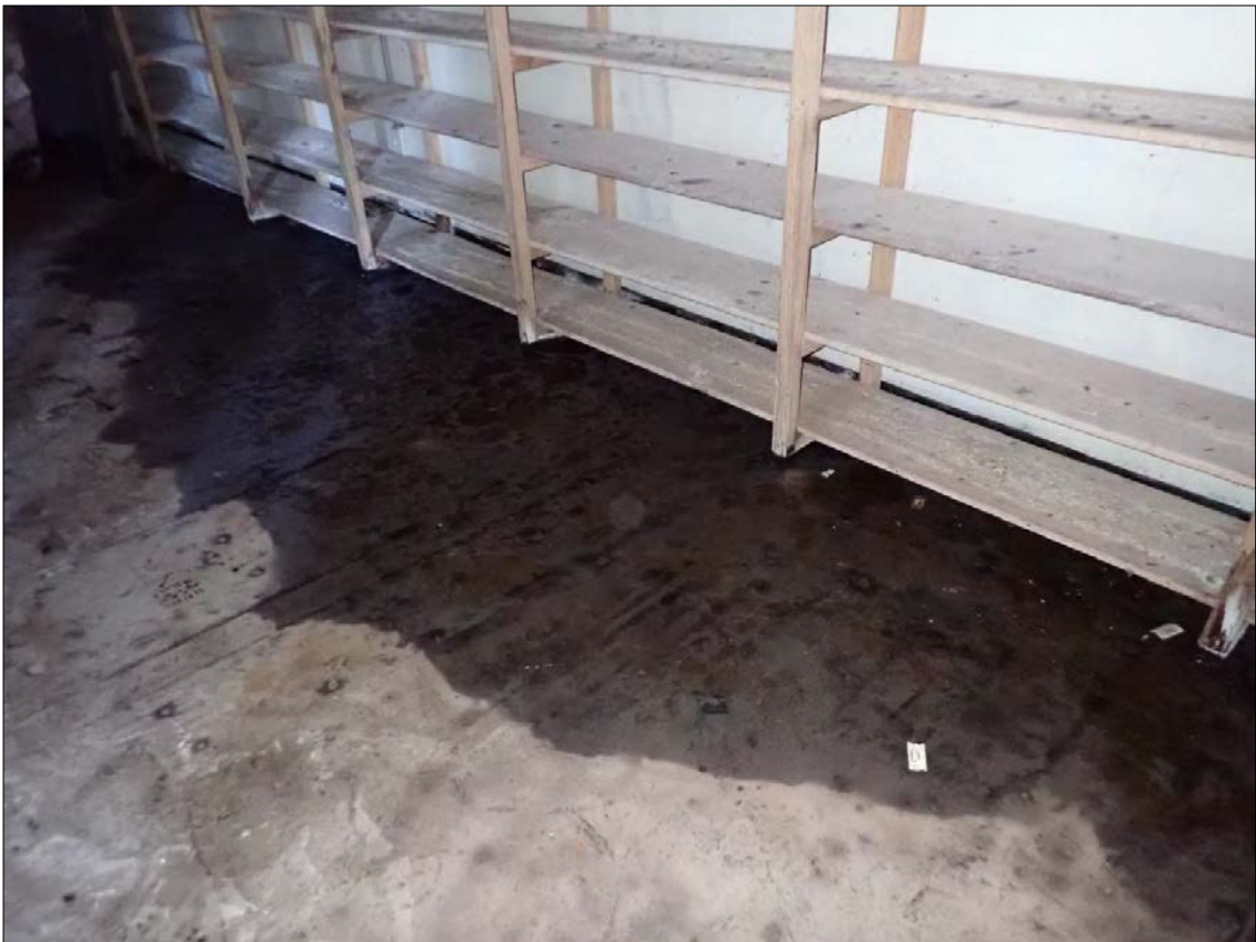
Figure 138. Feature 8: Magazine 8 Interior – Water is entering the structure.
