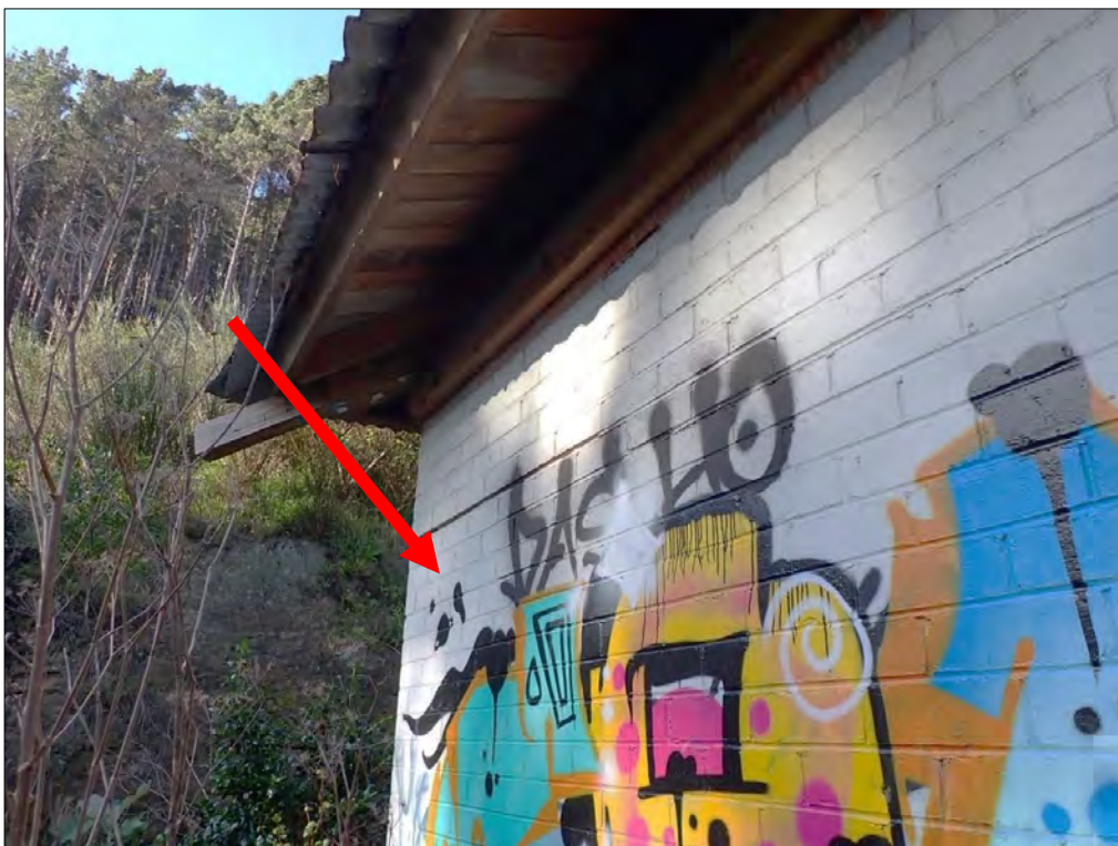
Figure 103. Feature 4: Magazine 4. Looking along the northern (front) elevation. Typical horizontal crack is indicated at the corner. Boarding to the closed eaves has come away and rainwater goods are missing.
