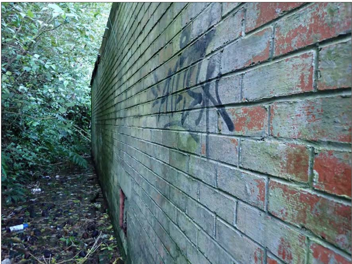
Figure 143. Feature 9: Magazine 9 Looking along the northern (side) elevation. Graffiti is present and water is ponding against the side of the structure.
