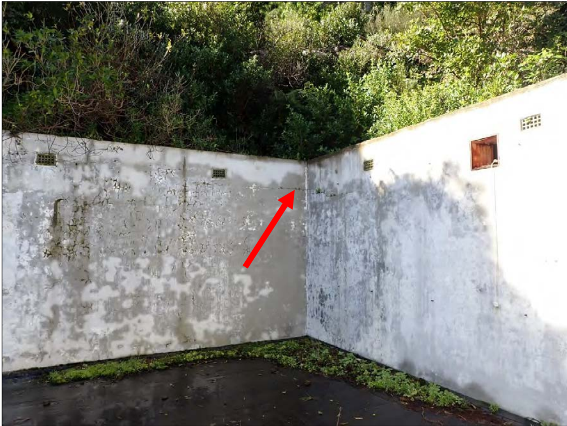
Figure 86. Feature 1: Magazine 1. Interior - Horizontal cracking is indicated at the rear northeastern corner.
