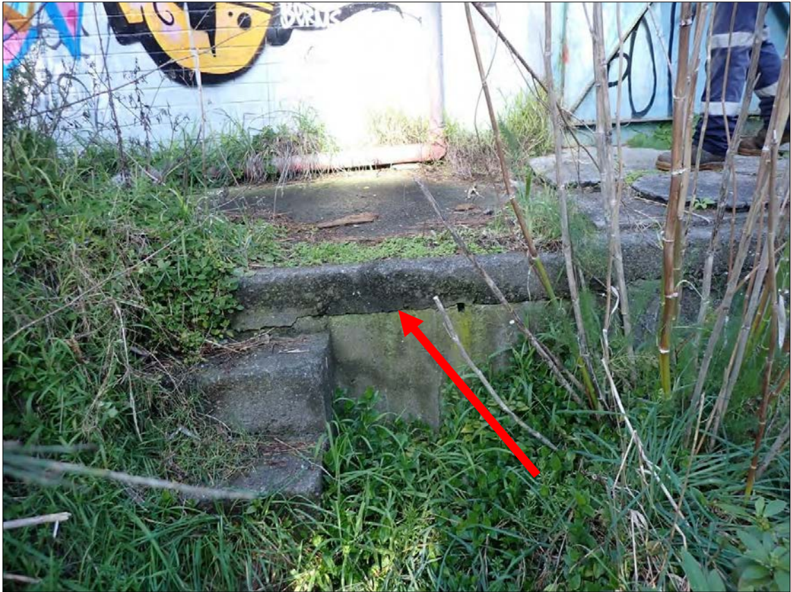
Figure 104. Feature 4: Magazine 4. Looking towards the northern (front) elevation. Horizontal cracking beneath the loading deck concrete slab is indicated.
