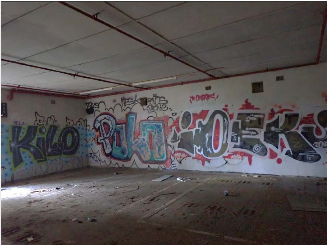
Figure 107. Feature 4: Magazine 4. Interior – Ceiling is present and fluorescent lights and sprinkler system remain. Graffiti is present. Water penetration is not evident.
