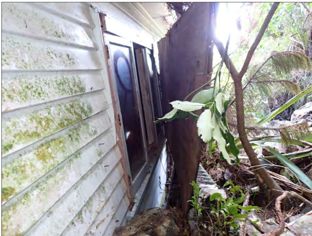
Figure 163. Feature 12: Former sergeant's house. Looking along the northern (side) elevation. Window boarding has been partially removed and access to the house is possible. Debris, the result of a slip, has accumulated against the house.
