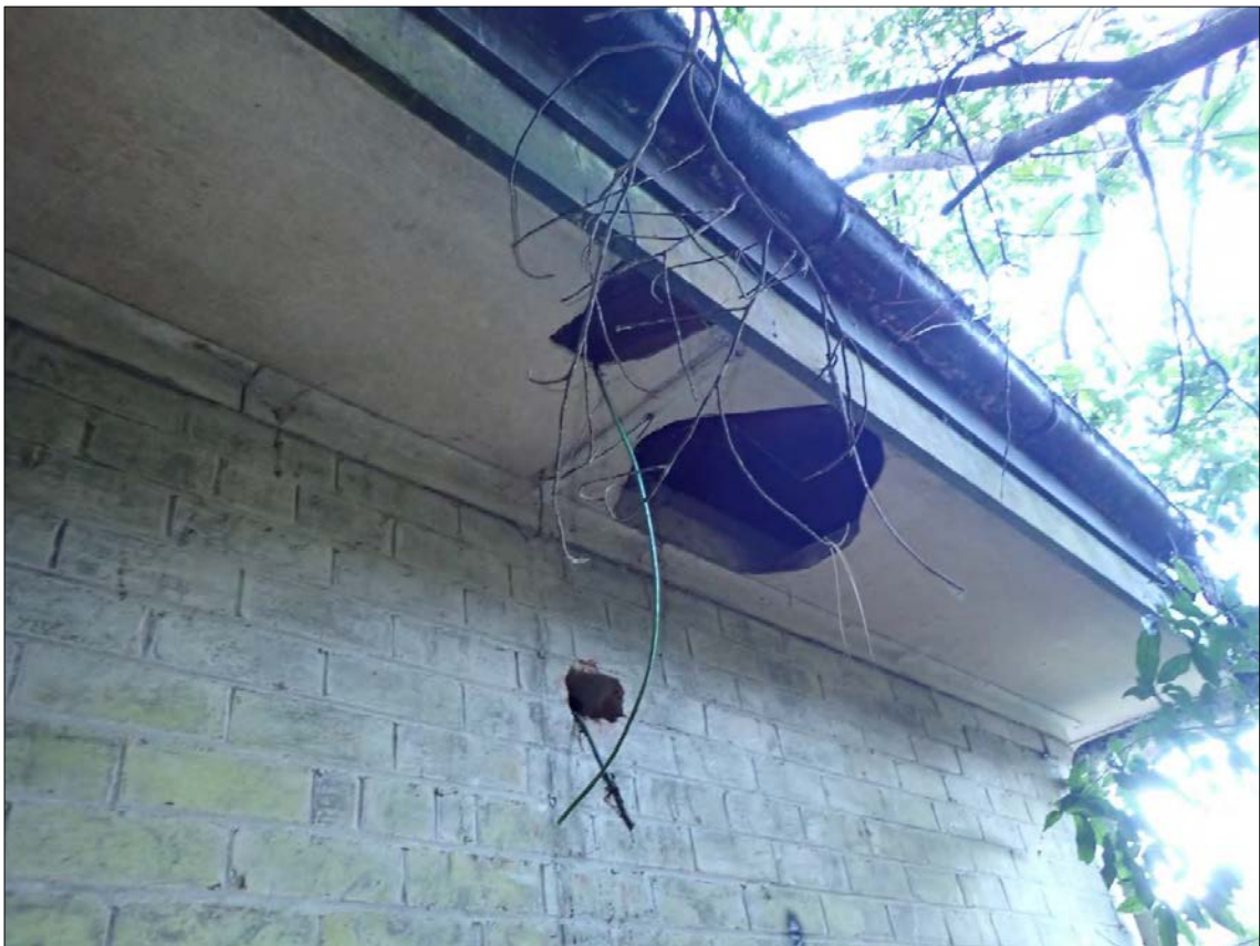
Figure 151. Feature 10: Magazine 10. Northern (side) elevation. Underside eaves is damaged.
