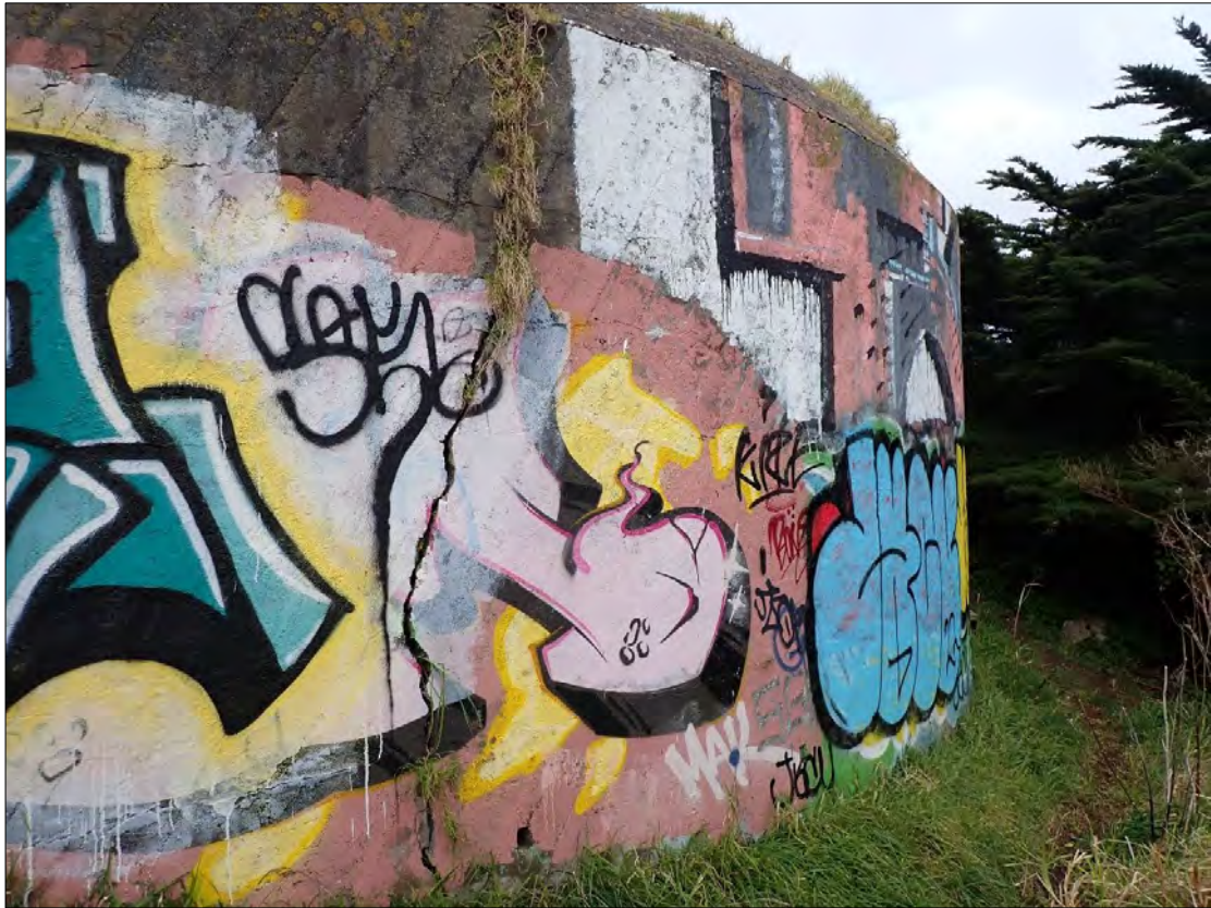
Figure 260. Feature 27: Fort Ballance. Example of cracking to walls.
