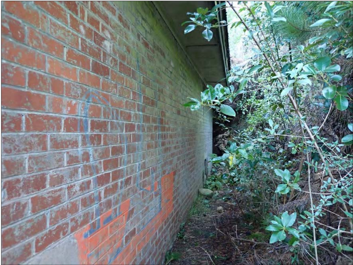
Figure 152. Feature 10: Magazine 10. Looking along the southern (side) elevation. Graffiti is present and a slip has occurred to the rear.
