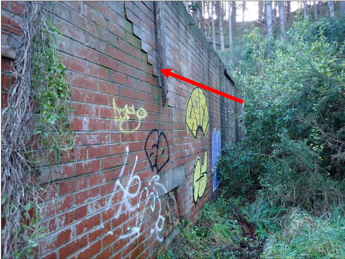
Figure 144. Feature 9: Magazine 9. Looking along the southern (side) elevation. Graffiti is present. Diagonal crack associated with horizontal cracking is indicated. Vegetation and debris have accumulated against the side of the structure.
