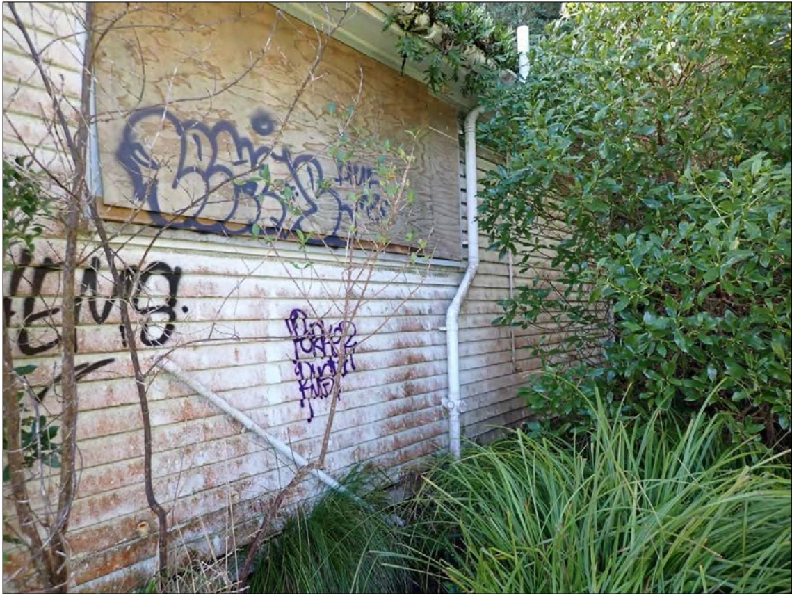
Figure 164. Feature 12: Former sergeant's house. Looking along the southern (side) elevation. Graffiti is present and openings have been boarded up. Vegetation is encroaching onto the house and there is vegetation in the gutters.
