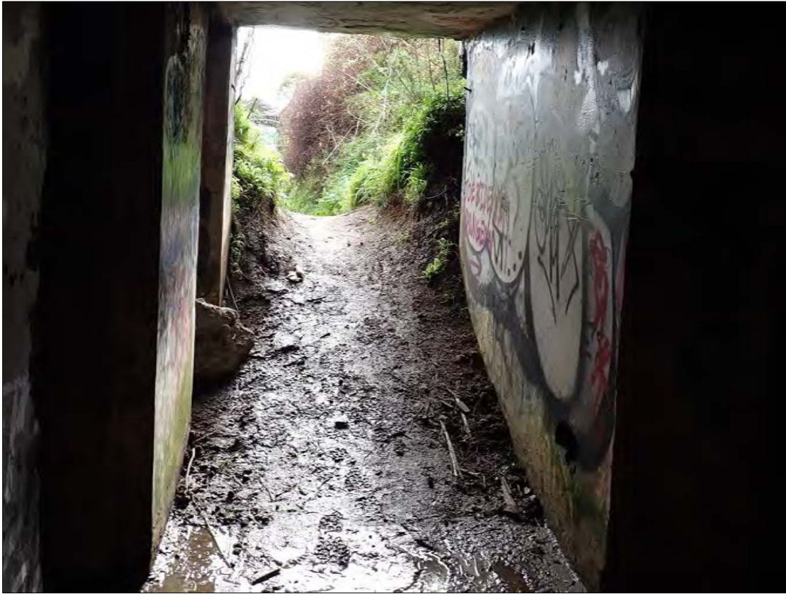
Figure 256. Feature 27: Fort Ballance. Earth build-up at tunnel entrance to the disappearing gun at 6inch BLHP (Pit A). Image cropped.
