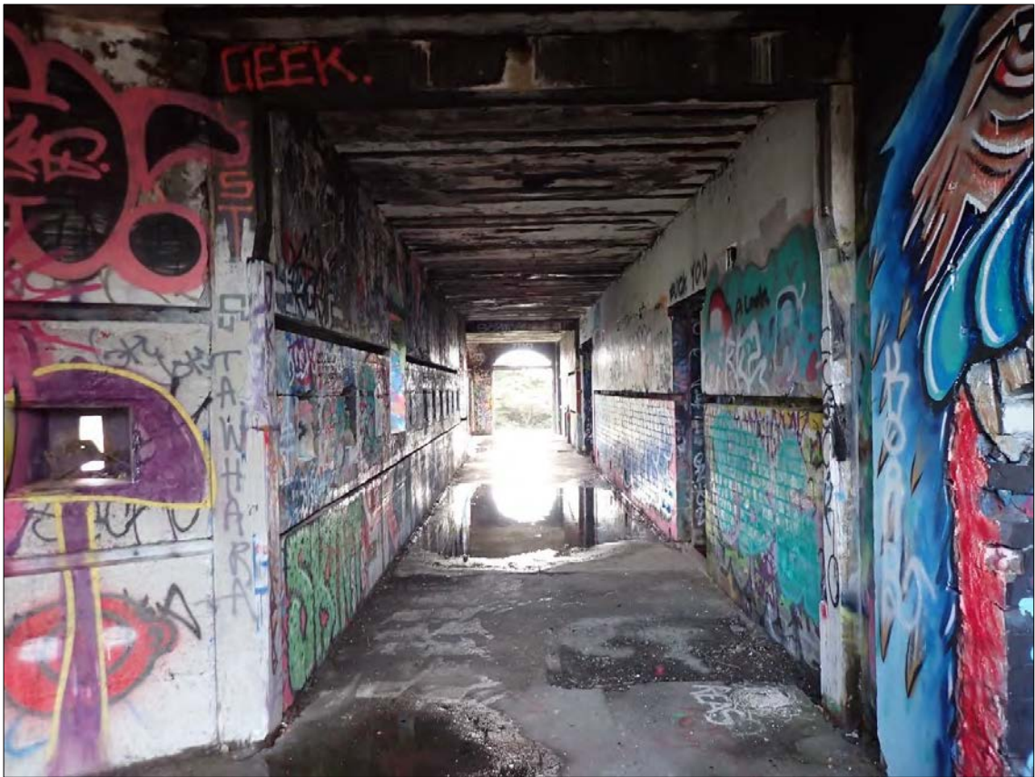
Figure 242. Feature 27: Fort Ballance. Artillery barracks. Water is ponding internally, and graffiti is present.
