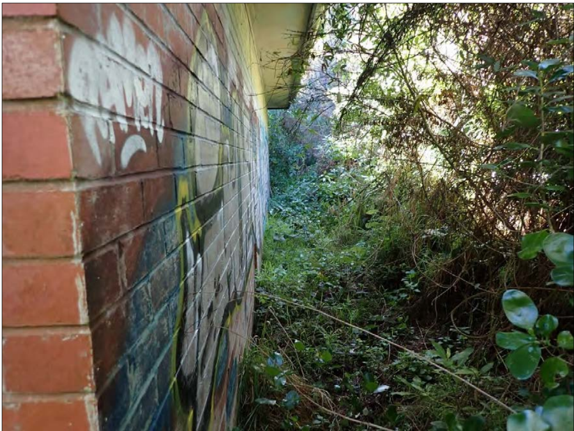
Figure 99. Feature 3: Magazine 3. Looking along the eastern (rear) elevation. Debris and vegetation have accumulated against the structure. Graffiti is present.
