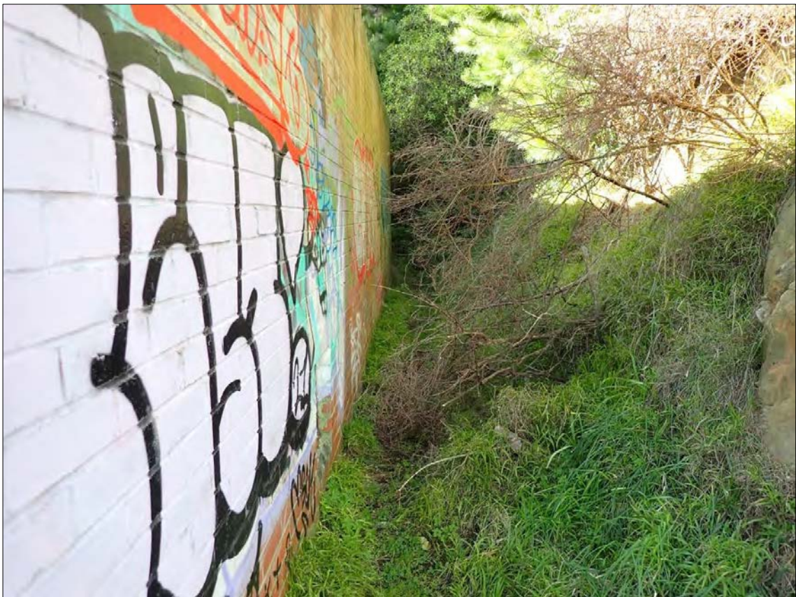
Figure 174. Feature 14: Magazine 11. Looking along the southern (side) elevation. Vegetation is accumulating against the side of the structure.
