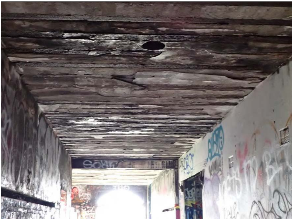
Figure 245. Feature 27: Fort Ballance. Artillery barracks. Underside roof steel reinforcement is rusting.
