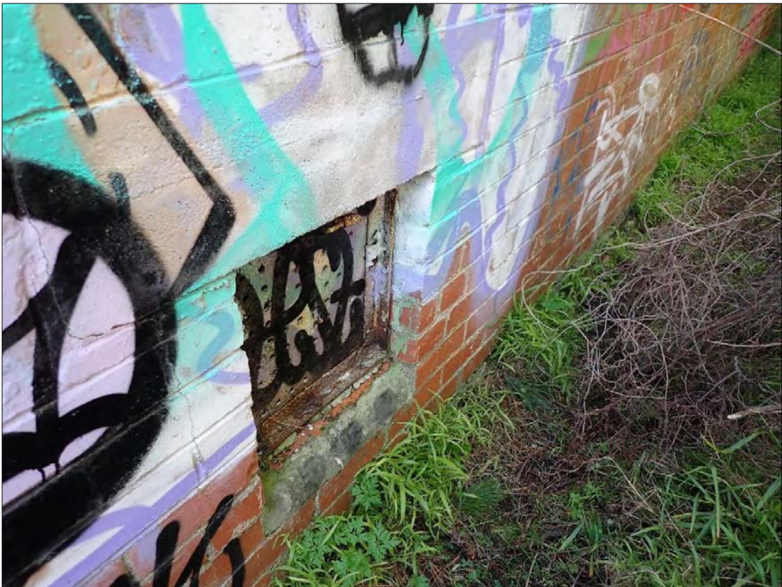
Figure 176. Feature 14: Magazine 11. Example of vermin proofing to vent between inner and outer wall of structure.
