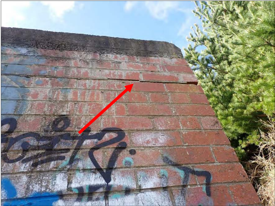
Figure 173. Feature 14: Magazine 11. Typical horizontal crack is evident at the corner of the western (front) elevation.
