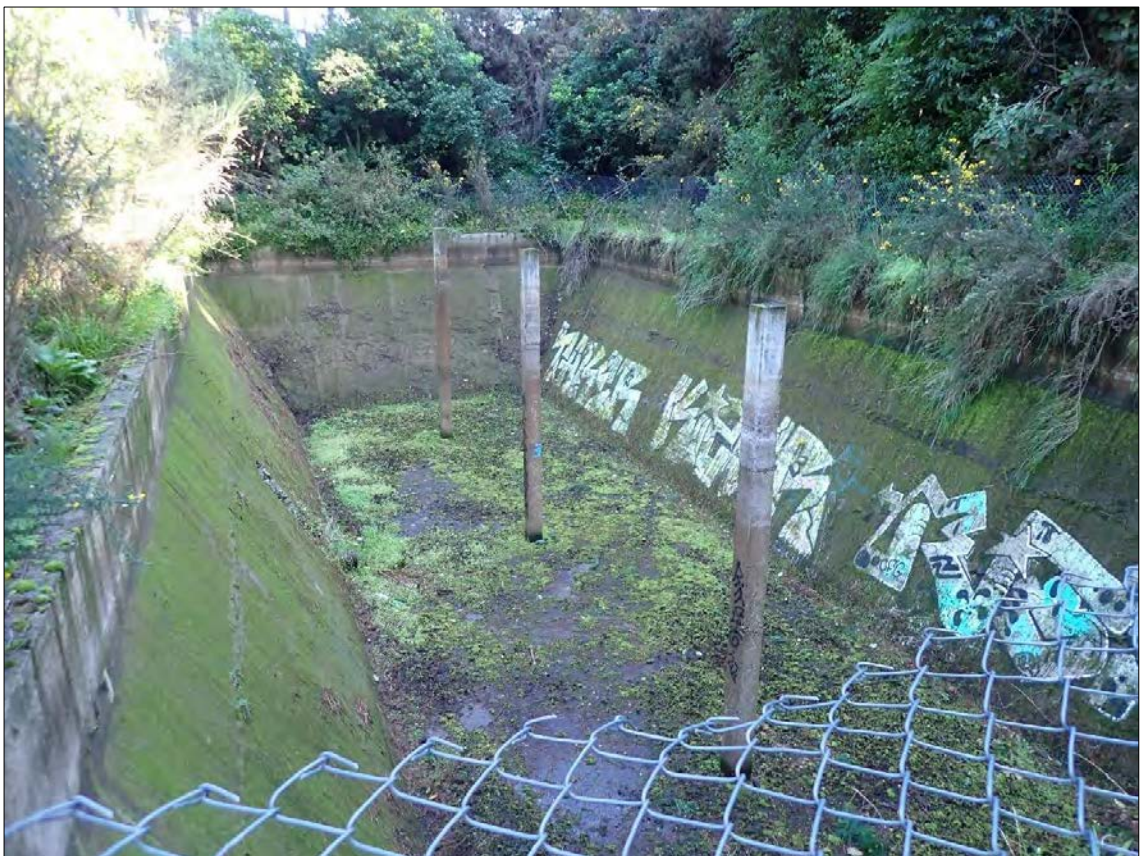
Figure 67: The reservoir used for holding water in case of the armaments within the magazines exploding (NZHP, 2022).
