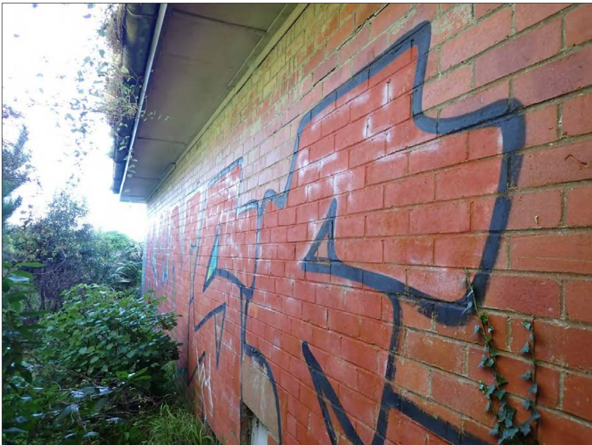
Figure 97. Feature 3: Magazine 3. Looking along the southern (side) elevation. Vegetation is present against the side of the structure; ivy is growing up the wall and graffiti is present.
