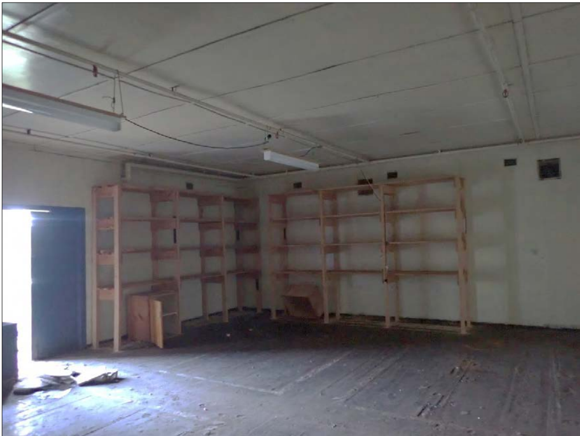
Figure 101. Feature 3: Magazine 3. Interior – Fluorescent lights are suspended from the sprinkler system. Water penetration is not evident. Some material goods associated with the most recent use remain within the structure.
