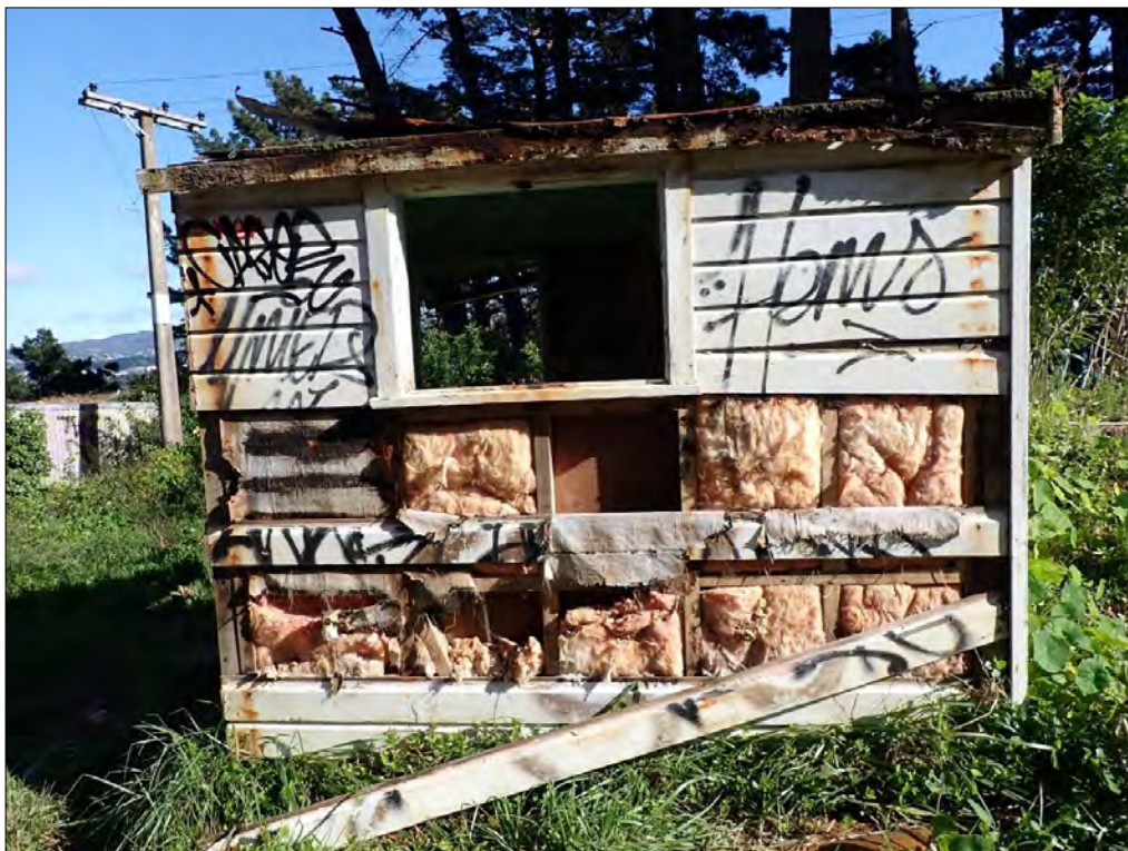
Figure 159. Feature 11: Hut (former use unknown). Looking towards the western elevation. Graffiti is present, weatherboards are coming away, window and rainwater goods are no longer in position.
