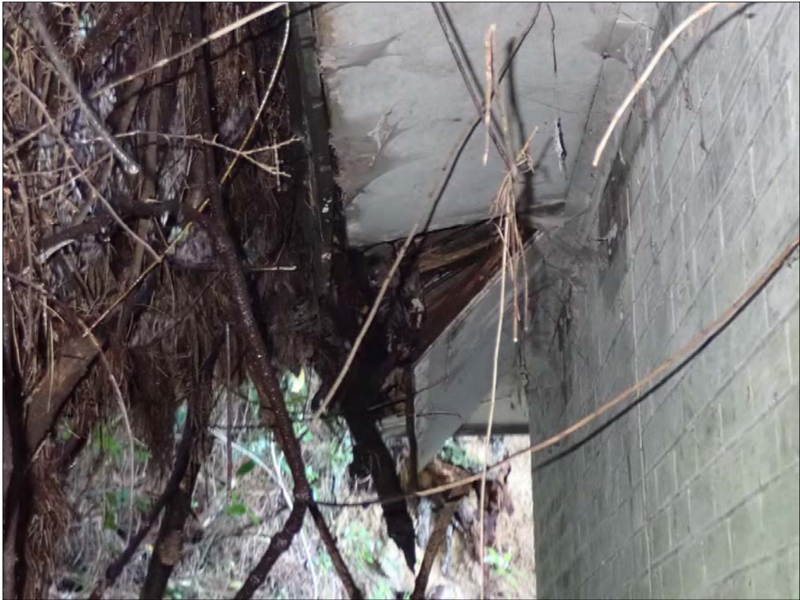
Figure 154. Feature 10: Magazine 10. Looking along the eastern (rear) elevation. The underside eaves is damaged.
