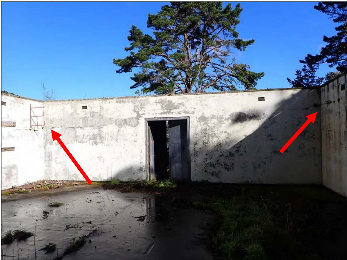
Figure 85. Feature 1: Magazine 1. Interior - Looking towards the entrance. Horizontal cracking is indicated at the corners.
