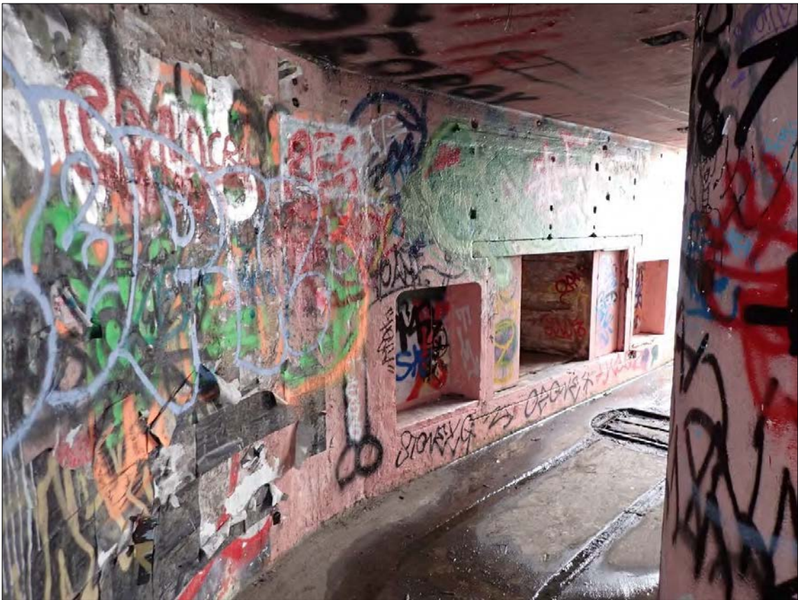
Figure 257. Feature 27: Fort Ballance. Trolley tracks at tunnel to the disappearing gun at 6inch BLHP.
