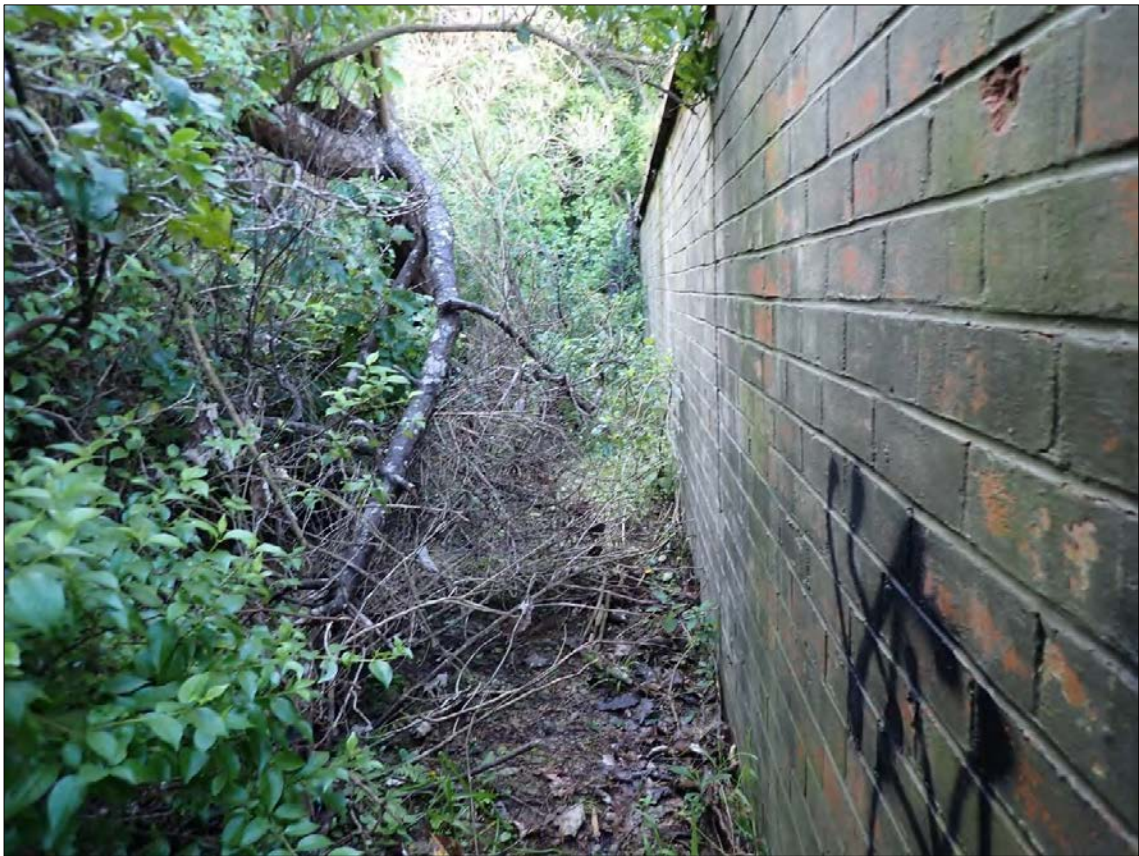
Figure 84. Feature 1: Magazine 1. Looking along the northern (side) elevation. Graffiti is present. A slip has occurred to the rear, and vegetation and debris has accumulated against the side of the structure.
