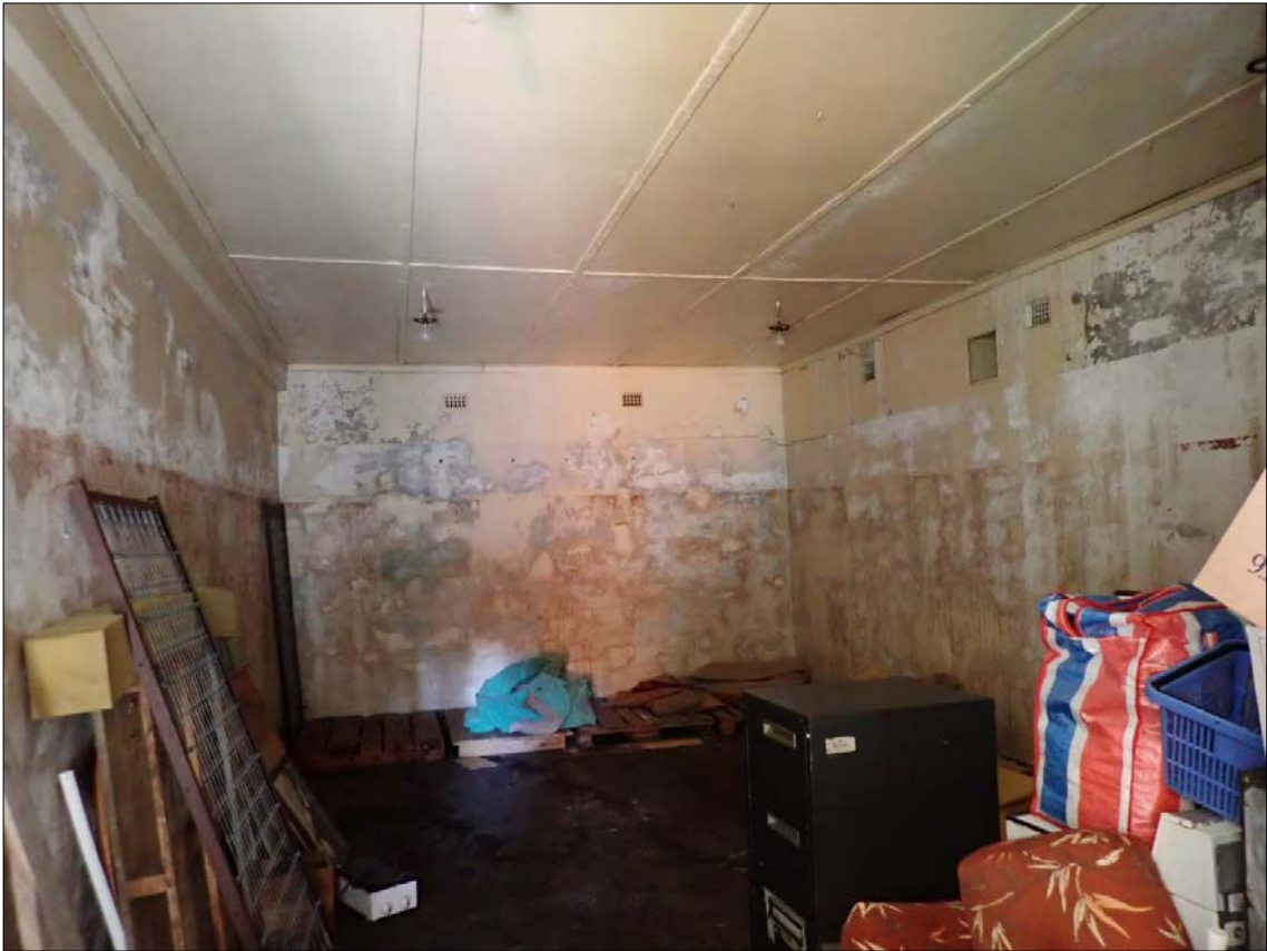
Figure 121. Feature 6: Magazine 6. Interior – Water penetration is evident. Some material goods remain within the structure.
