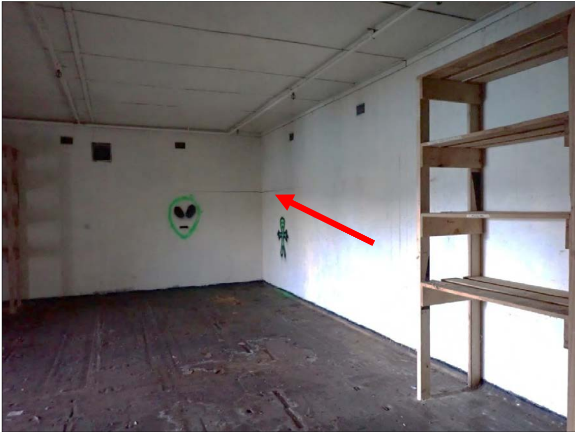
Figure 100. Feature 3: Magazine 3. Interior – Ceiling is present and fire sprinklers are evident. Graffiti is present. Typical horizontal crack at corner is indicated.
