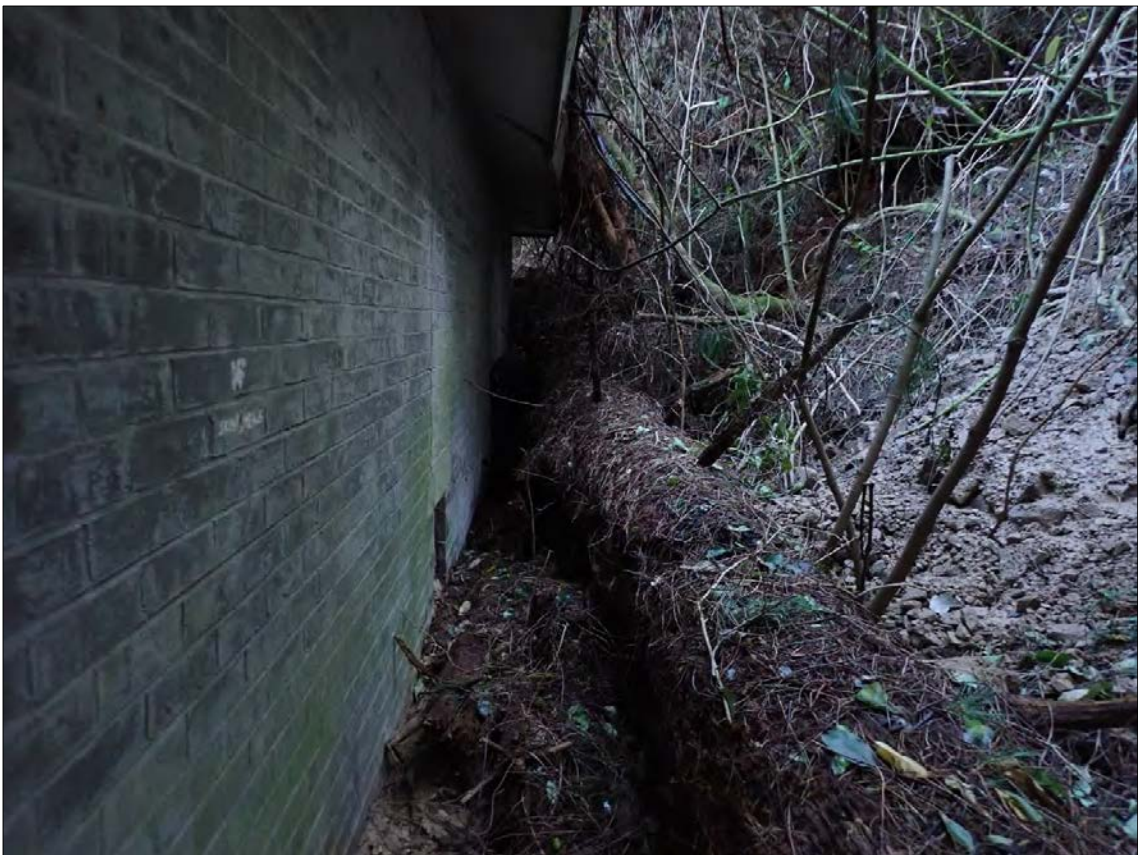
Figure 134. Feature 8: Magazine 8. Looking along the eastern (rear) elevation. A slip has occurred, and vegetation and debris are accumulating against the side of the structure.
