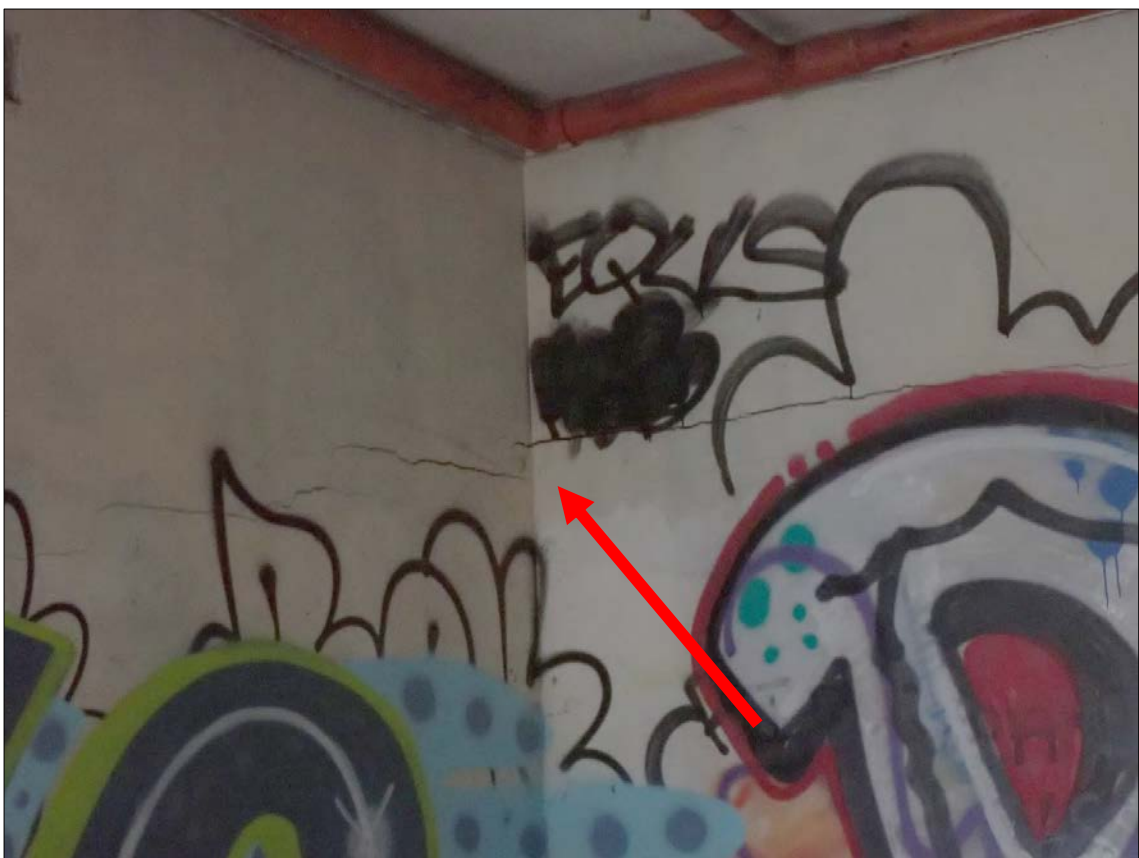
Figure 109. Feature 4: Magazine 4. Interior – Typical horizontal corner crack indicated.
