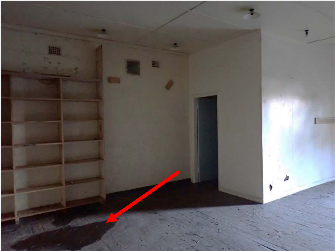
Figure 157. Feature 10: Magazine 10. Interior – Water is entering the structure.
