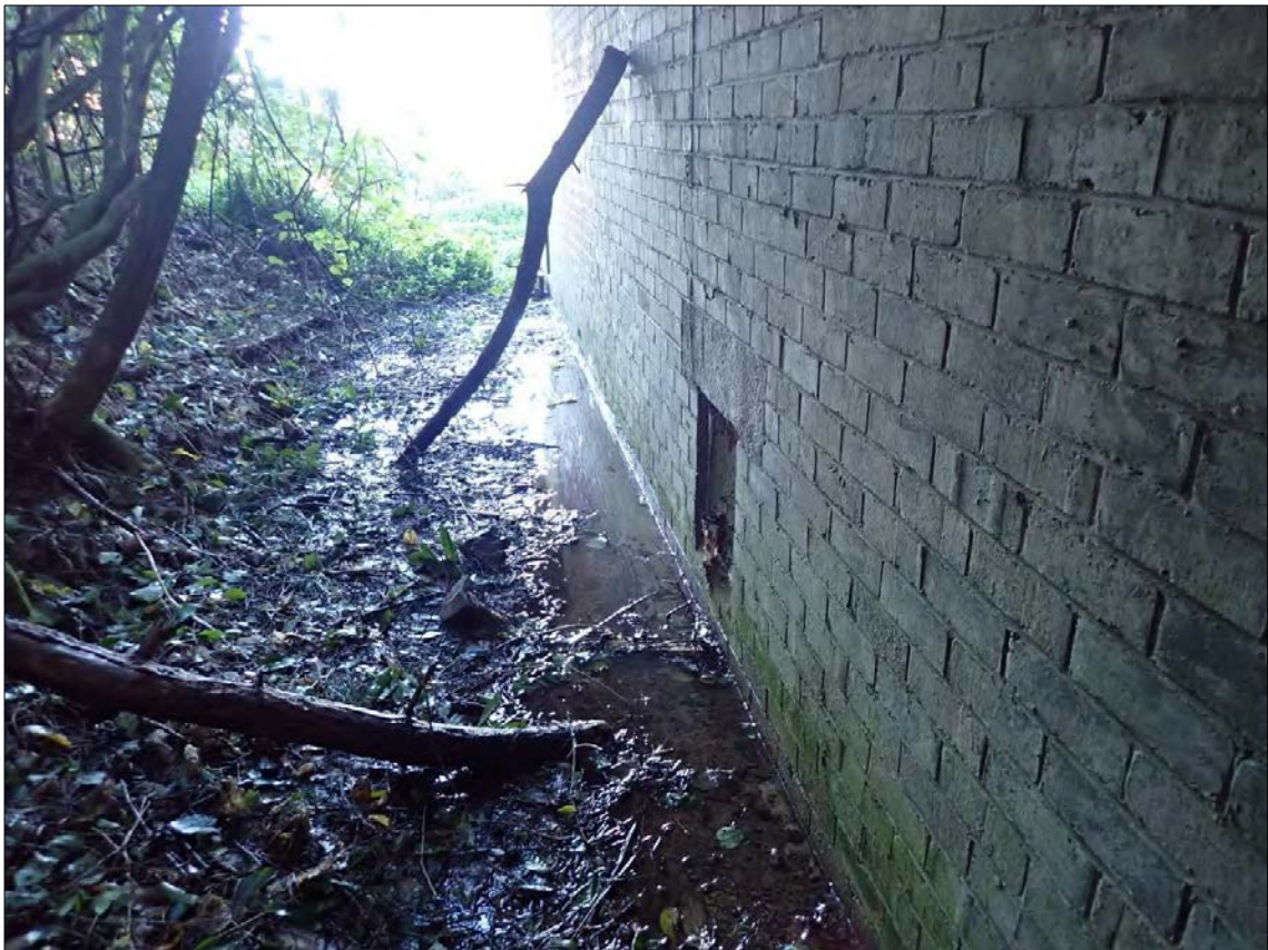
Figure 135. Feature 8: Magazine 8. Looking along the eastern (rear) elevation. Ponding is evident.
