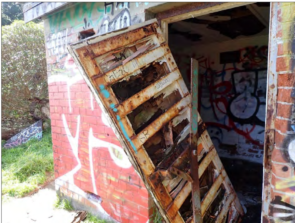
Figure 186. Feature 16: Arms store. Looking towards the western elevation. The entrance door has come off its hinges.
