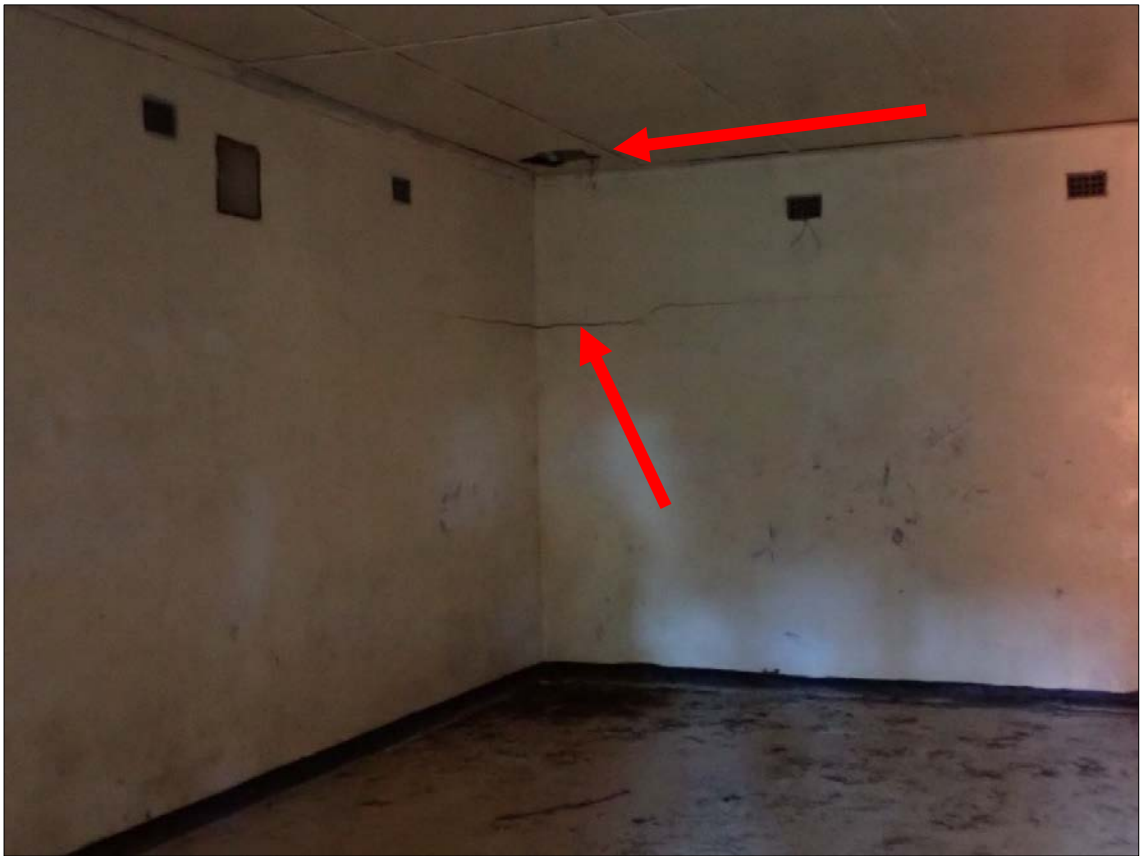
Figure 127. Feature 7: Magazine 7. Interior – typical horizontal corner crack indicated. Ceiling is failing in places.
