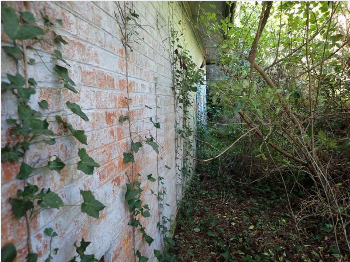
Figure 89. Feature 2: Magazine 2. Looking along the southern (side) elevation. Ivy is growing up the wall, and vegetation and debris has accumulated against the side of the structure.
