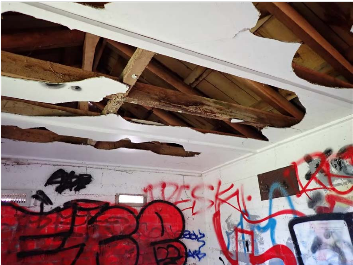
Figure 190. Feature 16: Arms store. Interior – Ceiling has been damaged. Graffiti is present.
