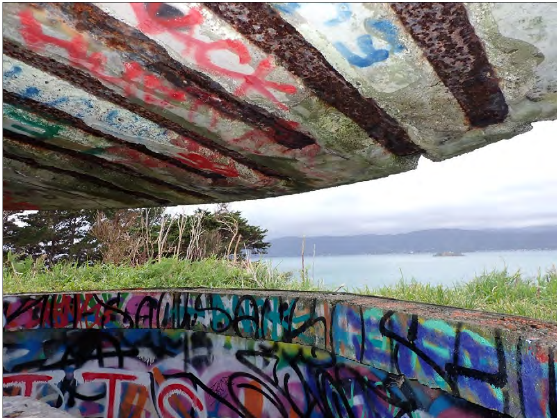
Figure 253. Feature 27: Fort Ballance. Pit B lookout. Underside slab reinforcement corroding and spalling of concrete, and extensive graffiti.
