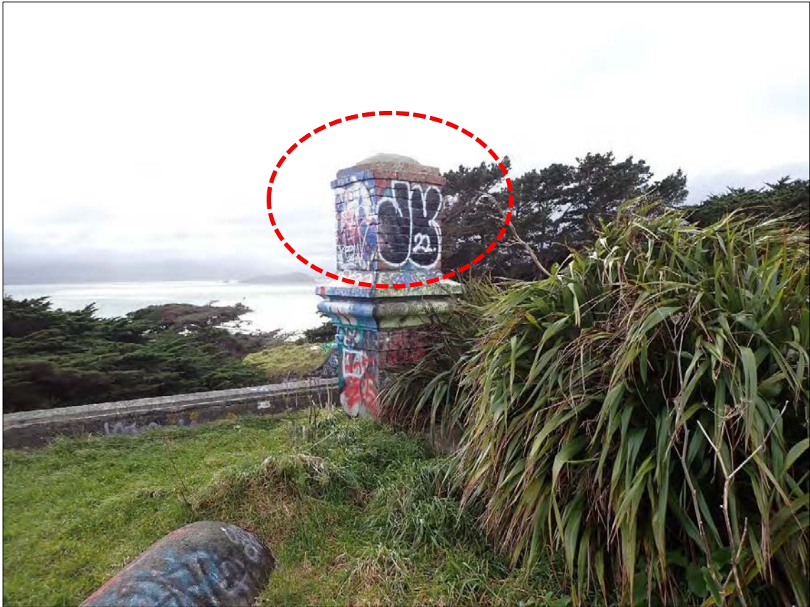
Figure 250. Feature 27: Fort Ballance. Artillery barracks roof. Original chimney has been increased in height.
