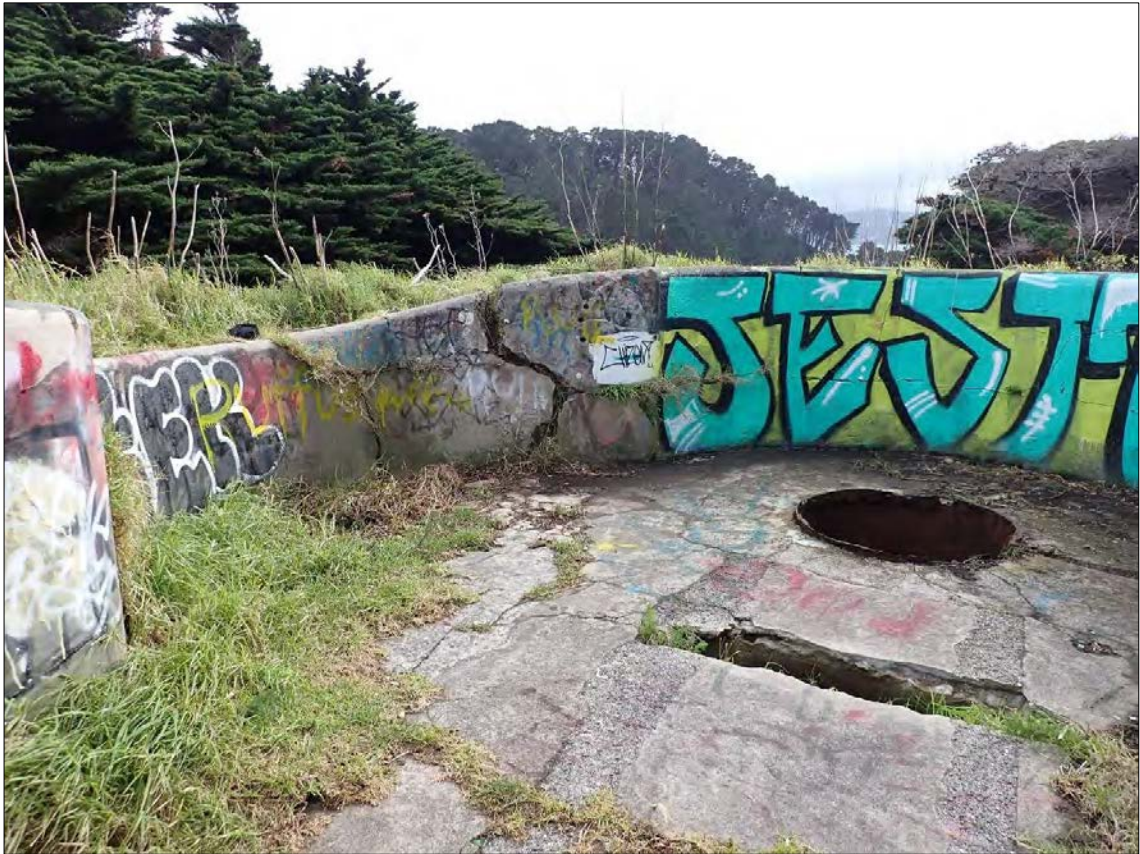
Figure 258. Feature 27: Fort Ballance. Extensive cracking at the 6QR PF.
