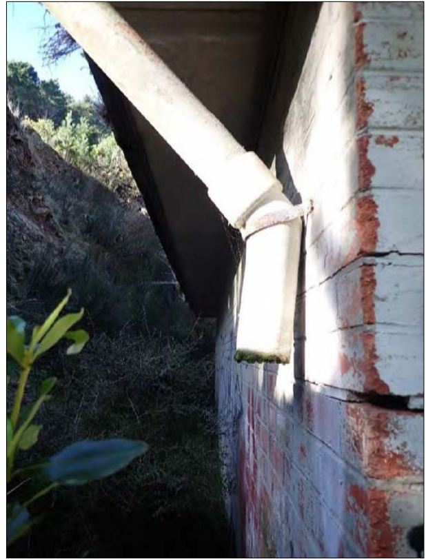
Figure 117. Feature 6: Magazine 6. Looking along the northwestern (side) elevation. Graffiti is present. Vegetation and debris are present against the side of the structure (LHS image). A rainwater downpipe is broken (RHS image).
