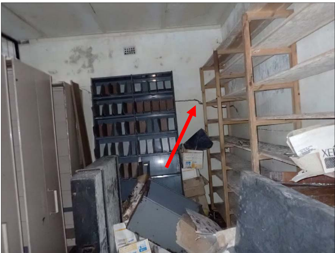
Figure 136. Feature 8: Magazine 8 Interior – Substantial horizontal corner crack indicated. Some material goods associated with the most recent use remain within the structure.
