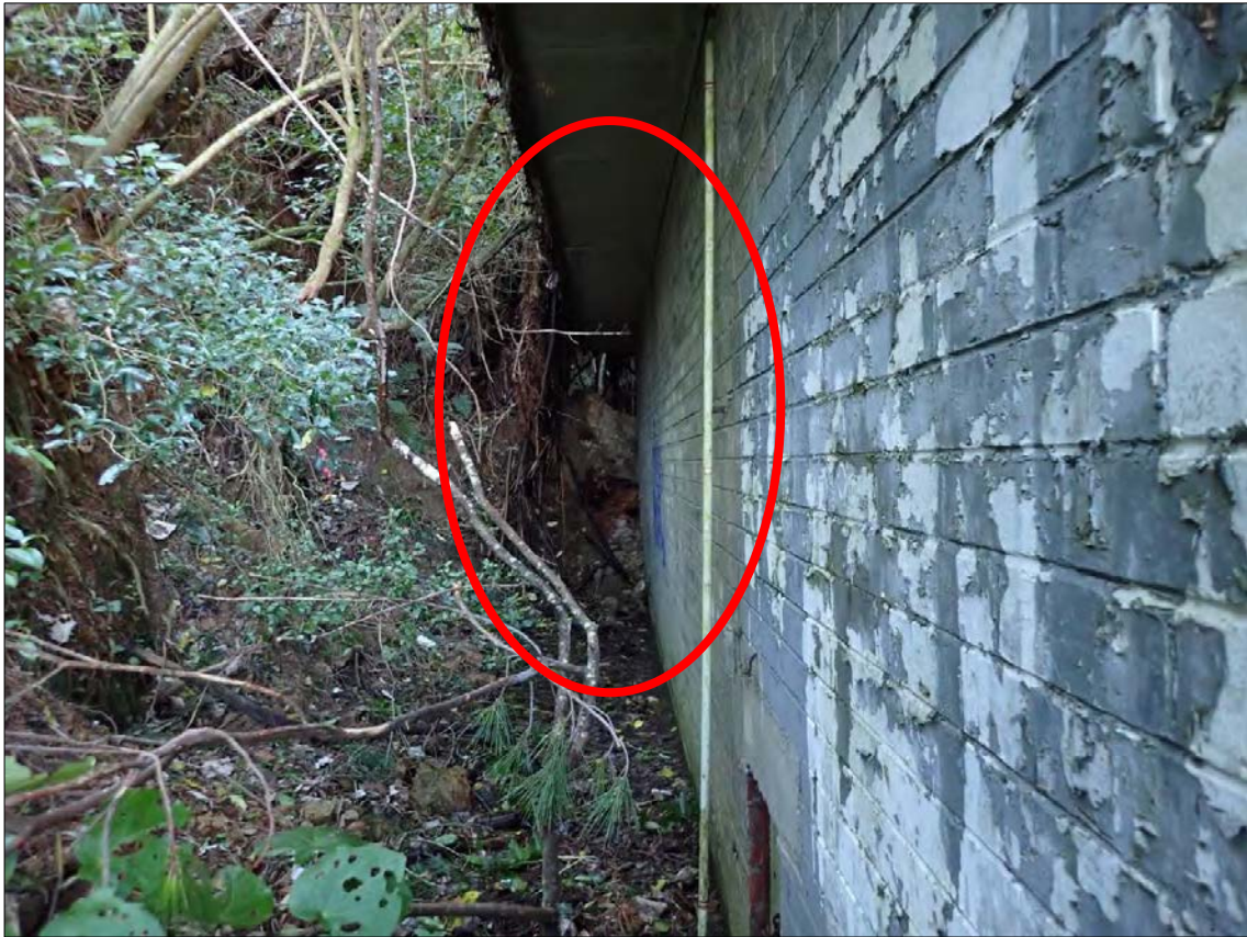
Figure 131. Feature 8: Magazine 8. Looking along the northern (side) elevation. Graffiti is present, and vegetation and debris are accumulating against the side of the structure. A slip is visible towards the rear.
