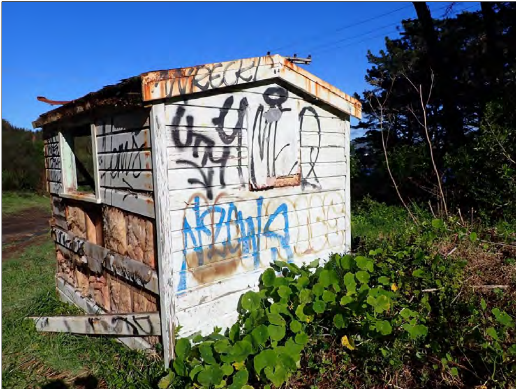
Figure 158. Feature 11: Hut (former use unknown). Looking southwest. Graffiti is present, weatherboards are coming away and rainwater goods are no longer in position.
