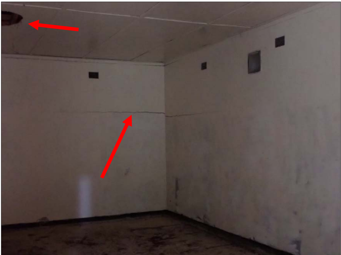
Figure 128. Feature 7: Magazine 7. Interior – typical horizontal corner crack indicated. Ceiling is failing in places.
