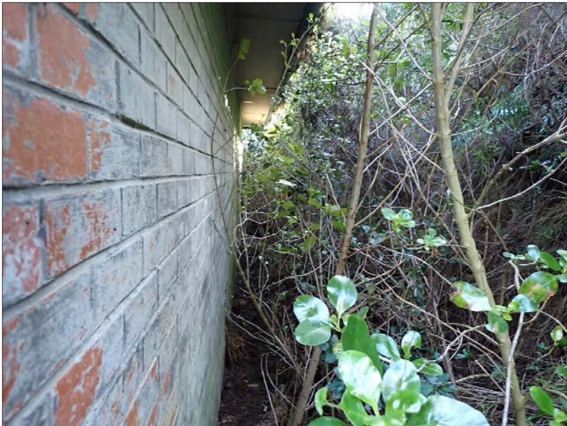
Figure 91. Feature 2: Magazine 2. Looking along the eastern (rear) elevation. A slip has occurred to the rear, and vegetation and debris has accumulated against the side of the structure.
