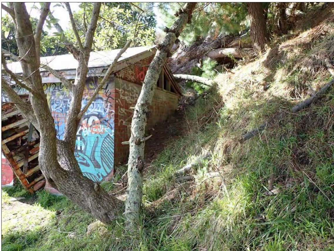
Figure 188. Feature 16: Arms store. Looking at the southern elevation. A slip has occurred, and vegetation and debris are accumulating against the side of the structure.
