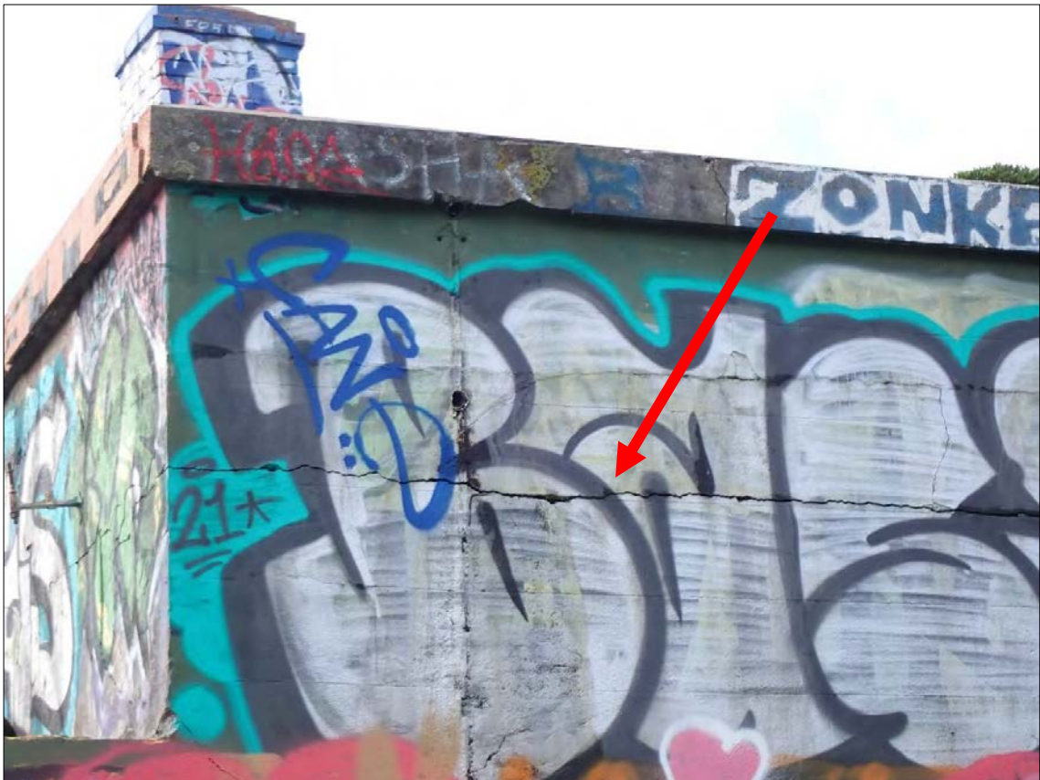
Figure 239: Feature 27: Fort Ballance. Artillery barracks. Typical example of horizontal cracking.
