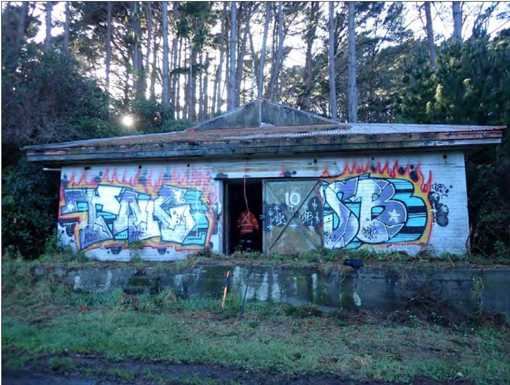
Figure 148. Feature 10: Magazine 10. Looking towards the western (front) elevation. Graffiti is present. The gutters are missing, and the narrow loading deck is being 'colonised' by vegetation.
