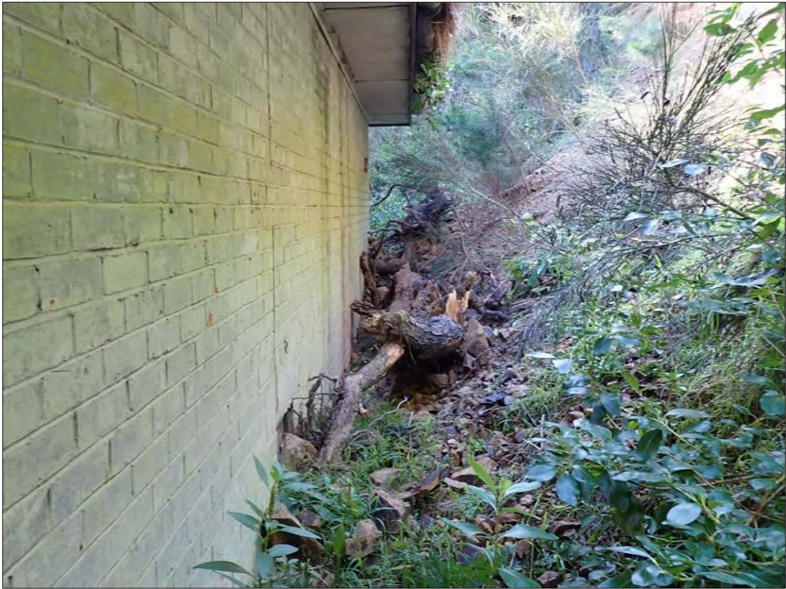
Figure 119. Feature 6: Magazine 6. Looking along the southeastern (rear) elevation – image cropped. A slip has occurred, and debris has accumulated against the structure.
