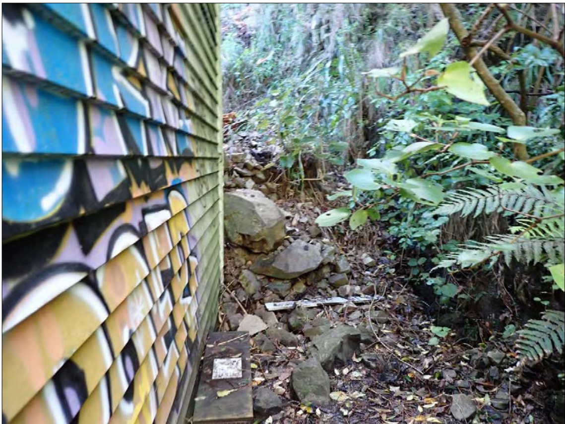
Figure 165. Feature 12: Former sergeant's house. Looking along the eastern (rear) elevation. A slip has occurred, and debris and vegetation have accumulated against the structure. Graffiti is present.
