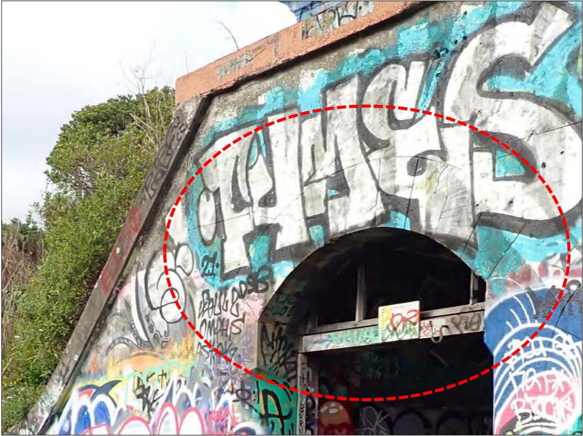
Figure 246. Feature 27: Fort Ballance. Artillery barracks. Graffiti obscures original scored concrete detailing to engine room. Image cropped.
