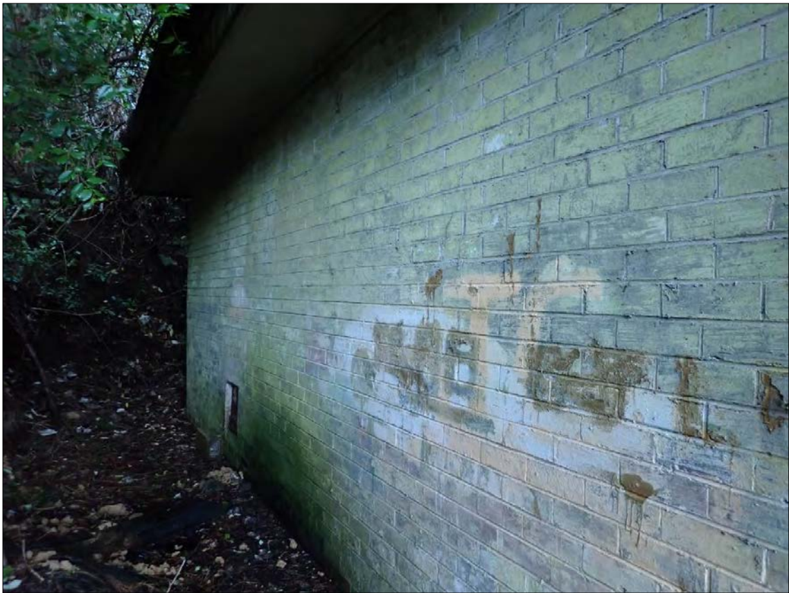
Figure 150. Feature 10: Magazine 10. Looking along the northern (side) elevation. Anti-graffiti coating is present.
