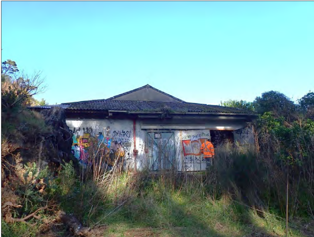
Figure 102. Feature 4: Magazine 4. Looking towards the northern (front) elevation. Graffiti is present and there is vegetation in the gutters. Some of the gutter is missing. The narrow loading deck is becoming 'colonised' by vegetation.
