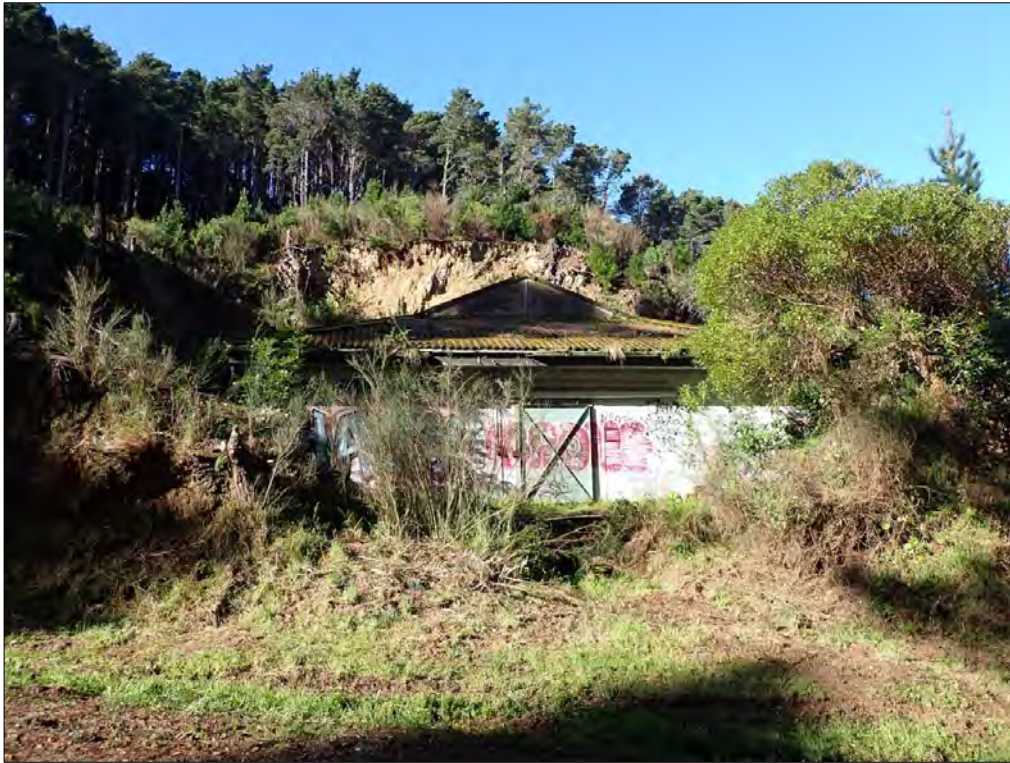
Figure 115. Feature 6: Magazine 6. Looking towards the northwestern (front) elevation. Graffiti is present and there is vegetation in the gutters
