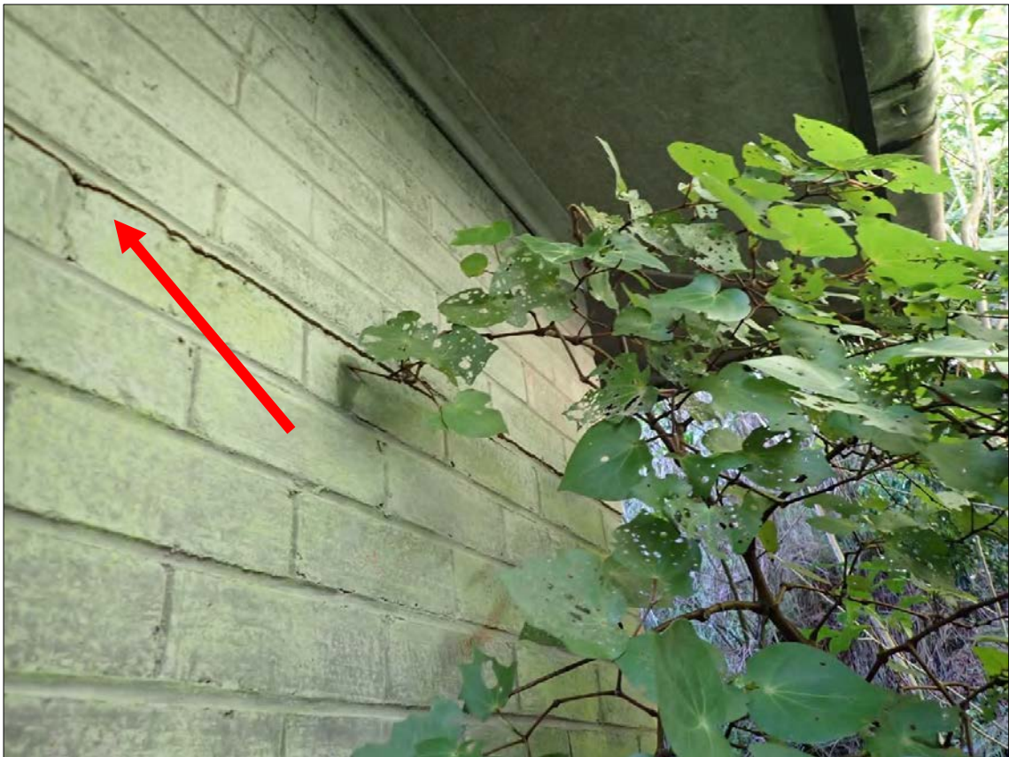
Figure 113. Feature 5: Magazine 5. Eastern (rear) elevation. Typical horizontal corner crack is indicated. Possible anti-graffiti coating.
