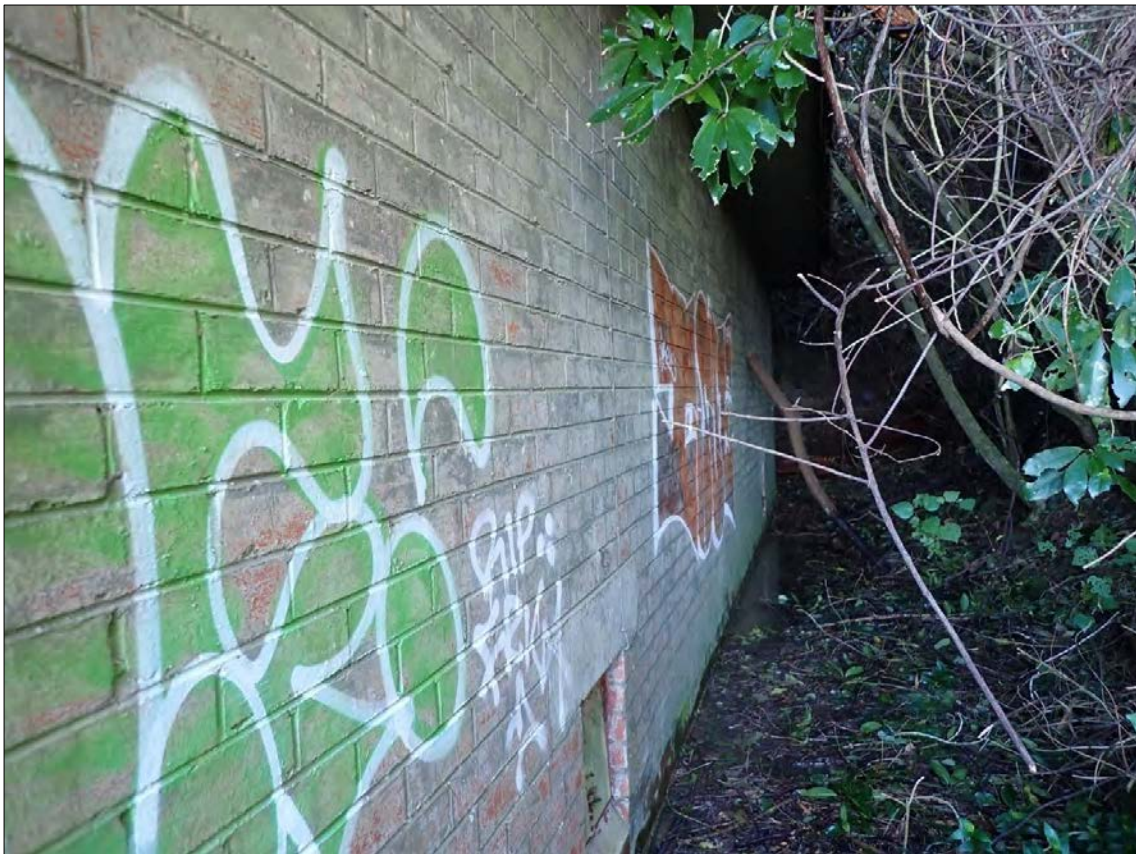
Figure 132. Feature 8: Magazine 8. Looking along the southern (side) elevation. Graffiti is present and water is ponding at the base of the structure.
