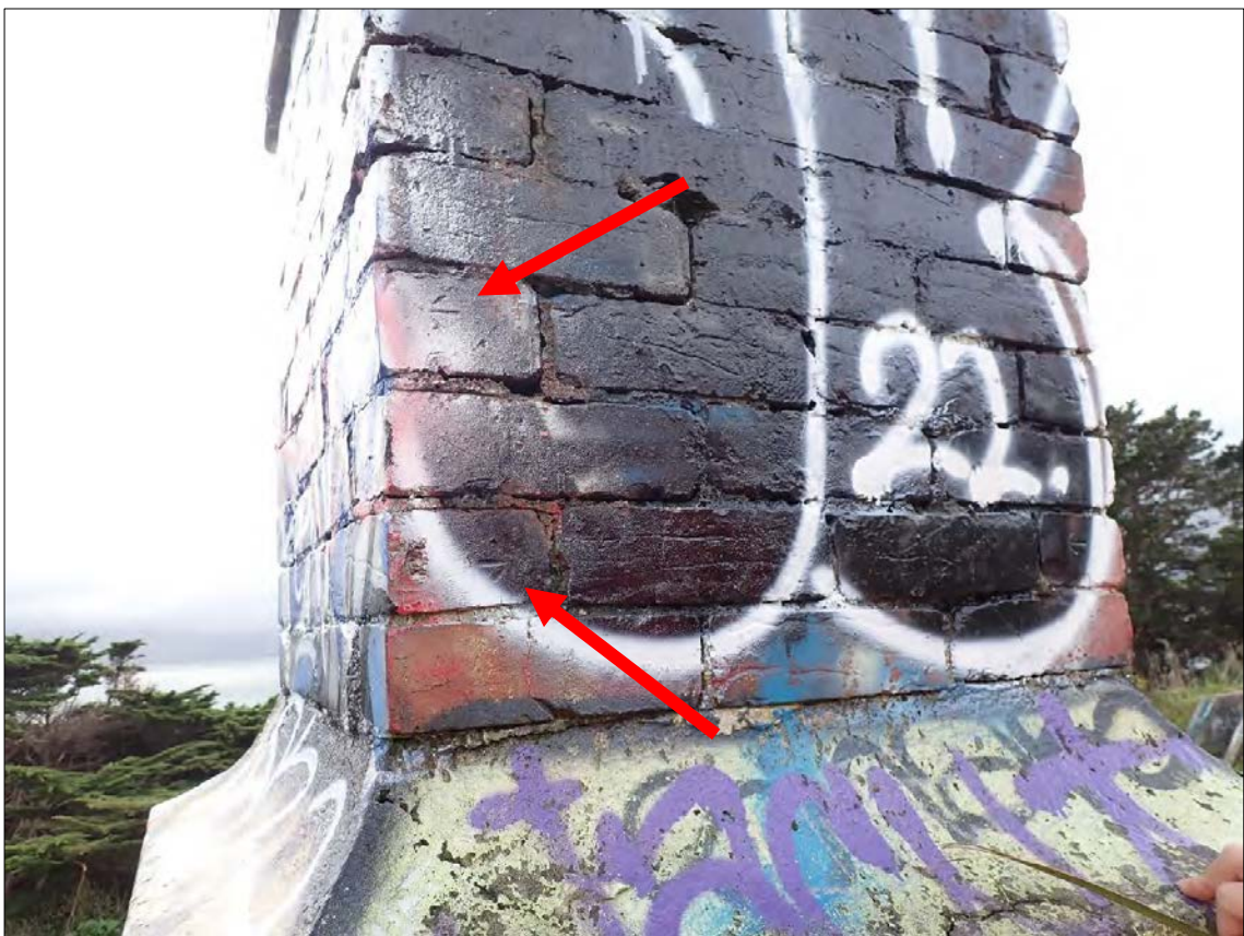
Figure 251. Feature 27: Fort Ballance. Artillery barracks roof. Original chimney increased in height using 'prison' bricks.
