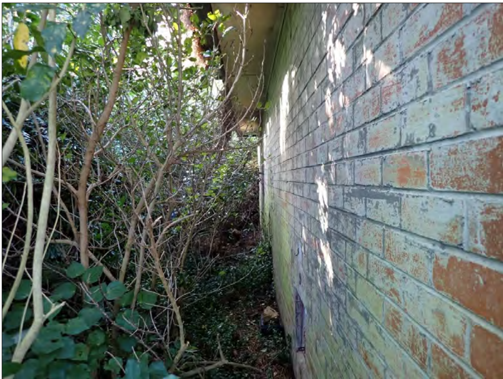
Figure 88. Feature 2: Magazine 2. Looking along the northern (side) elevation. A slip has occurred to the rear; and vegetation and debris has accumulated against the side of the structure.
