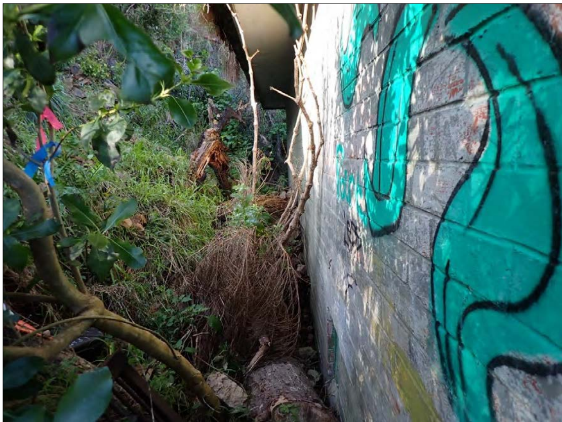
Figure 126. Feature 7: Magazine 7. Looking along the eastern (side) elevation. Vegetation and debris are accumulating against the side of the structure.
