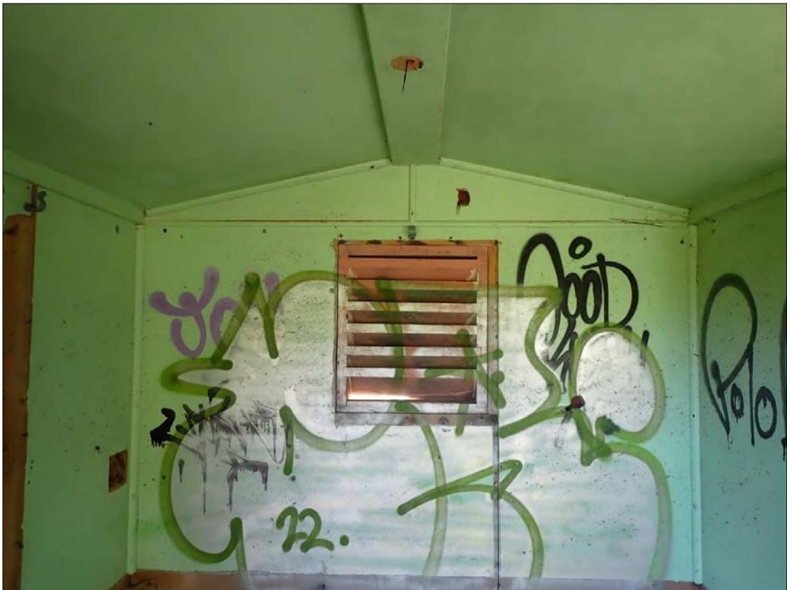
Figure 161. Feature 11: Hut (former use unknown). Interior – Timber louvre in northern elevation. Graffiti is present. Wall panelling has half round coverstrips.
