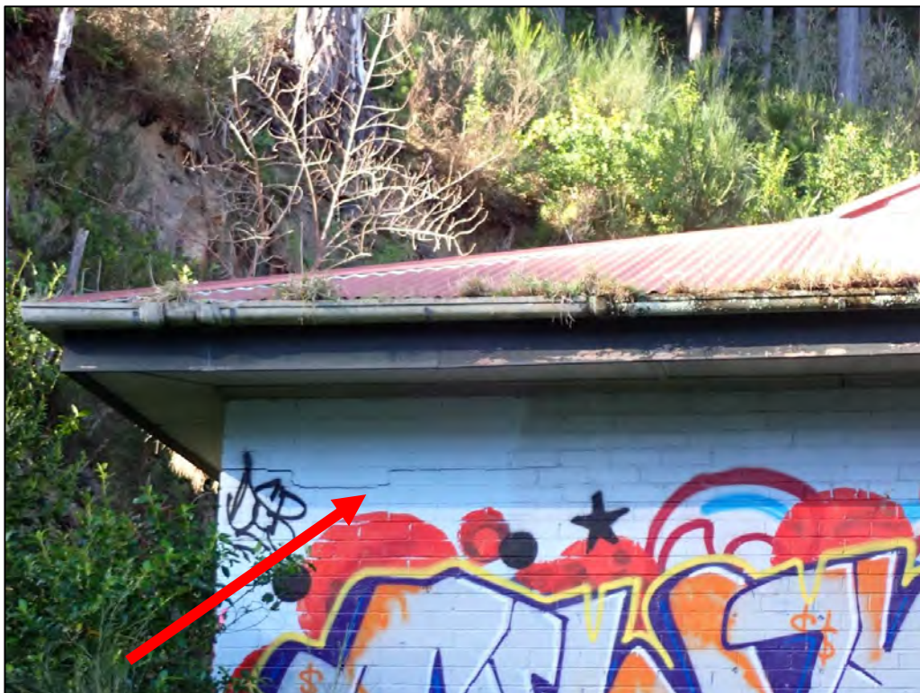
Figure 124. Feature 7: Magazine 7. Northern (front) elevation. Typical horizontal corner crack is indicated.
