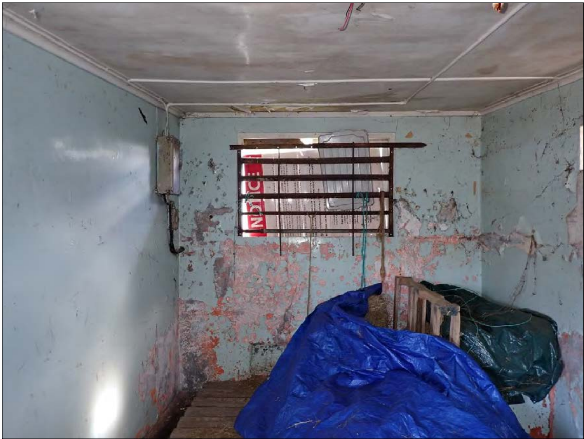
Figure 267. Feature 28: Farmstead. Milking shed interior displaying rising and falling damp, and horizontal cracking.
