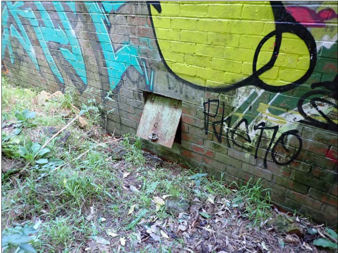
Figure 177. Feature 14: Magazine 11. Example of cover to vent between inner and outer wall of structure.
