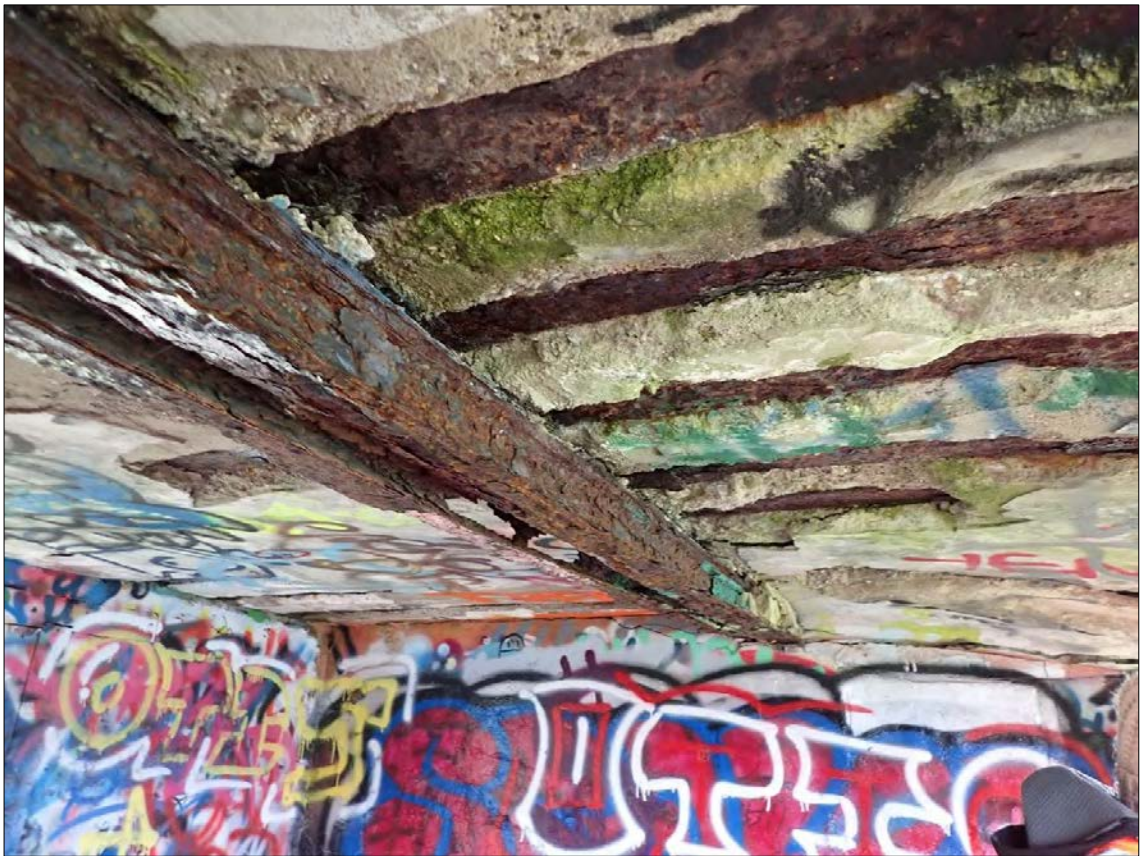
Figure 254. Feature 27: Fort Ballance. Pit B lookout. Underside slab reinforcement corroding and spalling of concrete.
