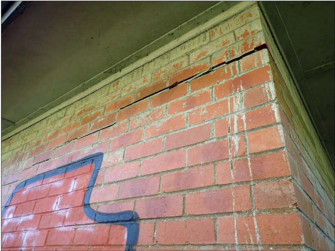
Figure 98. Feature 3: Magazine 3. Typical horizontal crack is evident at the corner of the southern (side) elevation.
