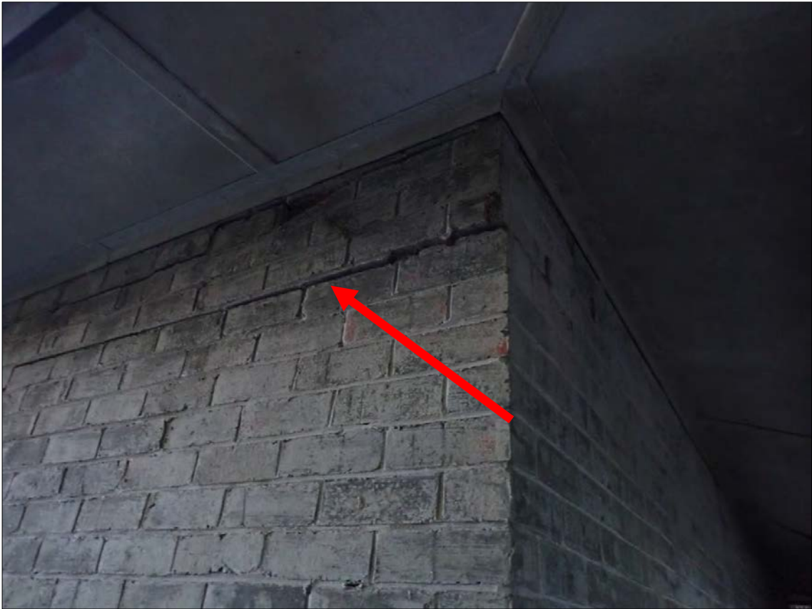
Figure 133. Feature 8: Magazine 8. Looking at the southeastern (rear) corner. A typical horizontal crack is indicated.
