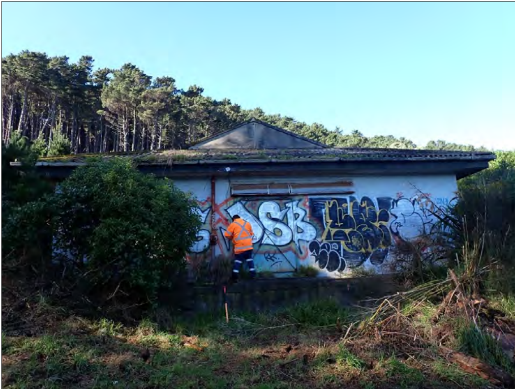
Figure 94. Feature 3: Magazine 3. Looking towards the western (front) elevation. Graffiti is present and there is vegetation in the gutters. The narrow loading deck is overgrown on the outer perimeters.
