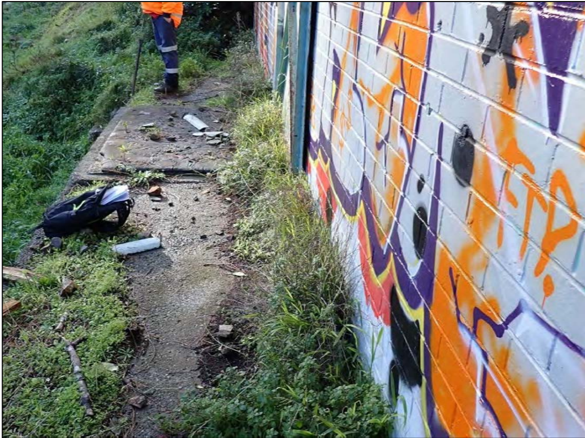
Figure 125. Feature 7: Magazine 7. Looking along the northern (front) elevation – cropped image. Vegetation is starting to ‘colonise’ the cracked loading deck.
